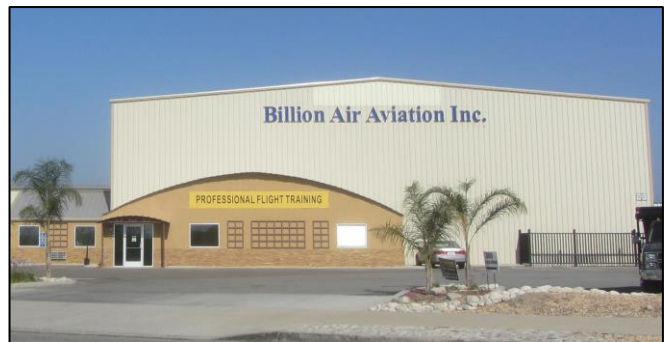
New hangar and flight school constructed along Fairplex Drive on the east side of Brackett Field, 2014.
