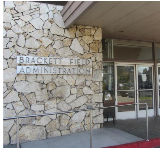
Brackett Field Administration Building, 2014.
