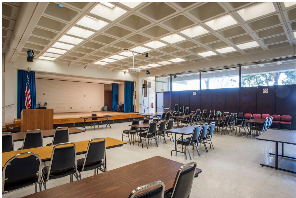
Figure 11 View of Existing Interior Illustrating Coffered Ceiling/Roof
