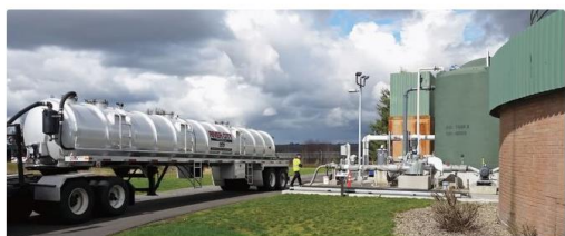
A hauler connects to FOG receiving station at City of Gresham, Oregon Water Resource Recovery Facility. Photo courtesy of City of Gresham WRRF
