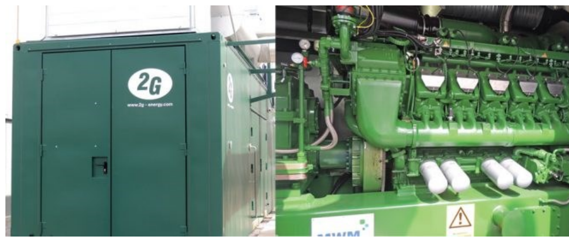
The 1.2 megawatt combined heat and power generator (right) is integrated with related components and housed in a container (left) supplied by 2G Energy.
