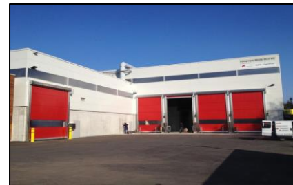
Winterthur (CH) PF1500 steel digester & biogas upgrading
