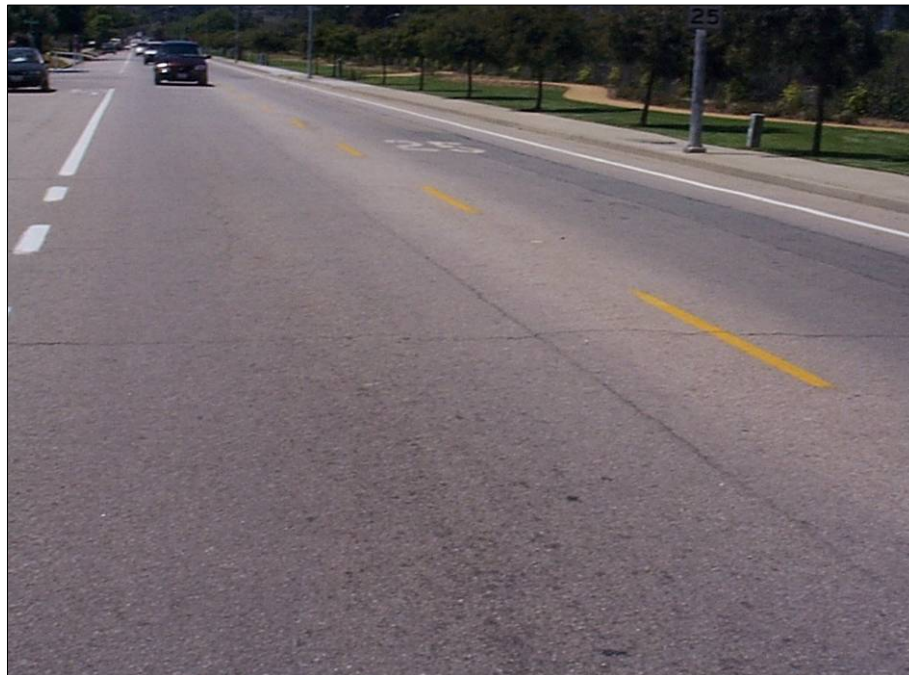
Figure 3.4 PCI = 82 (Good Condition)
