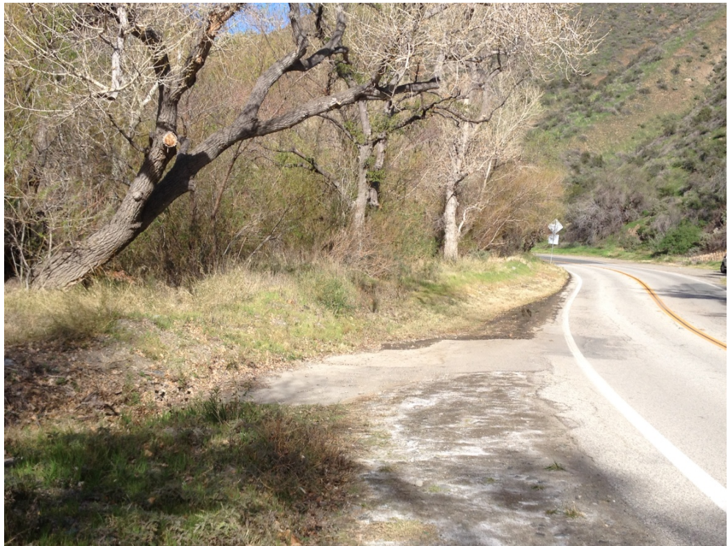
Photograph 6: North-facing view of Site 2, from the downstream end, depicting native trees, existing overshoot, and water seepage onto the road.
