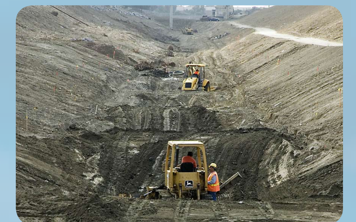
The Dominguez Gap Wetlands project under construction in 2006
