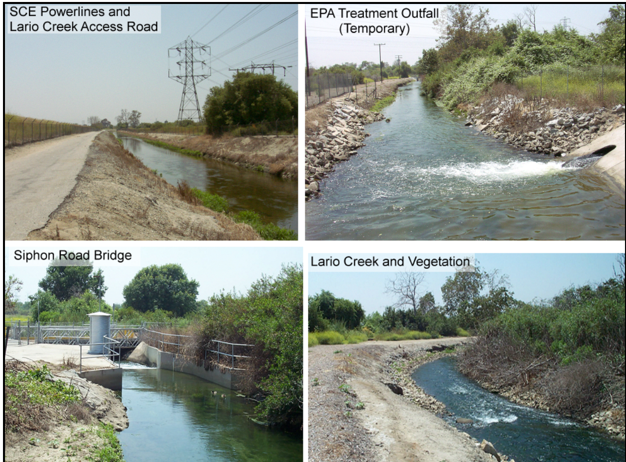
Figure 3-10 Lario Creek Existing Conditions
