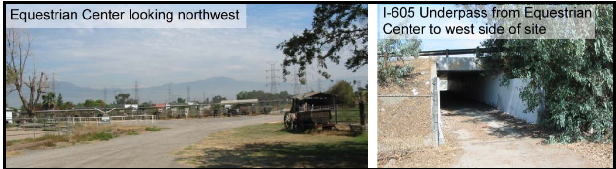
Figure 3-5 Equestrian Facility Existing Conditions
