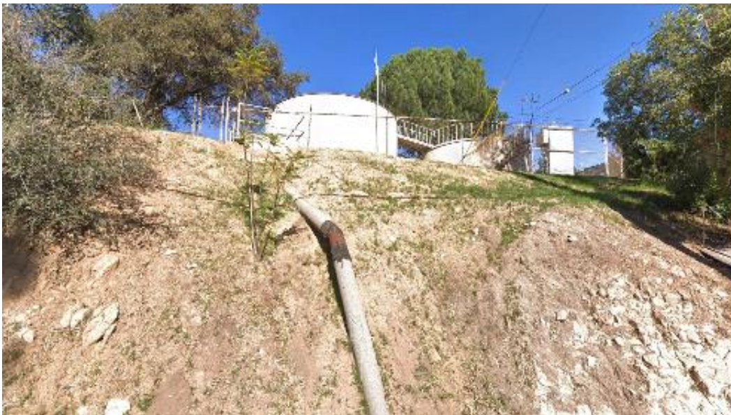
Photo 3.1-2 Fernwood Tanks, Fernwood Pacific Drive View
