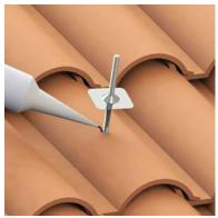
8. Apply fresh compatibale sealant to seal the tile openinig and lower the mini flashing.
