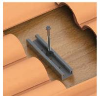
2. & 3. Insert the lag bolt through the tile strut base and apply compatible sealant.
