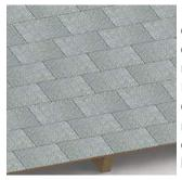
1. Locate, choose, and mark centers of rafters . Select the courses of shingles where mounts will be placed and Drill a pilot hole using 3/16" drill bit through the roof materials and into the center of the rafter at the planned location.
