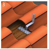
3. Position the roof hooks to the side of the underlying interlocking tile's valley.
