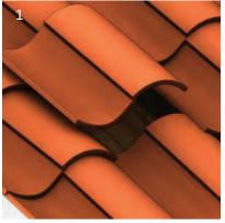
1. Remove the roof tiles at the marked position or, if possible simply push them up. When using 5/16" lag bolt drill a pilot hole 1st. Take care not to warp or damage the roof panel when tightening the nut.
