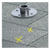
1. Drill two pilot holes using 3/16" drill bit through the roof material and into the center of the rafter at the planned location.
