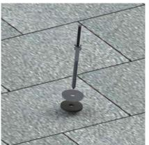
1. Drill a pilot hole using 3/16" drill bit through the roof material and into the center of the rafter at the planned location.
