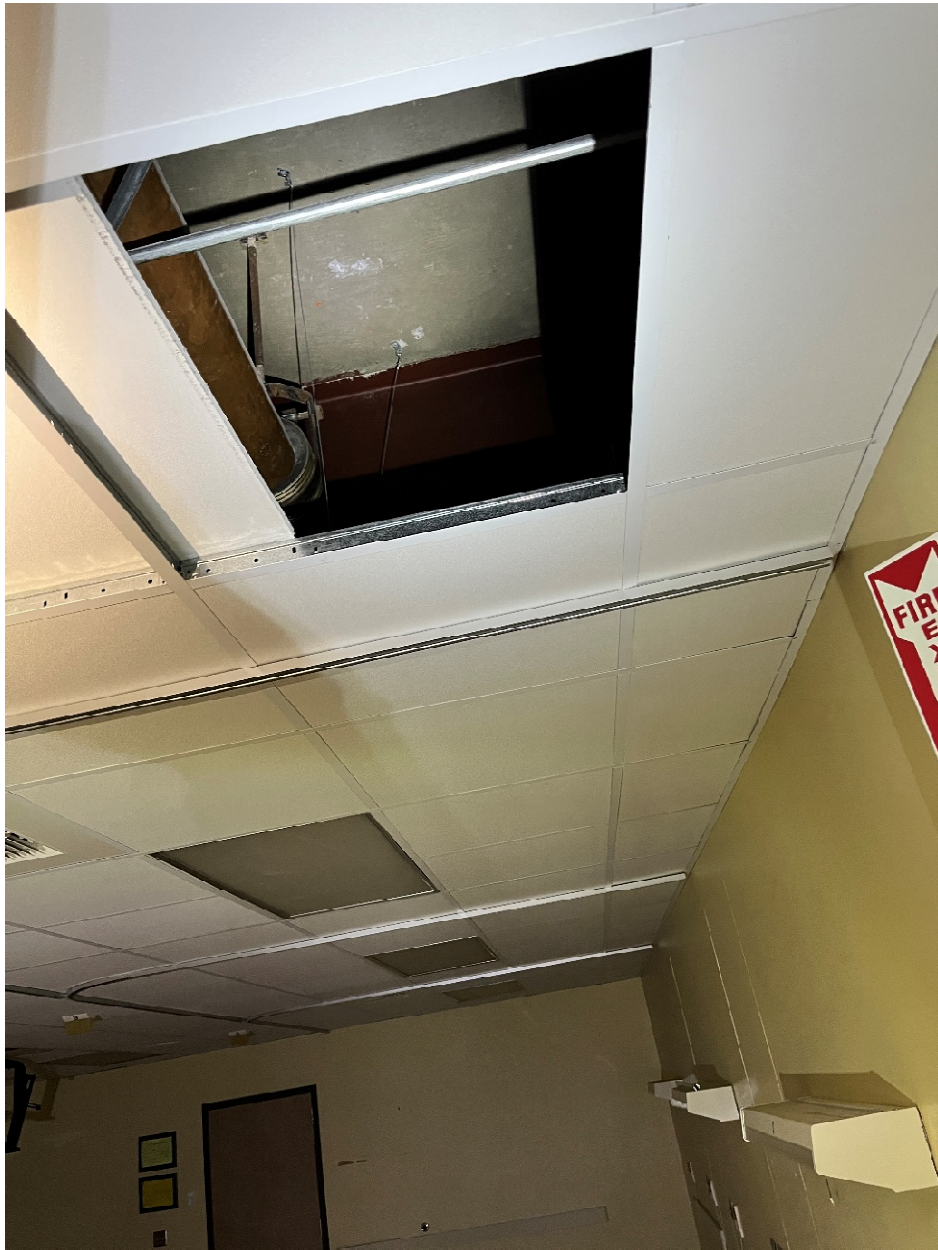
Beam in Ceiling
