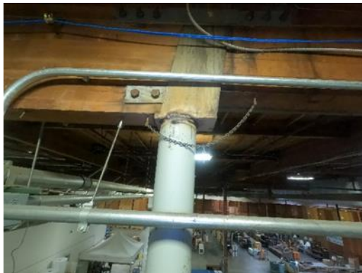
Image 14: Hinge Connector Support
