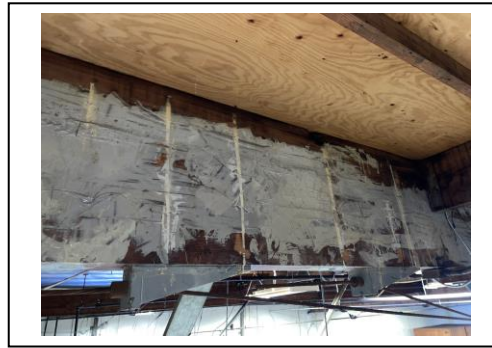
Image 13: Previously Repaired Beam
