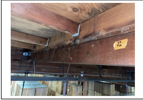
Image 9: Joist Hangers
