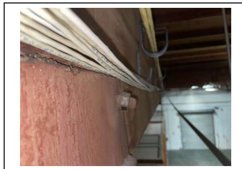
Image 12: Bent Column to Girder Connection Bolt
