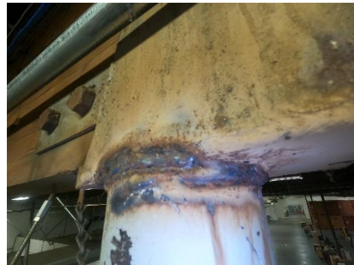
Image 15: Column to Hinge Connector Weld
