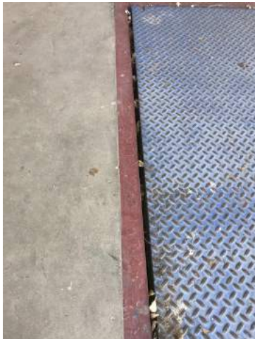
View of Red Metal Hydraulic Lift
