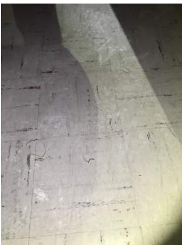
View of 9" x 9" Pink with Black and Red Streaked Resilient Flooring/Resilient Floor Mastic
