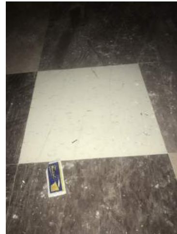
View of 12" x 12" White with Light Brown Streaked Resilient Flooring/Resilient Floor Mastic
