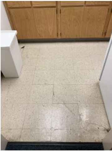
View of 12" x 12" Tan with Brown and White Streaked Resilient Floor Tile/Resilient Floor Mastic
