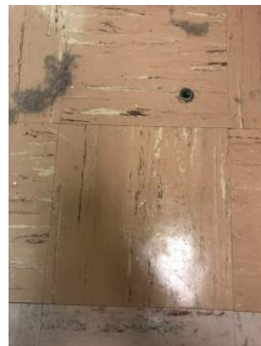
View of 9" x 9" Light Brown with Tan and Dark Brown Streaked Resilient Flooring/Resilient Floor Mastic
