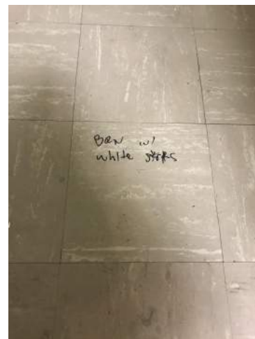
View of 9" x 9" Brown with White Streaked Resilient Flooring/Resilient Floor Mastic
