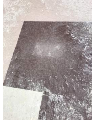
View of 12" x 12" Dark Brown Streaked Resilient Flooring/Resilient Floor Mastic
