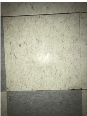
View of 12" x 12" White with Blue and Red Streaked Resilient Flooring/Resilient Floor Mastic
