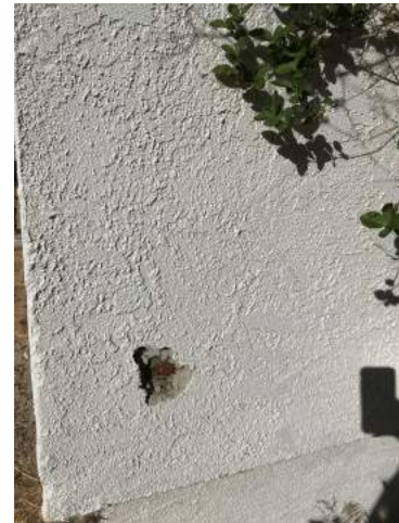
View of Exterior Stucco with Vapor Barrier
