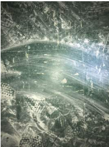
View of 9" x 9" Green with White Streaked Resilient Flooring/Resilient Floor Mastic
