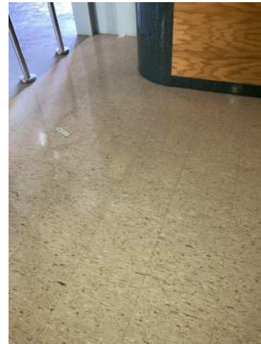
View of 12" x 12" Brown with Red Stripes Resilient Floor Tile/Resilient Floor Mastic
