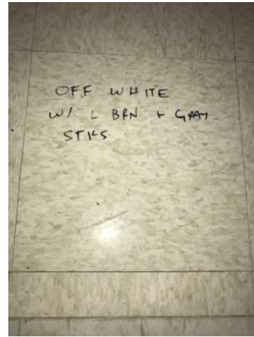
View of 12" x 12" Off-White with Light Brown and Gray Streaked Resilient Flooring/Resilient Floor Mastic
