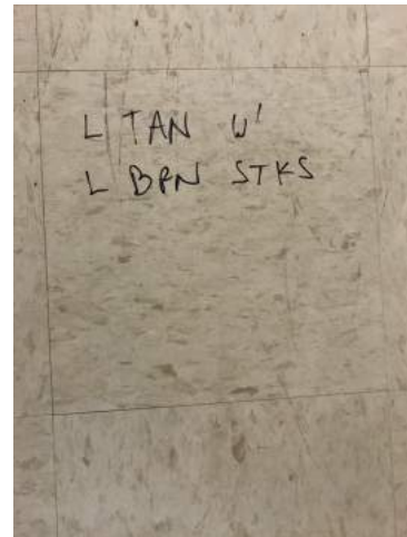
View of 12" x 12" Light Tan with Light Brown Streaked Resilient Flooring/Resilient Floor Mastic
