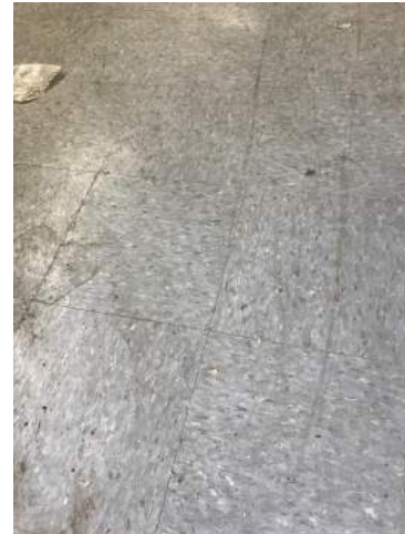
View of 12" x 12" Light Blue Streaked Resilient Flooring/Resilient Floor Mastic
