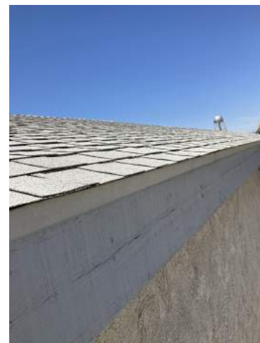
View of Shingle Roof
