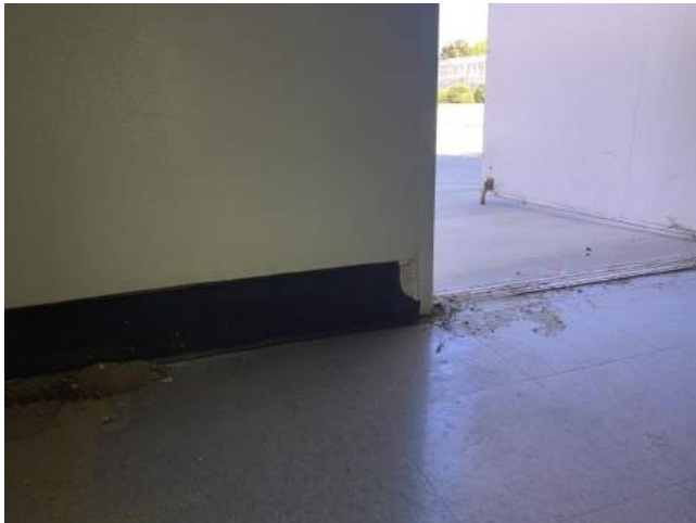
View of 6" Black Cove Base/Cove Base Mastic
