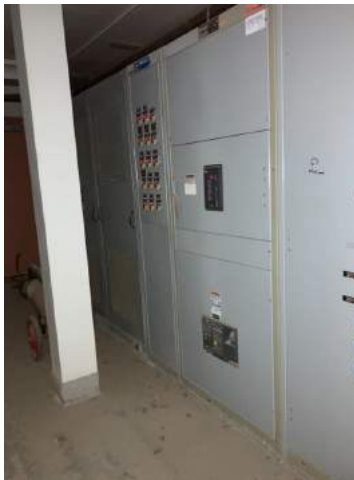
View of Transformers
