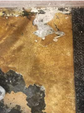
View of Carpet Glue with Leveling Compound
