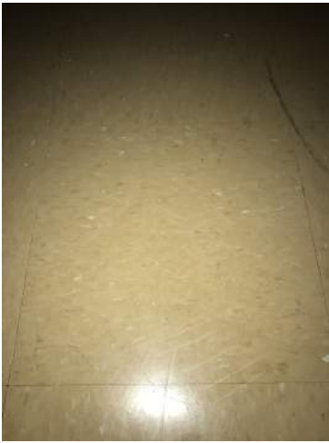
View of 12" x 12" Orange with White Streaked Resilient Flooring/Resilient Floor Mastic
