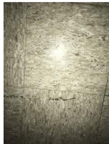
View of 12" x 12" Brown and White Streaked Resilient Flooring/Resilient Floor Mastic
