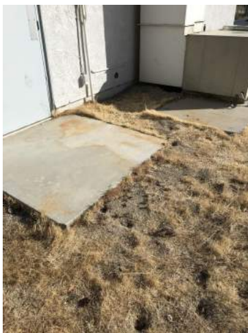
View of Concrete
