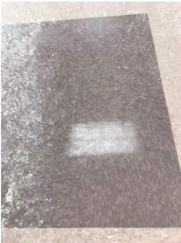
View of 12" x 12" Light Brown Streaked Resilient Flooring/Resilient Floor Mastic
