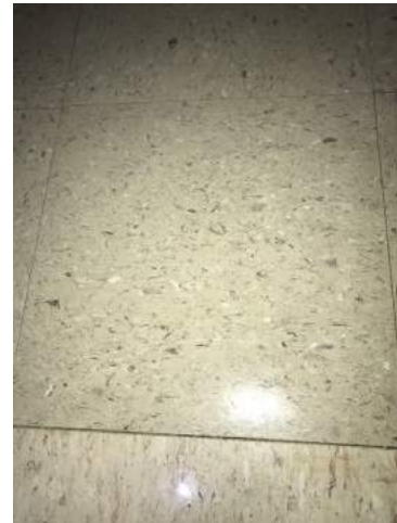
View of 12" x 12" Tan With Brown and White Streaked Resilient Flooring/Resilient Floor Mastic
