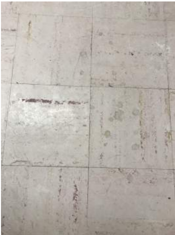
View of 9" x 9" Pink with Red and Brown Streaked Resilient Flooring/Resilient Floor Mastic
