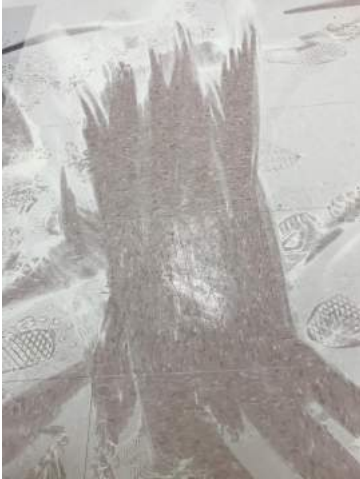
View of 12" x 12" Pink Streaked Resilient Flooring/Resilient Floor Mastic
