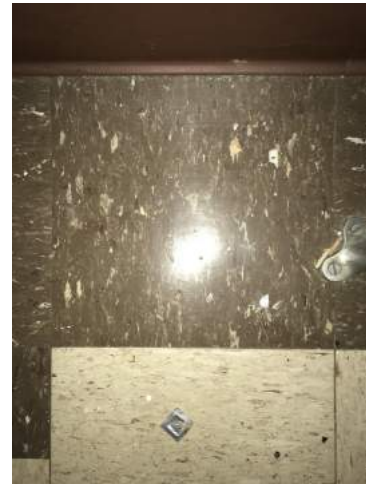
View of 12" x 12" Dark Brown with Tan Streaked Resilient Flooring/Resilient Floor Mastic
