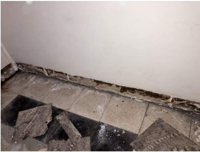
View of 12" x 12" Brown with Brown Streaked Resilient Floor Tile/Resilient Floor Mastic
