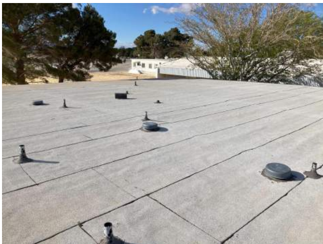
View of Rolled Roof
