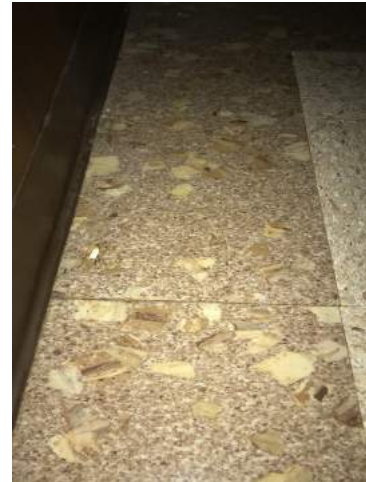
View of 12" x 12" Brown with Gold Flakes Resilient Flooring/Resilient Floor Mastic
