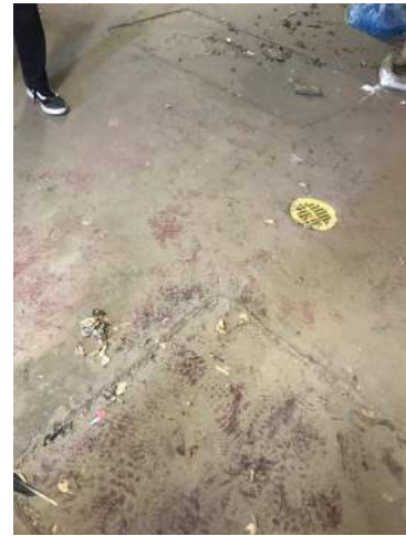
View of Concrete
