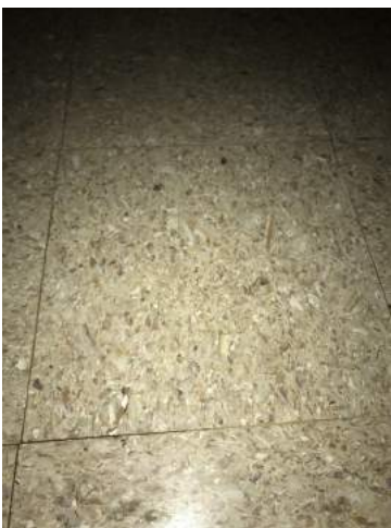
View of 12" x 12" Granite Pattern Resilient Flooring/Resilient FloorMastic
