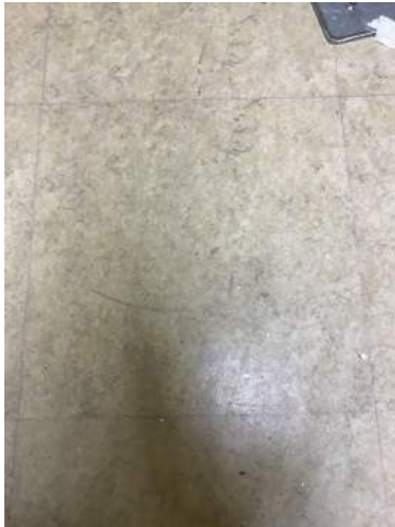
View of 24" x 24" Gold Resilient Flooring/Resilient Floor Mastic
