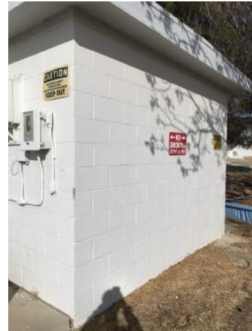
View of Brick and Mortar
