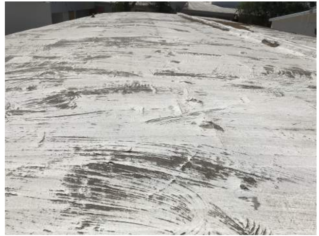
View of Woven Roof Material with Sealant
