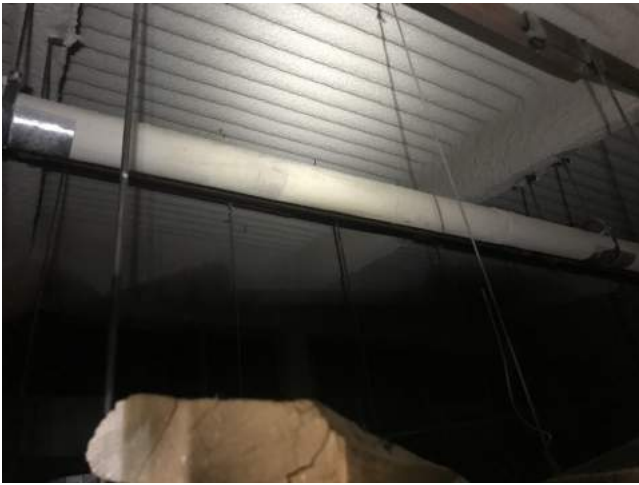
View of Wheat Tape with Yellow Insulation Pipe Wrap
