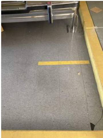
View of 12" x 12" Blue with Gray Stripes Resilient Flooring/Resilient Floor Mastic
