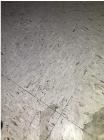
View of 12" x 12" Light Brown with Red Streaked Resilient Flooring/Resilient Floor Mastic
