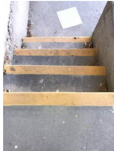
View of Yellow Concrete Stair
