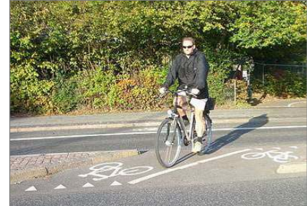
Medians on bicycle boulevards should provide space for a bicyclist to wait.
