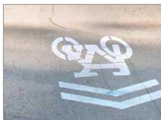
Shared lane markings also provide directional support for bicyclists.
