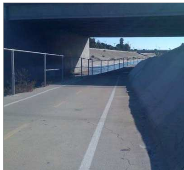
Undercrossings provide key connections and allow path users to avoid a potentially dangerous at-grade crossing of a major street.
