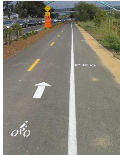
Centerline striping and directional arrows encourage trail users to provide space for other users to pass.
