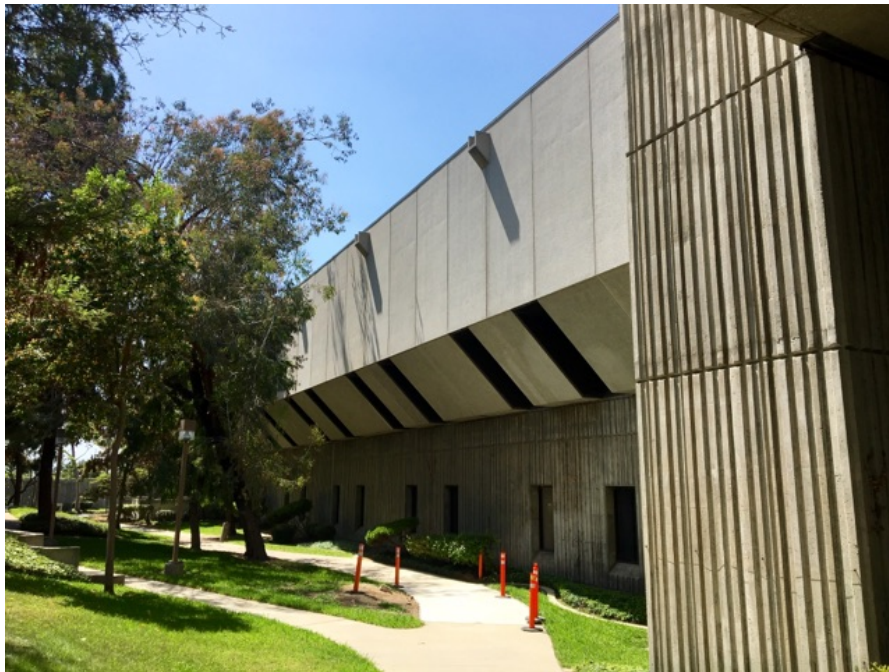
Figure 8 View of Hawkins Building and Walled Courtyard looking West
