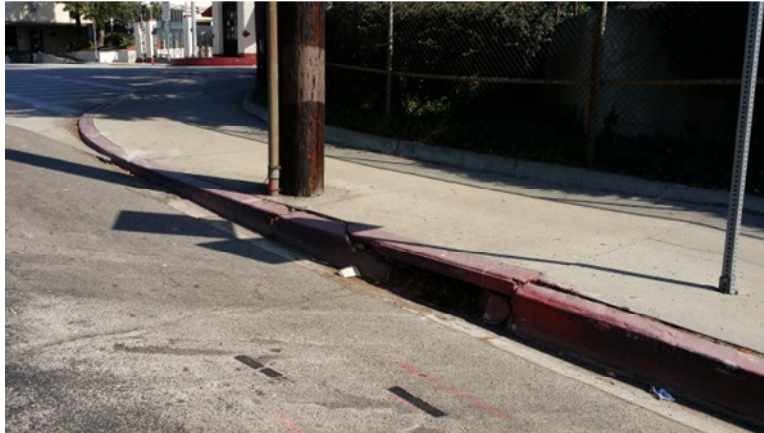
Photo 13: Storm Drain Inlet Along Zonal Avenue
