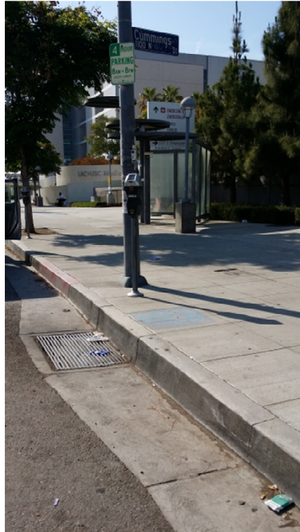
Photo 28: Storm Drain Inlet Along Marengo Street
