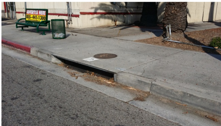
Photo 44: Storm Drain Inlet Along Mission Road
