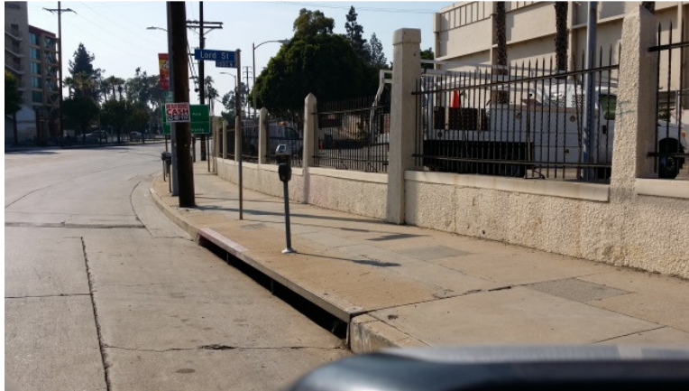
Photo 42: Storm Drain Inlet Along Marengo Street at Lord Street Intersection
