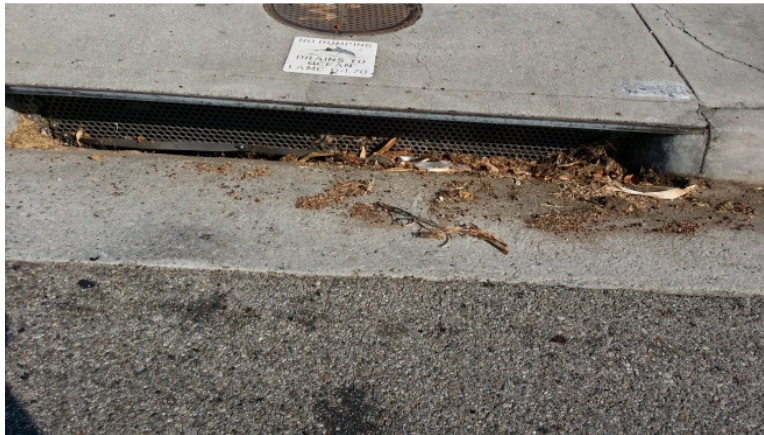
Photo 45: Storm Drain Inlet with Screens Along Mission Road
