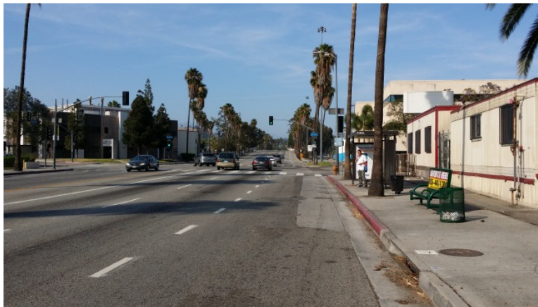
Photo 43: Storm Drain Inlet Along Mission Road
