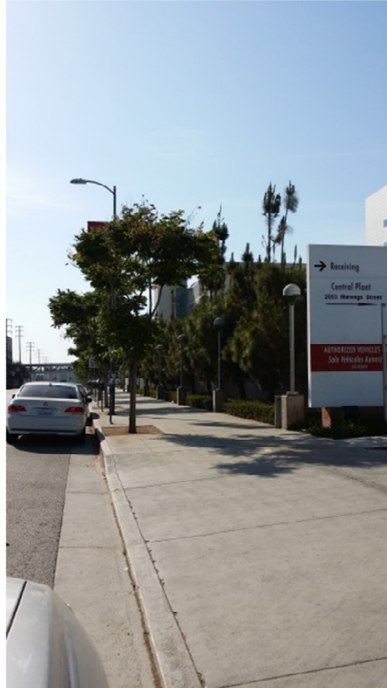
Photo 26: Storm Drain Inlet Along Marengo Street
