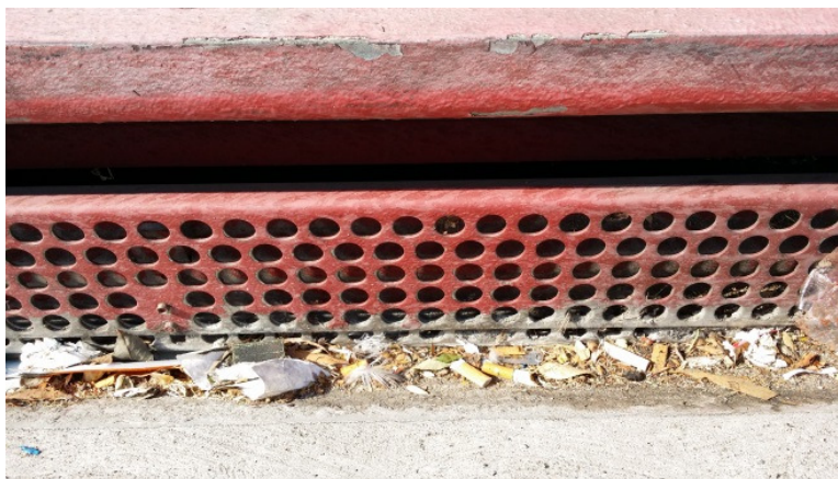
Photo 41: Storm Drain Inlet with Screens Along Marengo Street
