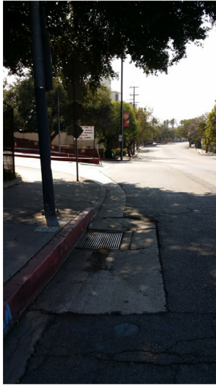
Photo 9: Storm Drain Inlet Along Zonal Avenue
