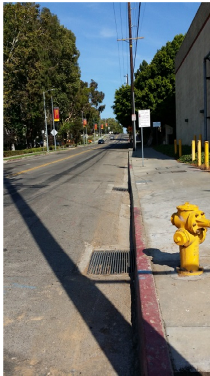
Photo 14: Storm Drain Inlet Along Zonal Avenue
