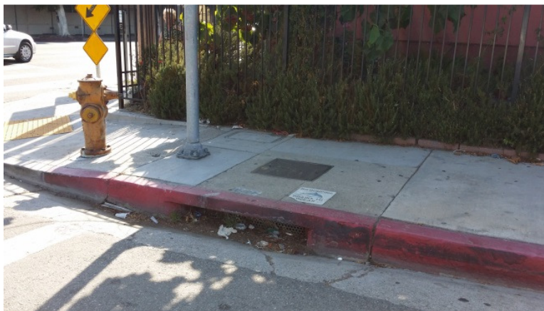
Photo 22: Storm Drain Inlet Along Cornwell Street at Marengo Street Intersection
