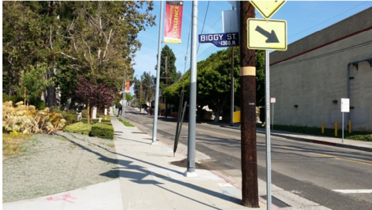
Photo 17: Storm Drain Inlet Along Zonal Avenue at Biggy Street Intersection
