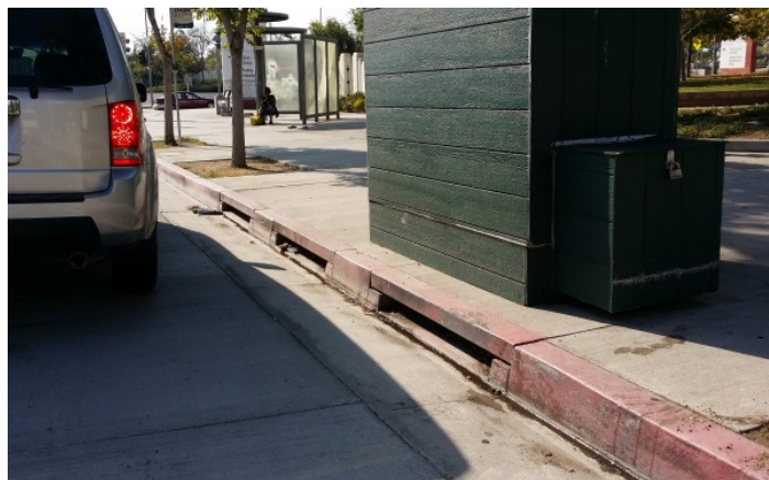
Photo 35: Storm Drain Inlet Along Marengo Street
