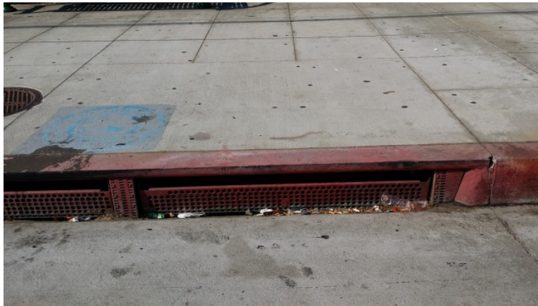
Photo 40: Storm Drain Inlet with Screens Along Marengo Street
