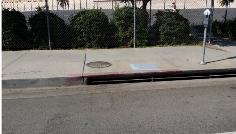
Photo 7: Storm Drain Inlet Along Zonal Avenue
