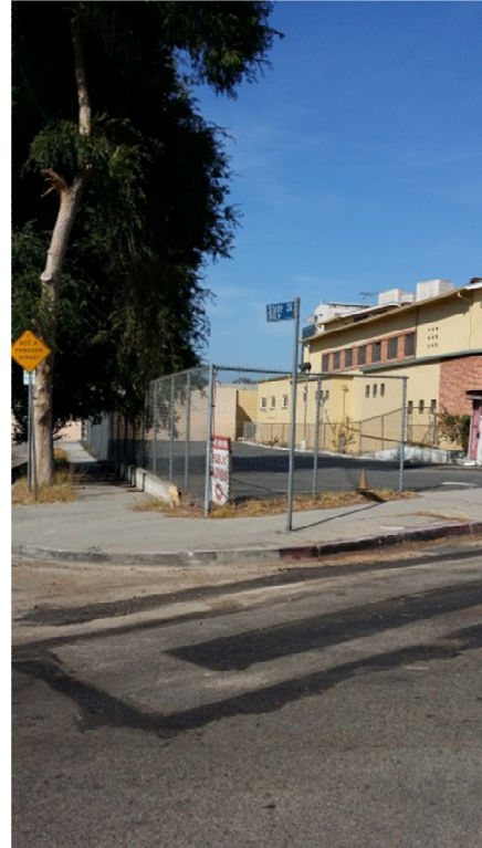
Photo 12: Storm Drain Inlet Along Zonal Avenue
