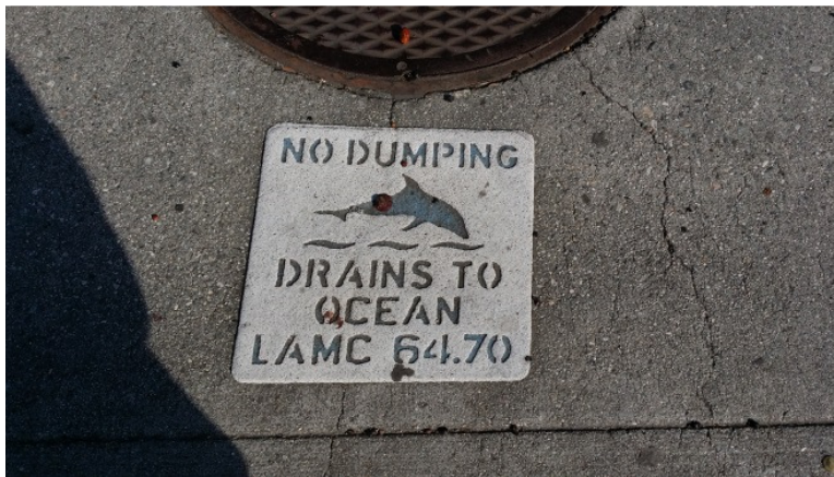
Photo 46: No Dumping Stencil at Storm Drain Inlet Along Mission Road
