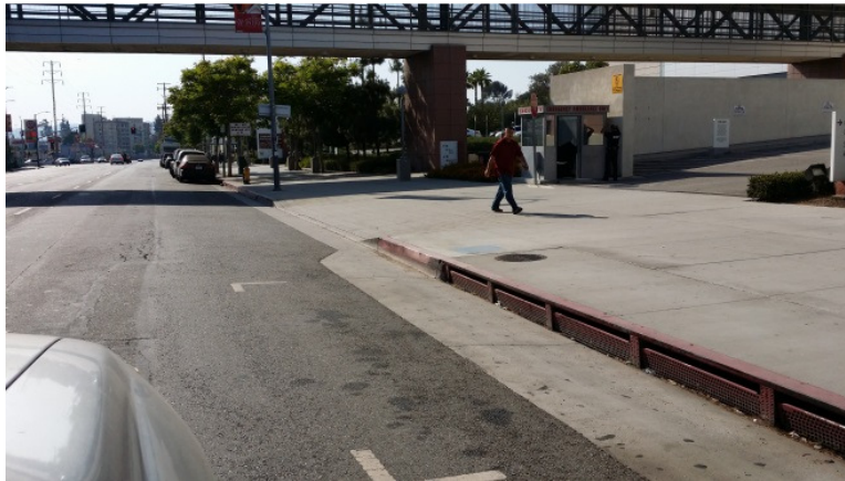
Photo 33: Storm Drain Inlet with Screens Along Marengo Street
