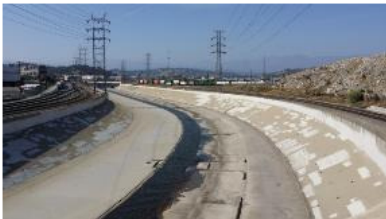
Photo 3: Los Angeles River Looking North from East Cesar Chavez Avenue Crossing Near Mission Road
