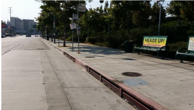
Photo 39: Storm Drain Inlet with Screens Along Marengo Street
