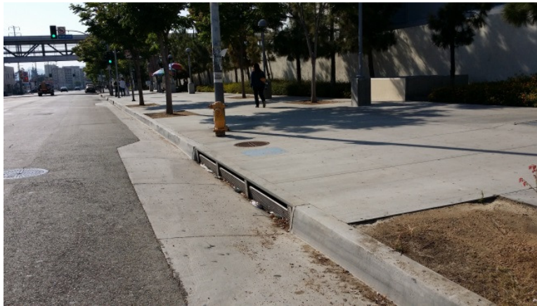
Photo 29: Storm Drain Inlet with Screens Along Marengo Street
