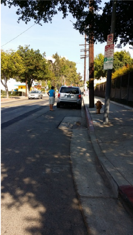
Photo 11: Storm Drain Inlet Along Zonal Avenue
