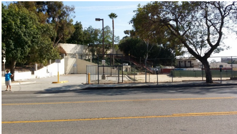
Photo 8: Storm Drain Inlet Along Zonal Avenue
