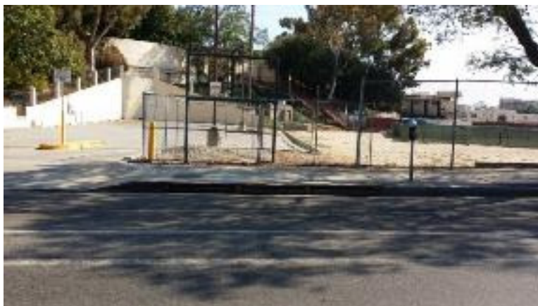
Photo 6: Storm Drain Inlet Along Zonal Avenue
