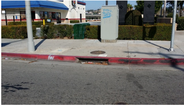
Photo 23: Storm Drain Inlet Along Marengo Street
