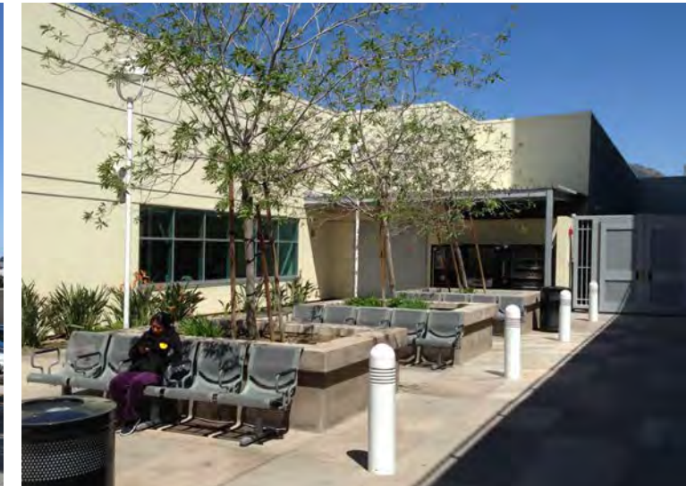
3.20 Photo of Emergency Services Building Courtyard
