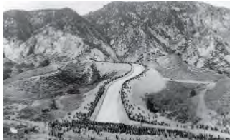
1.03 Historical photo of Los Angeles Aqueduct
