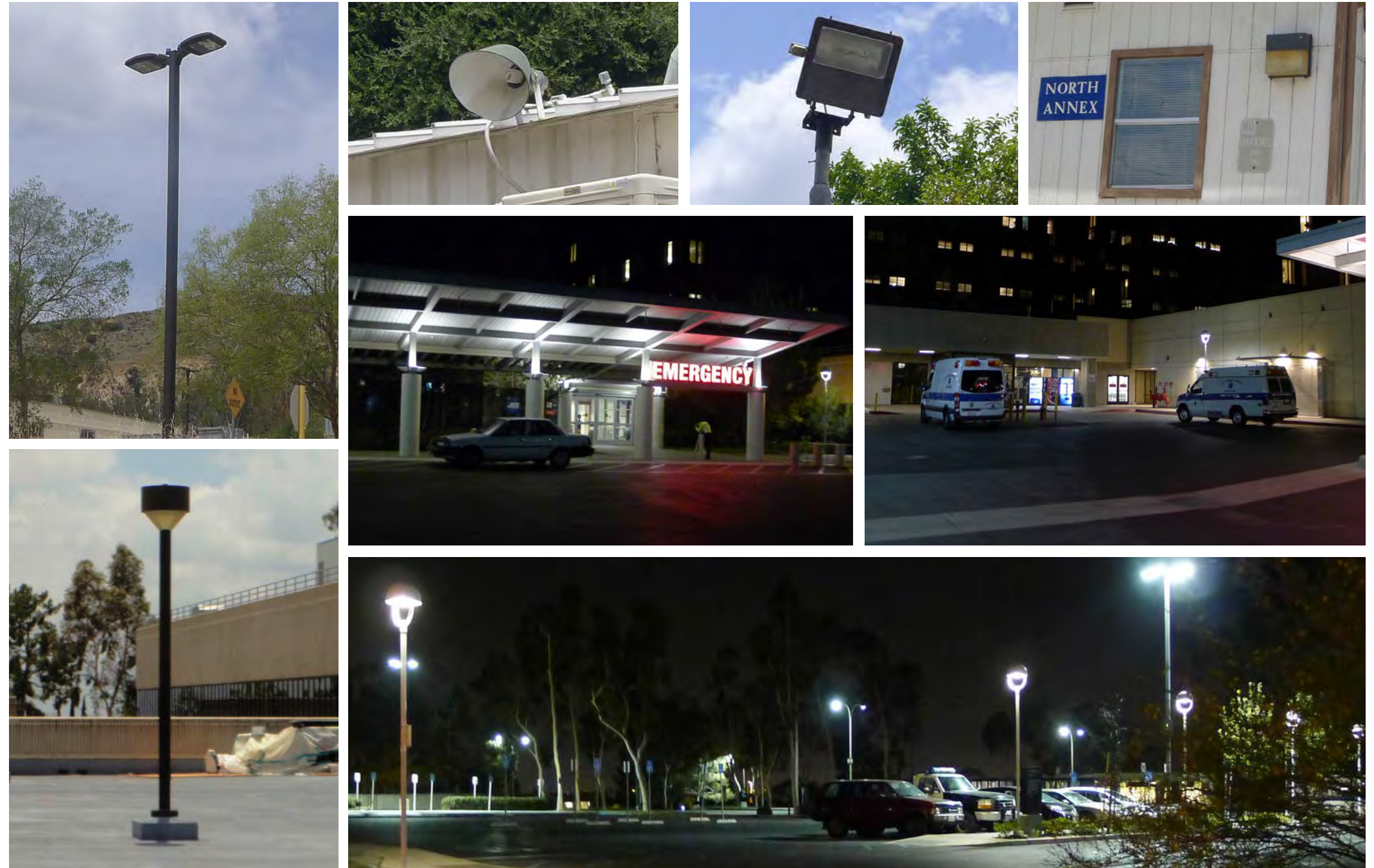
3.35 Photos of Existing Site Lighting
