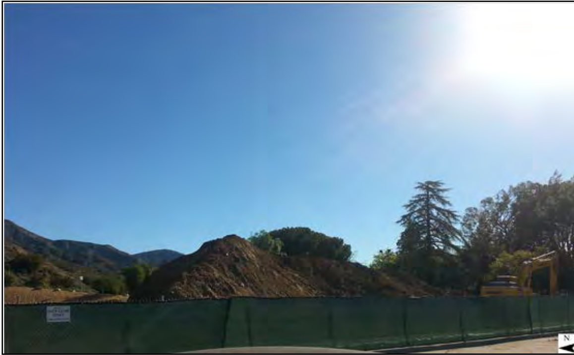
Figure 11. Construction Zone and Fenced Area at Northeast Corner of Survey Area
