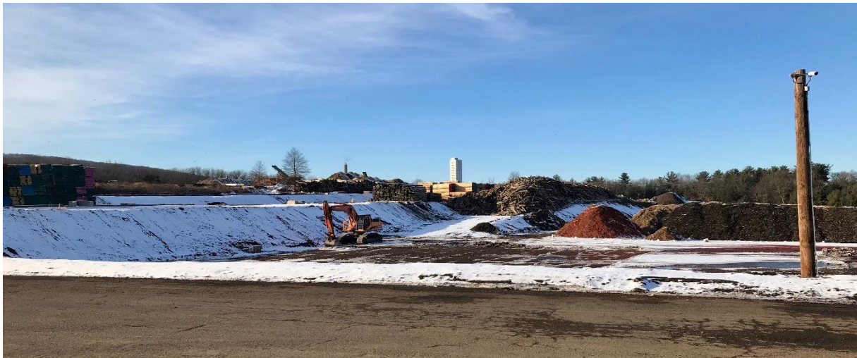
Site of future depackaging facility Credit: Cole Rosengren
