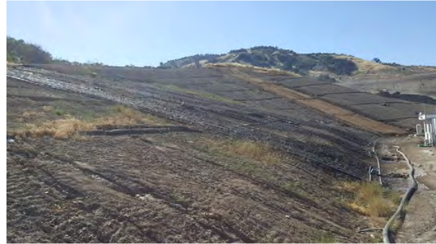
Photo 9 – Topsoil placement on section 4 complete
