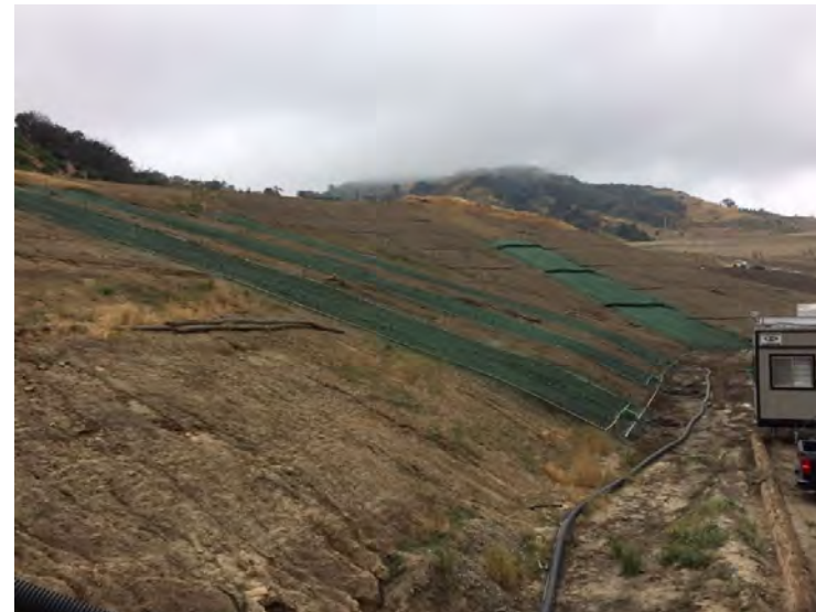
Photo 11 – Hydroseed placement complete
