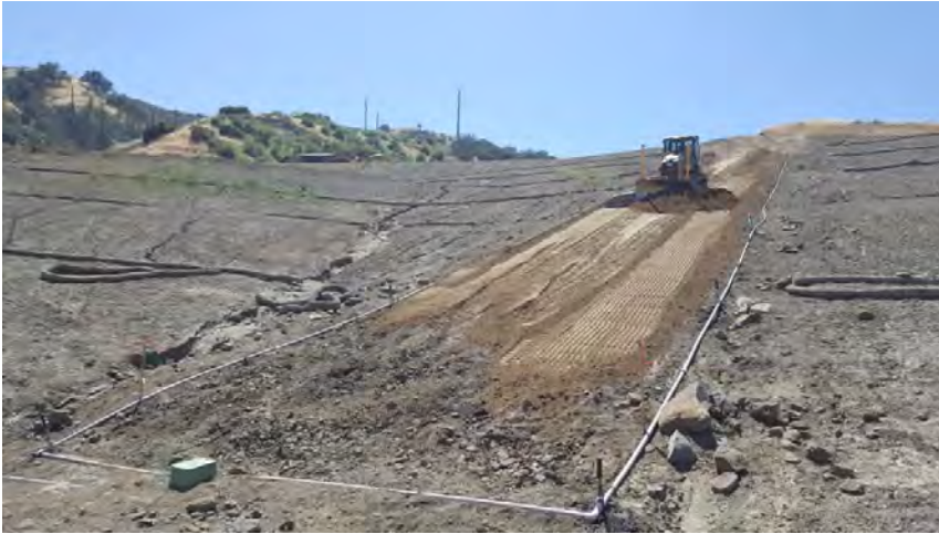
Photo 8 – Topsoil placement on section 4
