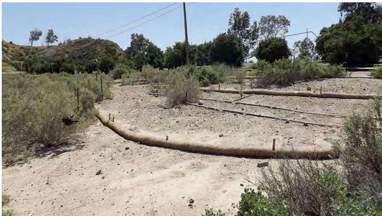
Newly installed straw wattles within the areas that are more exposed
