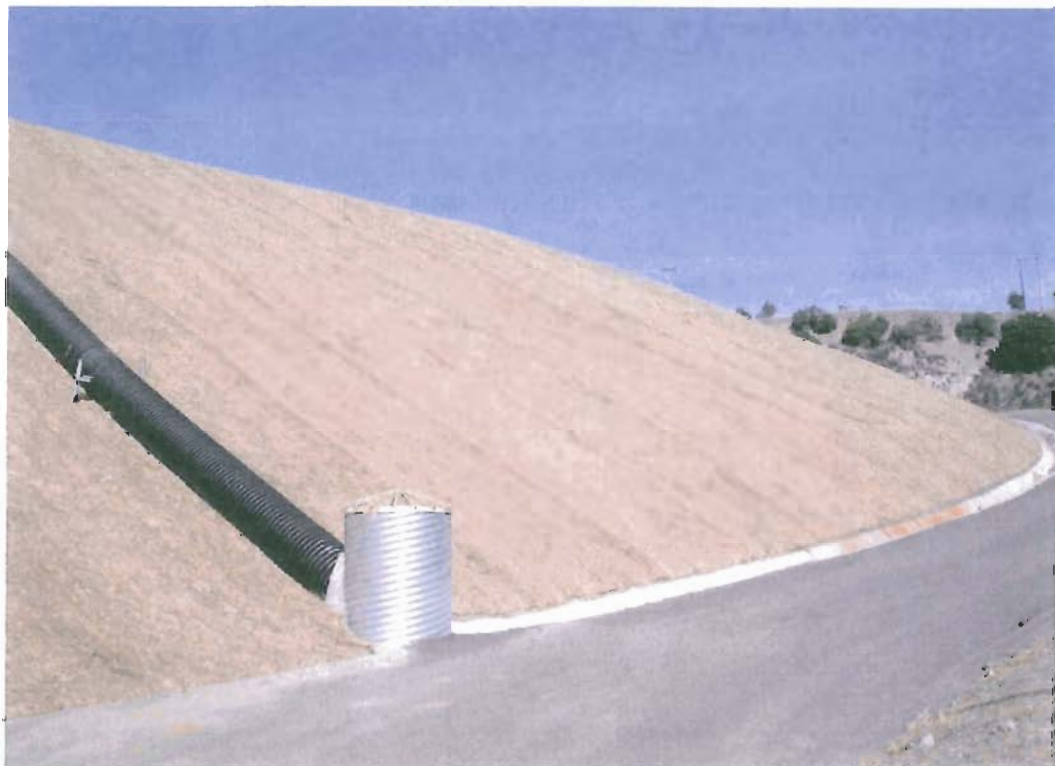
Figure 3. Straw Coconut Matting Installation
