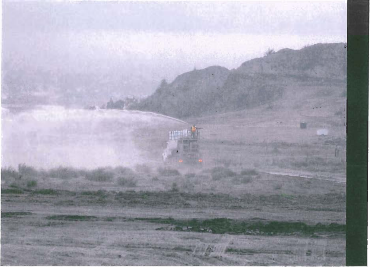
Figure 8. Application of final compost layer.
