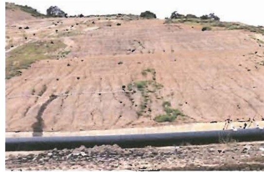
Vegetation coverage in the soils characterized as "poor" is still poor. (Note leaky irrigation head.)
