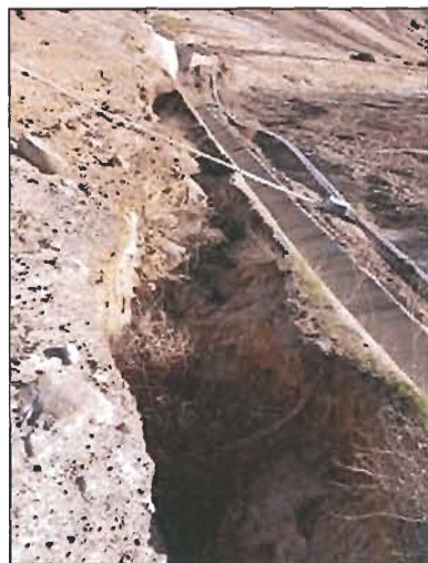
Continuing erosion was observed adjacent to the concrete V-ditches.
