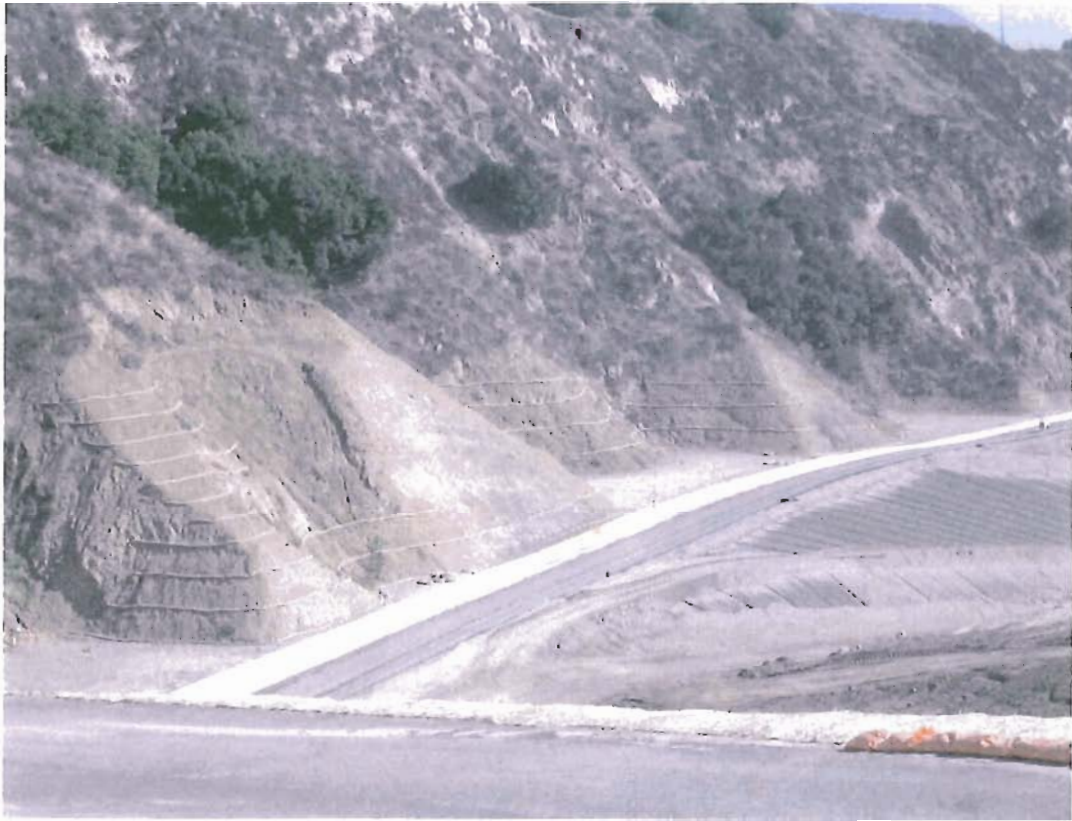
Figure 4. Installation of Straw Wattle on East Slope
