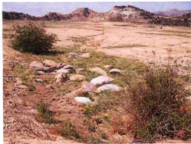
Flowering poppies in a drainage on the top deck. This low spot feeds a drain pipe that carries water off the top deck.
