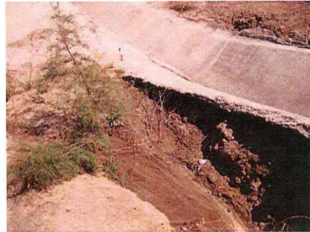
A fennel ( Foeniculum vulgare ) is growing on the erosion ridge caused by the leaking sprinklers or pipes
