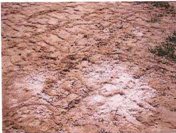
Salt deposits observed on the top deck.
