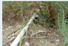
TEMPORARY (2-3 YEARS) ON-GRADE DRIP/BUBBLER SYSTEM "POINT TO POINT" DELIVERY FOR SPECIFIC TREE & SHRUB PLANTINGS
