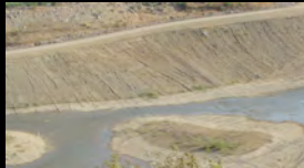
Phase 1 - construction grading of slopes, construction of wetland islands, drop structures and boulder lined channels
