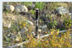
TEMPORARY (2-3 YEARS) ON-GRADE IRRIGATION SYSTEM "OVERHEAD ROTOR SPRAY" (FOR LARGER HYDROSEEDED AREAS)
