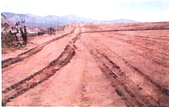
Poles were installed around part of the perimeter of the top deck. The installation of poles had disturbed some of the topsoil.
