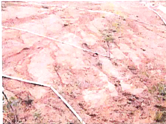
Erosion rills developed after the heavy rain in December 2009.
