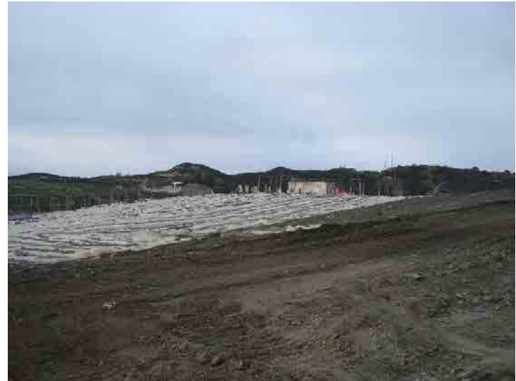
Photo 614: Site Working Area 830-930 am: January 27, 2016
