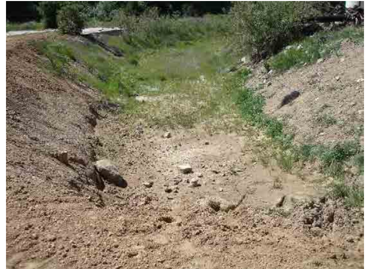
Photo 128: Hillside Drainage into Basin D: March 23, 2016
