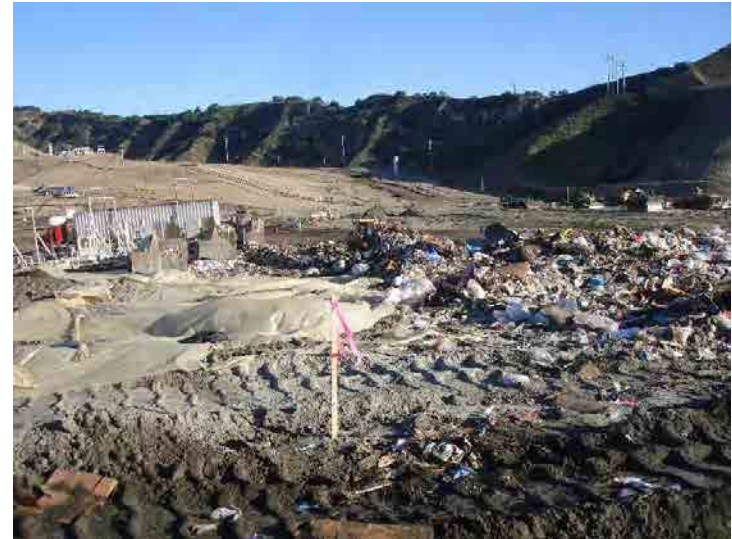
Photo 666: Site Working Area 800am: March 23, 2016
