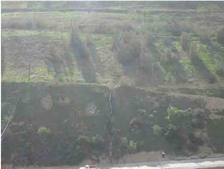
Photo 317: Main Access Road: January 27, 2016
