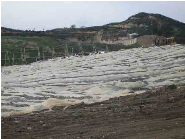
Photo 611: Site Working Area 830-930 am: January 27, 2016
