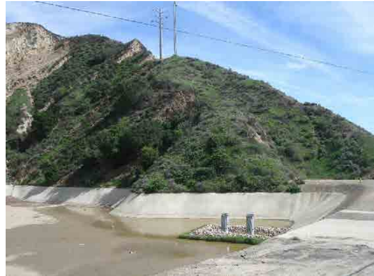
Photo 198: Basin B: March 9, 2016
