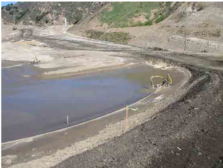
Photo 367: Ponding on City Top Deck: March 9, 2016
