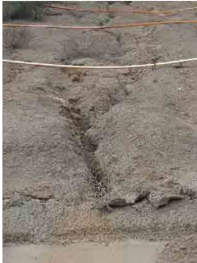
Photo 105: Westside Drainage Channel: January 27, 2016
