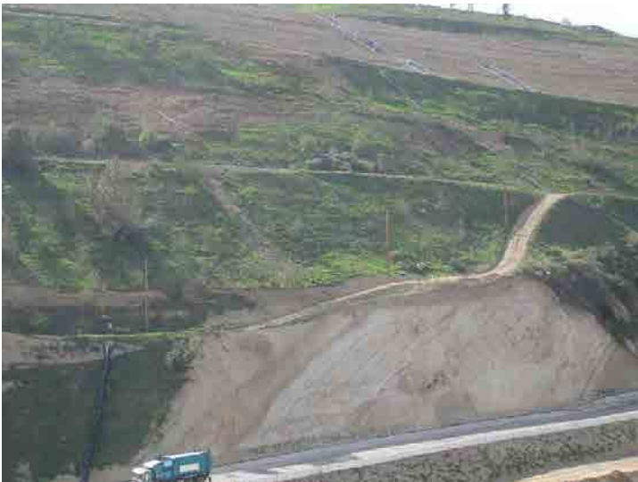
Photo 319: Main Access Road: January 27, 2016
