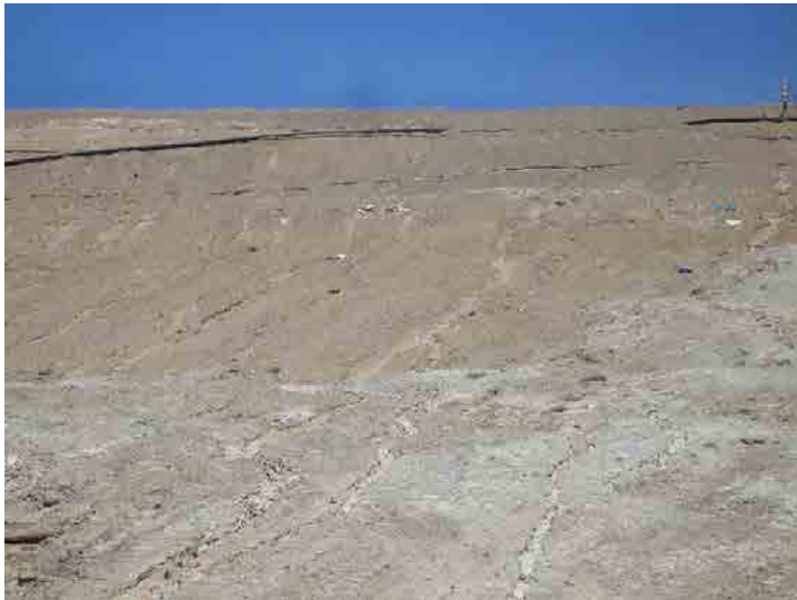
Photo 355: City Slope Erosion, Inert Waste Exposed: February 24, 2016
