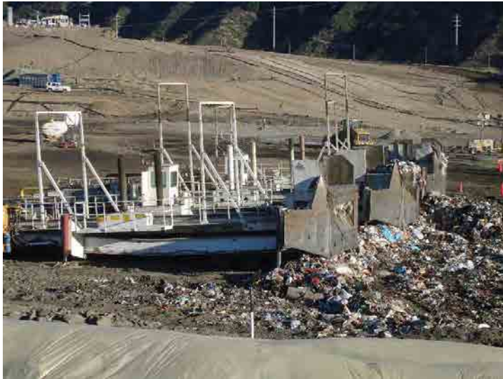
Photo 669: Site Working Area 800am: March 23, 2016
