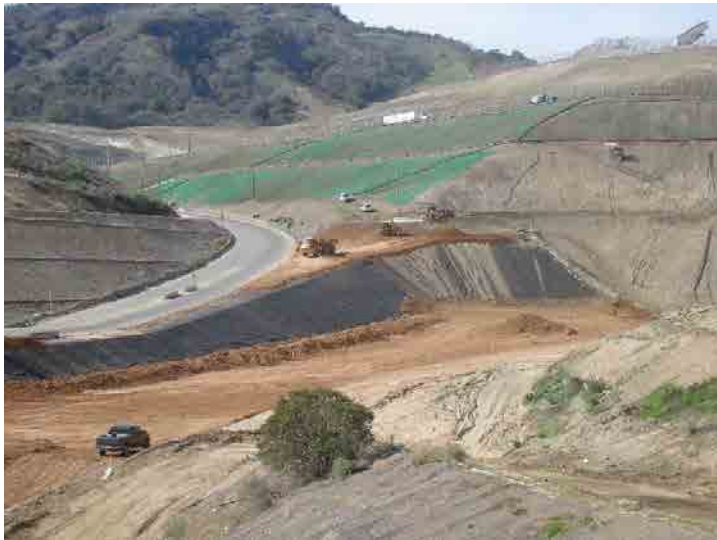
Photo 271: City Cell CC3B Construction: January 27, 2016
