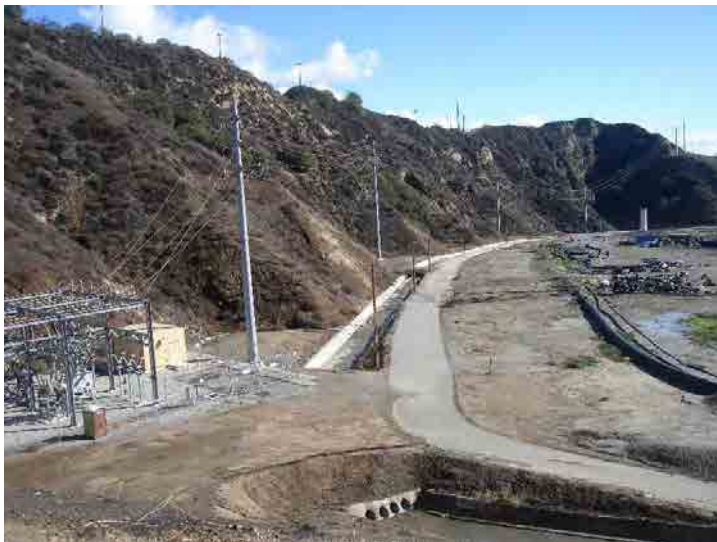
Photo 159: County Top Deck: January 7, 2016
