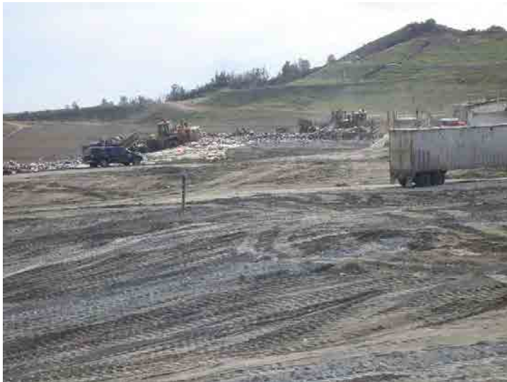
Photo 635: Site Working Area 200 pm: January 27, 2016
