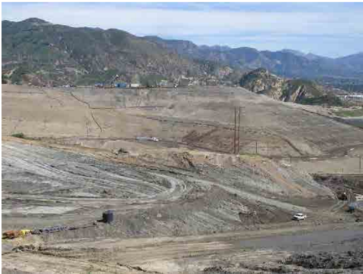
Photo 63: Site Grading South of Basin A: March 9, 2016
