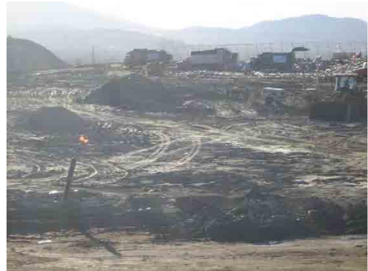
Photo 660: Site Working Area 800am: March 23, 2016
