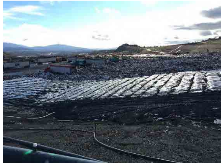
Photo 588: Site Working Area 1000 AM: January 7, 2016
