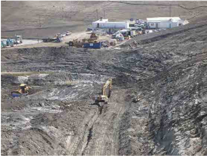
Photo 61: Site Grading South of Basin A: February 24, 2016
