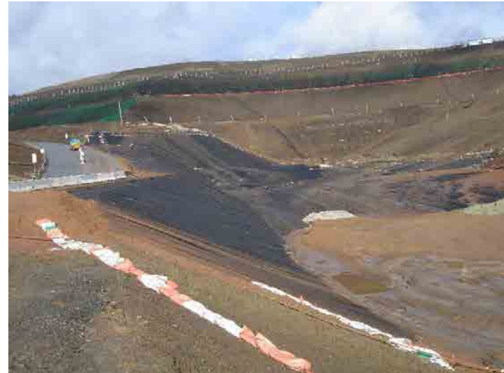
Photo 258: City Cell CC3B Construction: January 7, 2016
