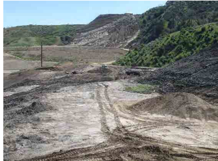
Photo 66: Site Grading South of Basin A March 9, 2016
