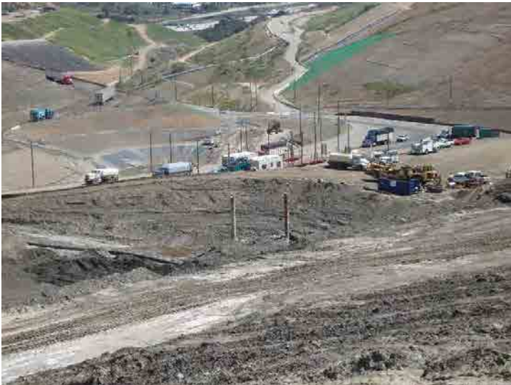
Photo 75: Oil Well Casings to be Abandoned: March 23, 2016
