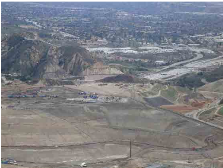
Photo 627: Site Working Area 12 noon: January 27, 2016
