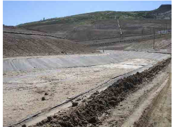
Photo 86: City Lined Drainage Lift Area: February 24, 2016
