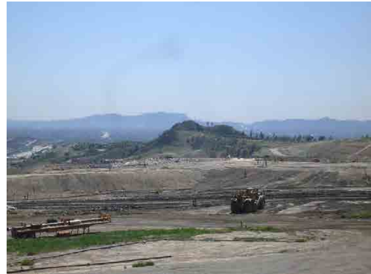
Photo 676: Site Working Area 100 pm: March 23, 2016
