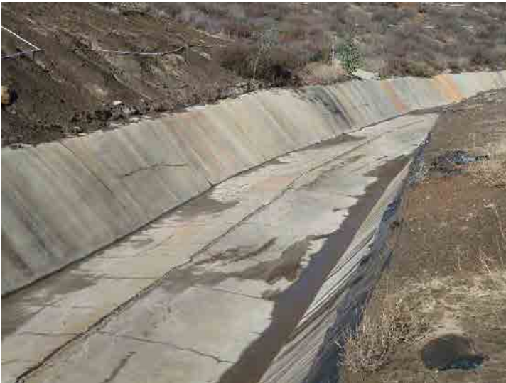
Photo 95: Westside Drainage Channel: January 7, 2016
