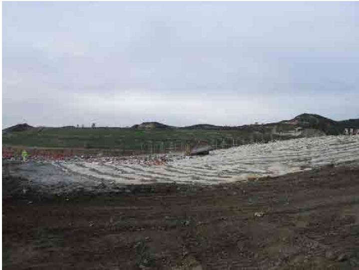
Photo 613: Site Working Area 830-930 am: January 27, 2016
