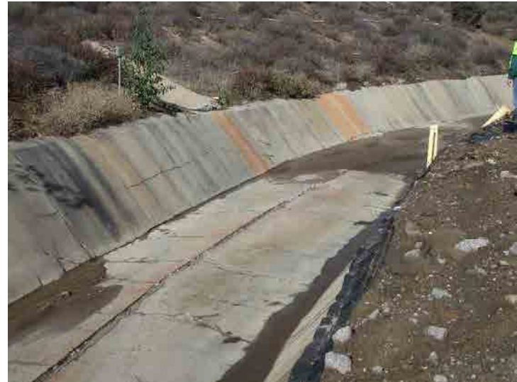
Photo 96: Westside Drainage Channel: January 7, 2016
