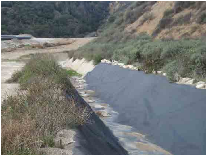
Photo 137: Basin D Outlet Channel: January 27, 2016
