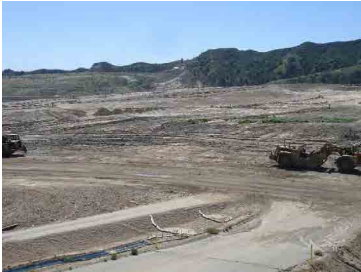
Photo 177: Site County Top Deck: March 23, 2016
