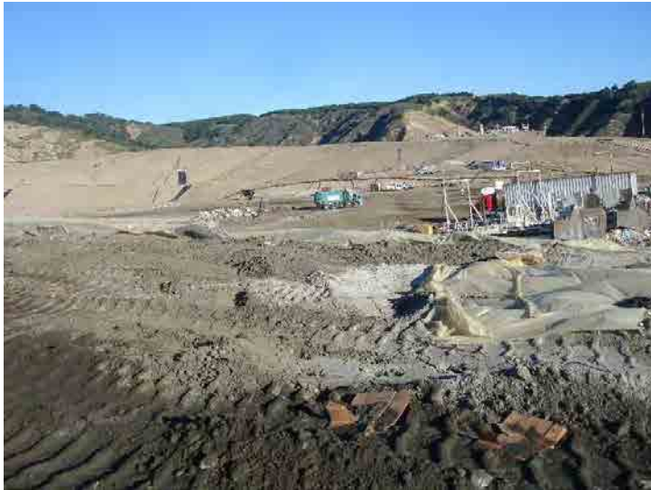
Photo 665: Site Working Area 800am: March 23, 2016
