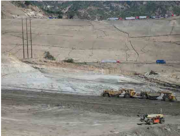
Photo 677: Site Working Area 100 pm: March 23, 2016
