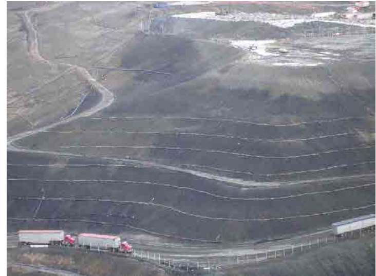
Photo 598: Site Working Area 2:00 pm: January 7, 2016
