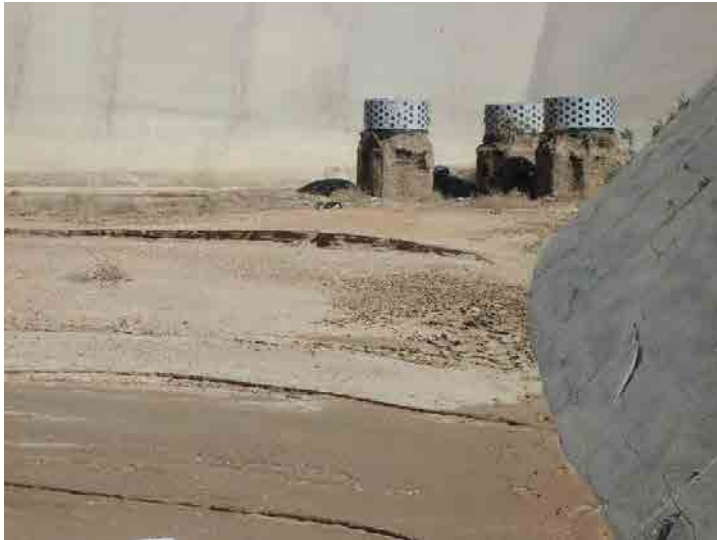
Photo 245: Terminal Basin: February 24, 2016
