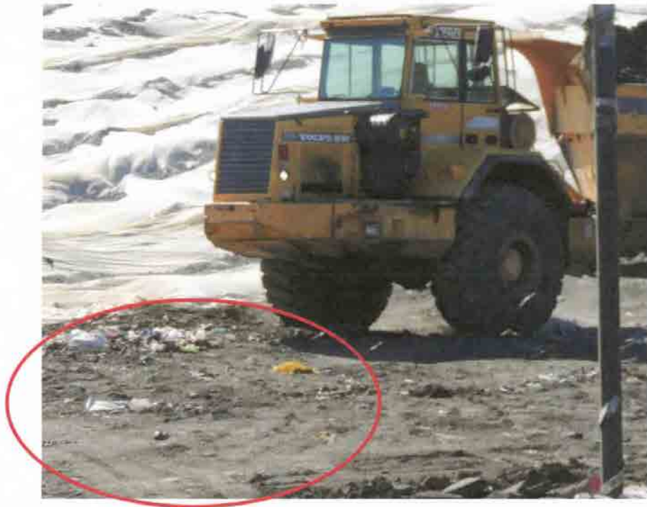
Photo 11: Waste not covered by ADC along the edges
