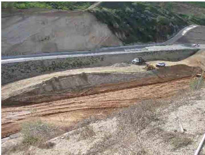
Photo 279: City Cell CC3B Construction: January 27, 2016
