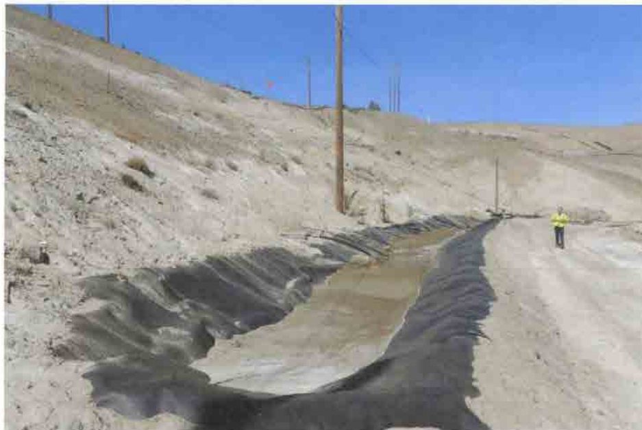
Photo 12: Seep collection at toe of future Cell CCII
