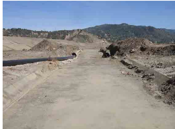
Photo 24: Basin A Outlet: February 24, 2016
