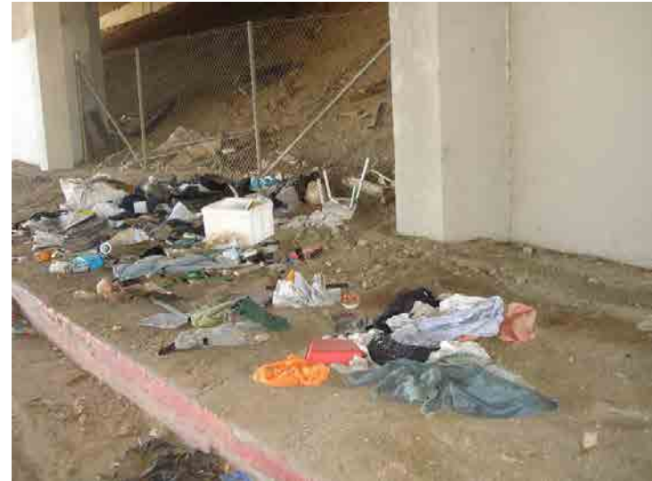
Photo 546: San Fernando Road Near I-5 Overpass: February 24, 2016
