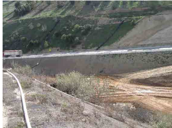
Photo 274: City Cell CC3B Construction: January 27, 2016
