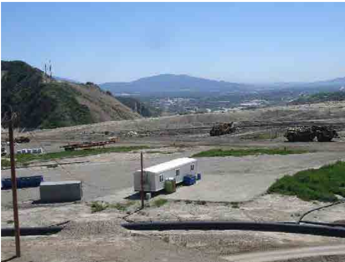
Photo 175: Site County Top Deck: March 23, 2016
