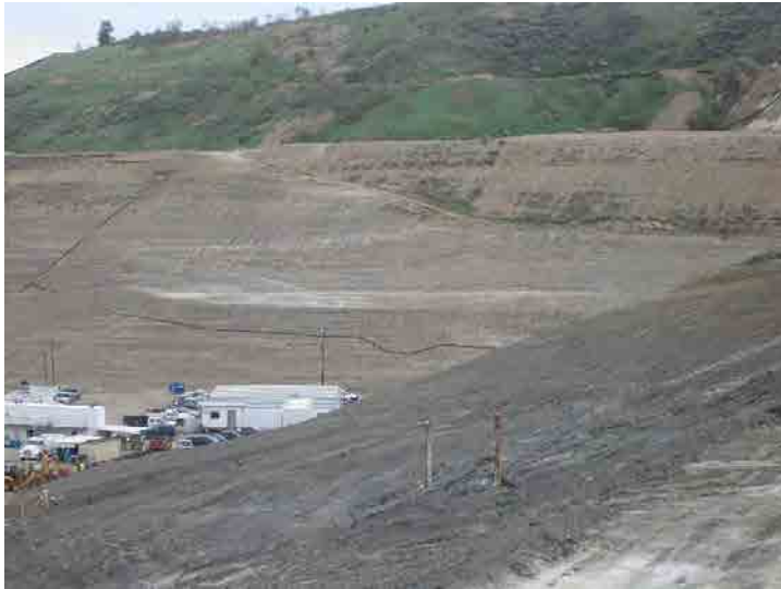
Photo 49: Site Grading South of Basin A: January 27, 2016
