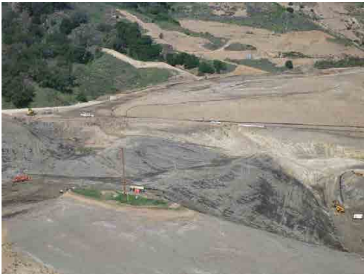
Photo 67: Site Grading South of Basin A: March 9, 2016
