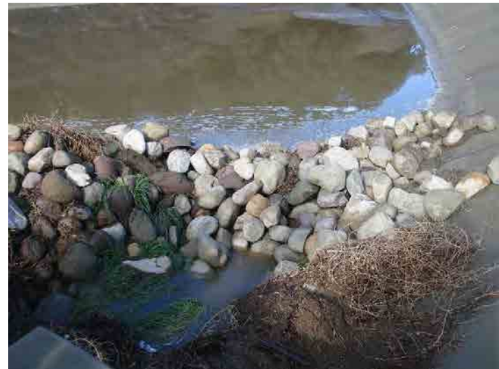
Photo 4: Basin A: January 7, 2016
