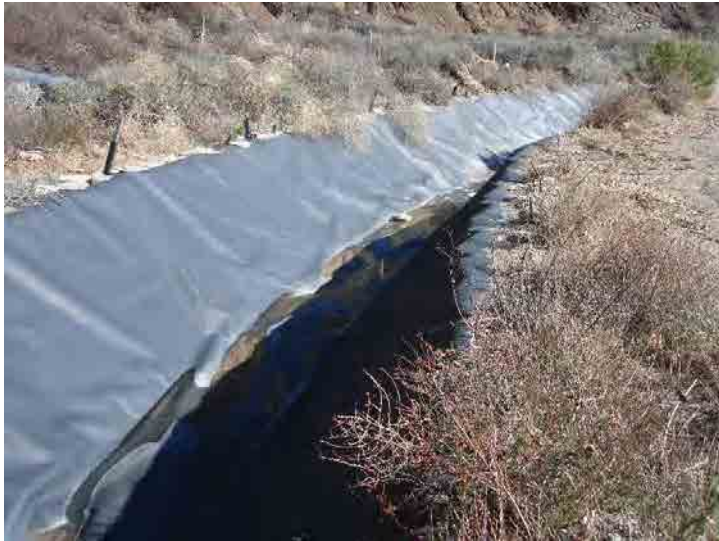
Photo 133: Basin D Outlet Channel: January 7, 2016
