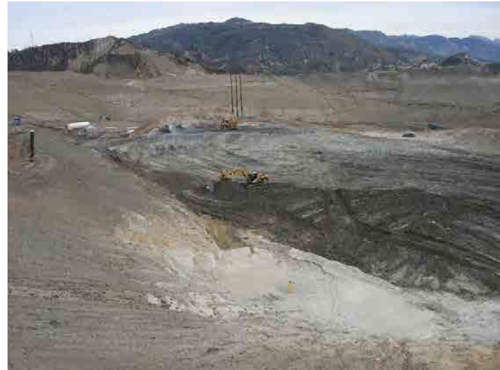
Photo 54: Site Grading South of Basin A: January 27, 2016
