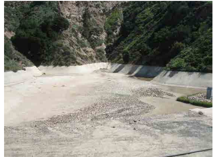
Photo 204: Basin B: March 23, 2016
