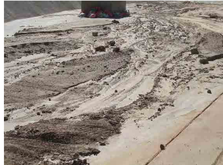
Photo 246: Terminal Basin: February 24, 2016
