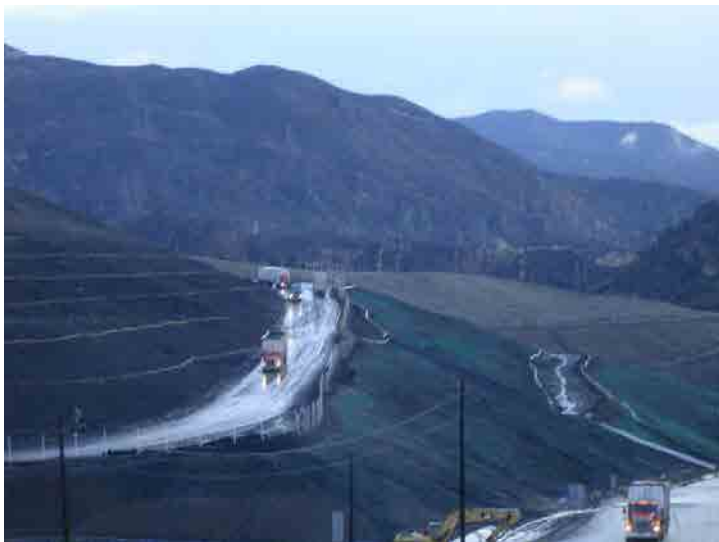
Photo 575: Haul Road to Working Face: January 7, 2016
