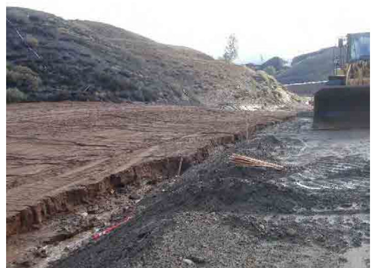
Photo 266: City Cell CC3B Construction: January 7, 2016
