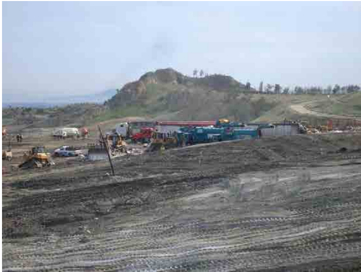
Photo 633: Site Working Area 200 pm: January 27, 2016
