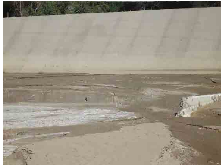
Photo 244: Terminal Basin: February 24, 2016
