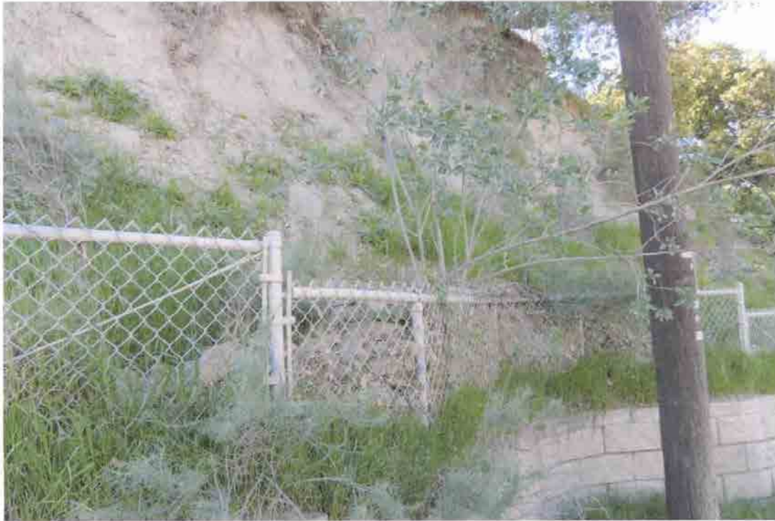
Photo 13: Soil accumulated against the wire fence at wall along San Fernando Road
