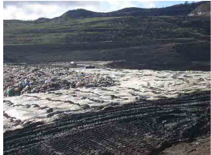
Photo 596: Site Working Area 1100 am: January 7, 2016
