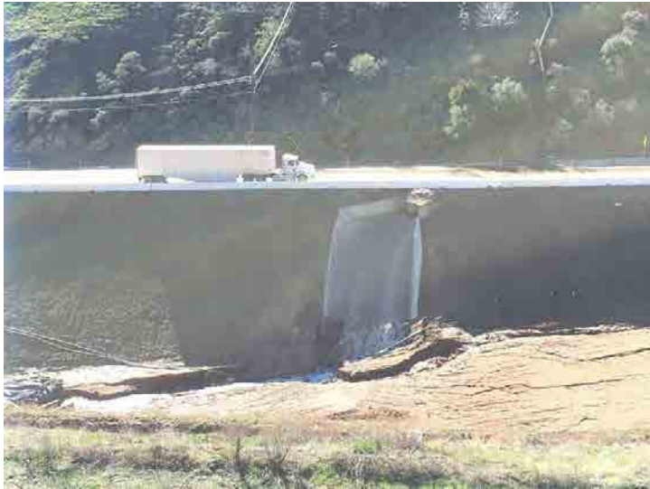
Photo 309: City South Access Road Drainage Control: January 7, 2016
