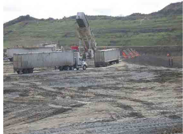
Photo 636: Site Working Area 200 pm: January 27, 2016
