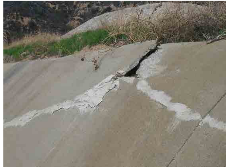
Photo 106: Westside Drainage Channel: January 27, 2016
