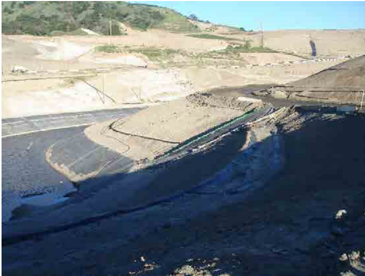
Photo 93: City Lined Drainage Lift Area: March 23, 2016
