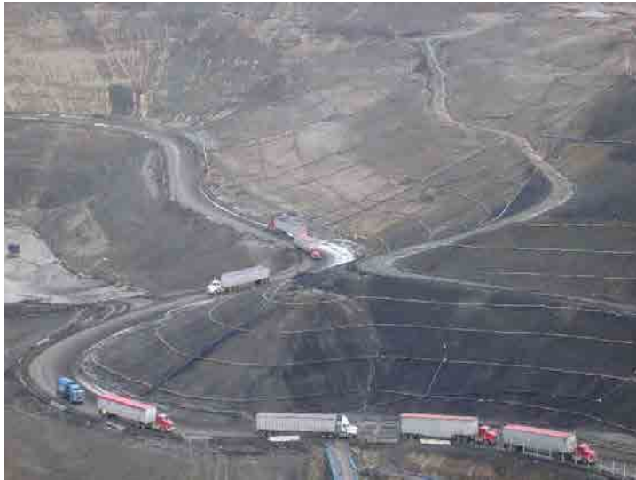
Photo 597: Site Working Area 200 pm: January 7, 2016
