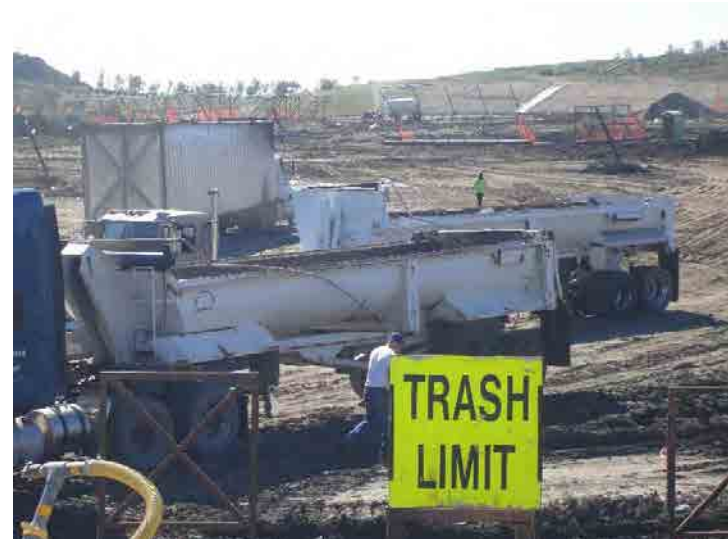
Photo 654: Site Working Area 1100am: March 9, 2016
