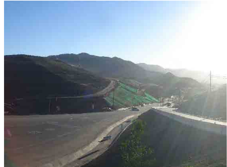
Photo 658: Site Working Area 800am: March 23, 2016
