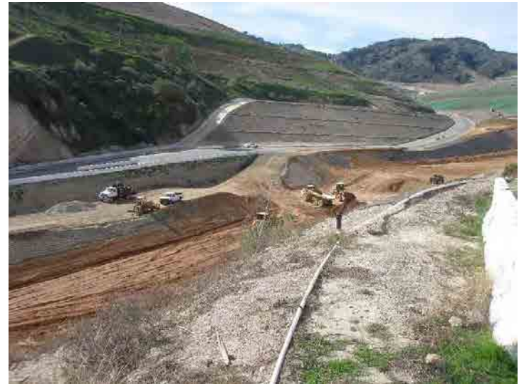
Photo 280: City Cell CC3B Construction: January 27, 2016
