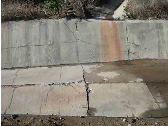
Photo 97: Westside Drainage Channel: January 7, 2016
