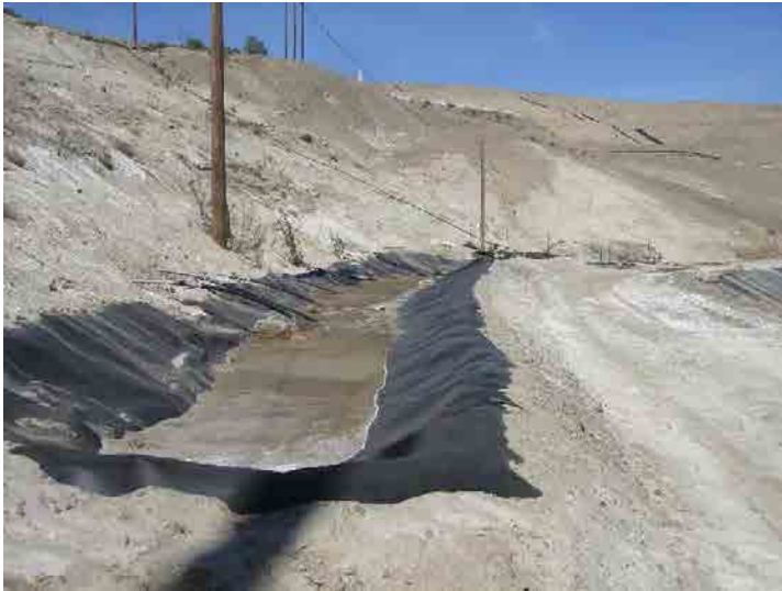
Photo 89: City Lined Drainage Lift Area: February 24, 2016
