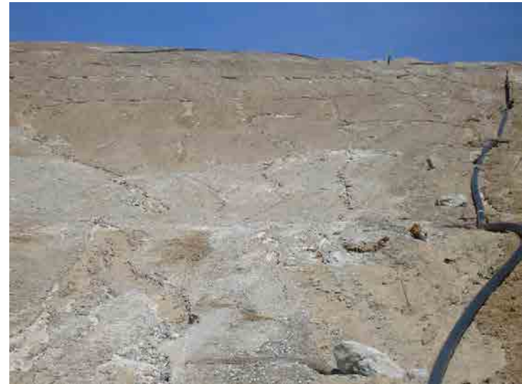
Photo 356: City Slope Erosion, Inert Waste Exposed: February 24, 2016
