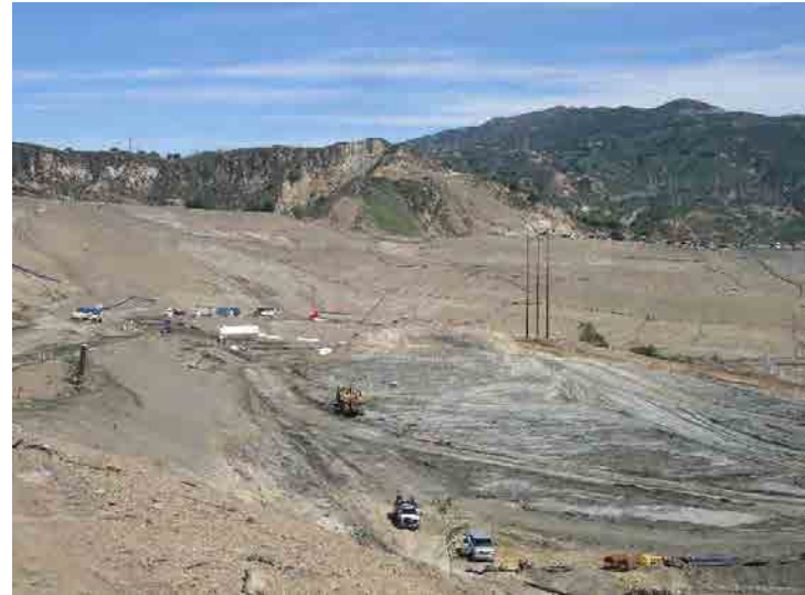
Photo 62: Site Grading South of Basin A: March 9, 2016
