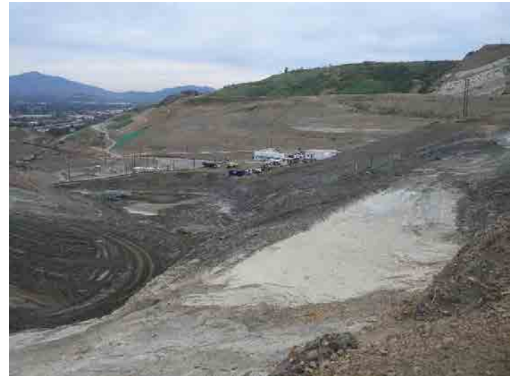
Photo 48: Site Grading South of Basin A: January 27, 2016
