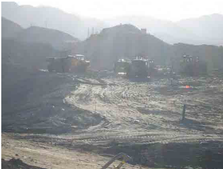
Photo 659: Site Working Area 800am: March 23, 2016
