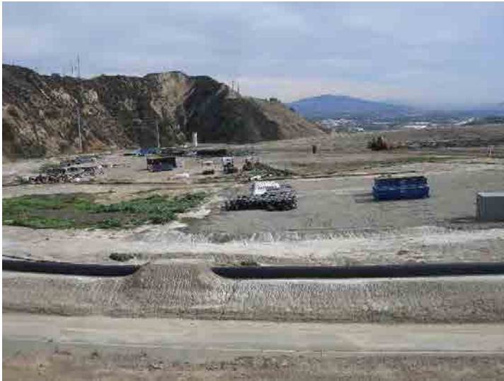
Photo 165: County Top Deck: January 27, 2016
