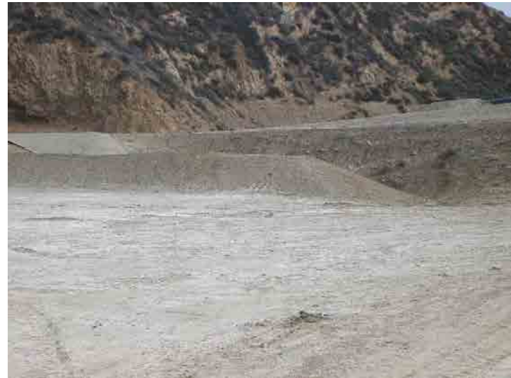
Photo 124: Basin D: January 27, 2016
