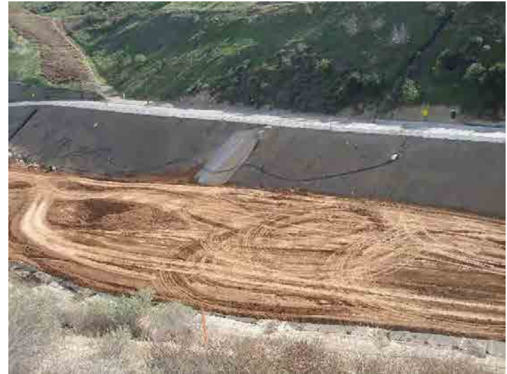
Photo 276: City Cell CC3B Construction: January 27, 2016
