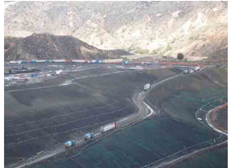
Photo 600: Site Working Area 2:00 pm: January 7, 2016
