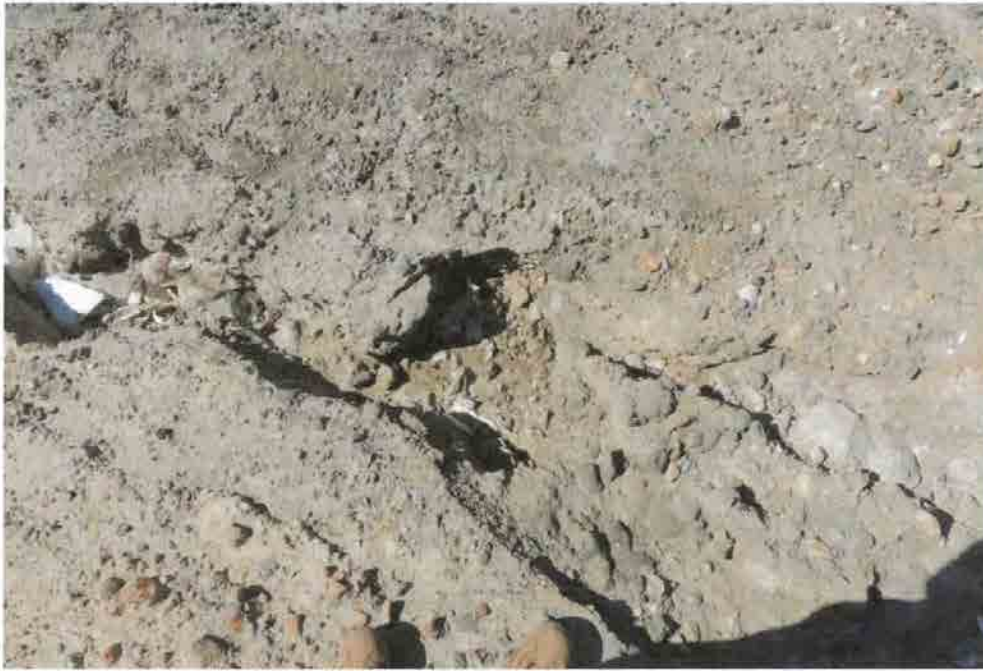
Photo 5: Deep gully on on side slope at Cell II showing refuse
