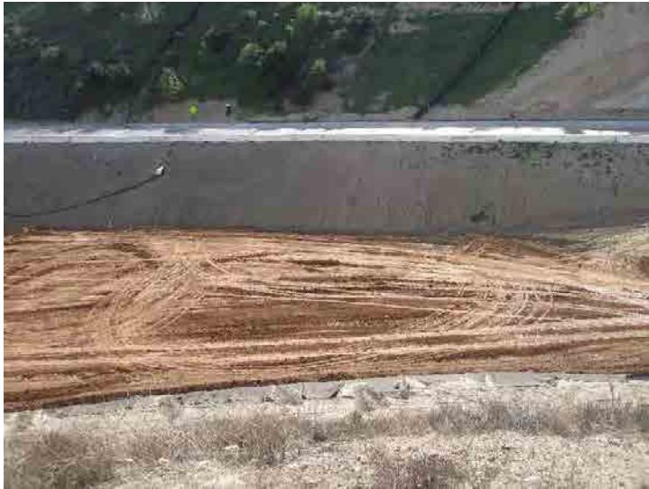
Photo 277: City Cell CC3B Construction: January 27, 2016
