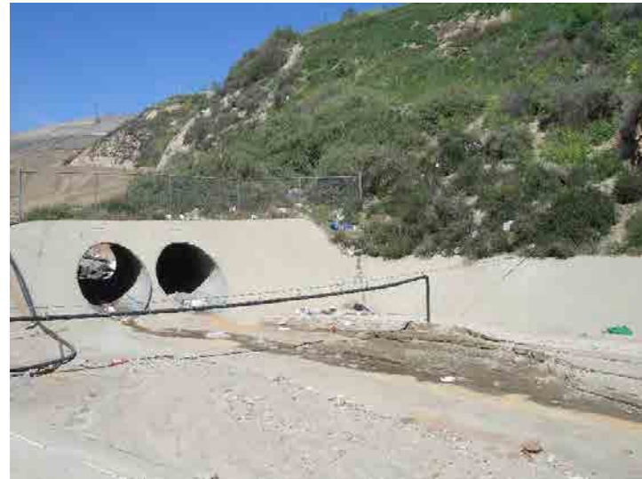
Photo 252: Terminal Basin Inlet: March 23, 2016
