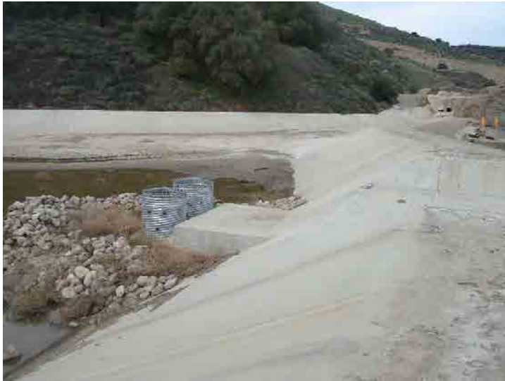
Photo 13: Basin A: January 27, 2015
