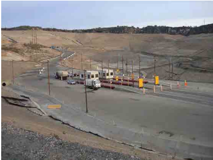
Photo 601: Site Working Area 830-930 am: January 27, 2016
