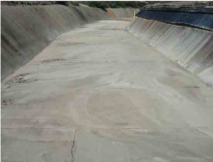
Photo 115: Westside Drainage Channel: March 9, 2016
