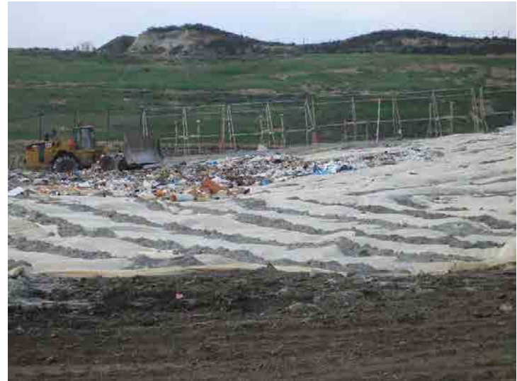
Photo 610: Site Working Area 830-930 am: January 27, 2016
