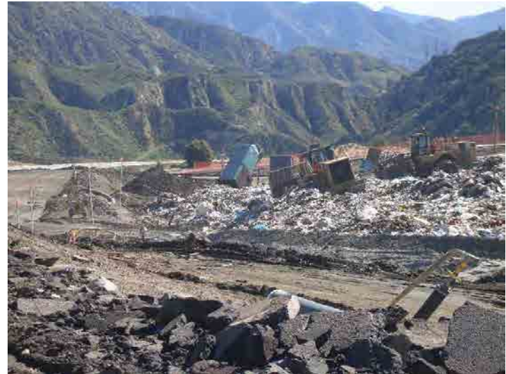
Photo 650: Site Working Area 1100am: March 9, 2016
