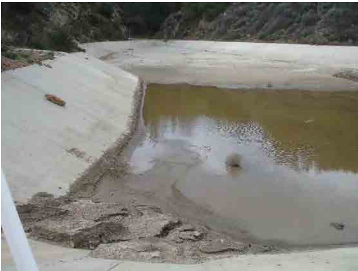
Photo 11: Basin A: January 27, 2015
