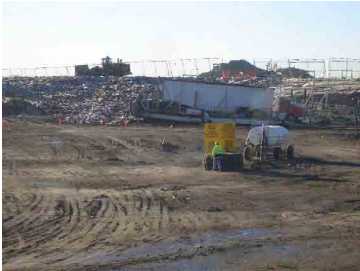
Photo 661: Site Working Area 800am: March 23, 2016
