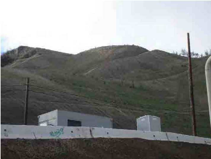
Photo 303: City South Access Road Drainage Control: January 7, 2016
