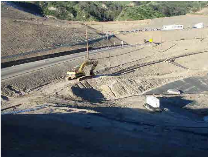
Photo 91: City Lined Drainage Lift Area: March 23, 2016
