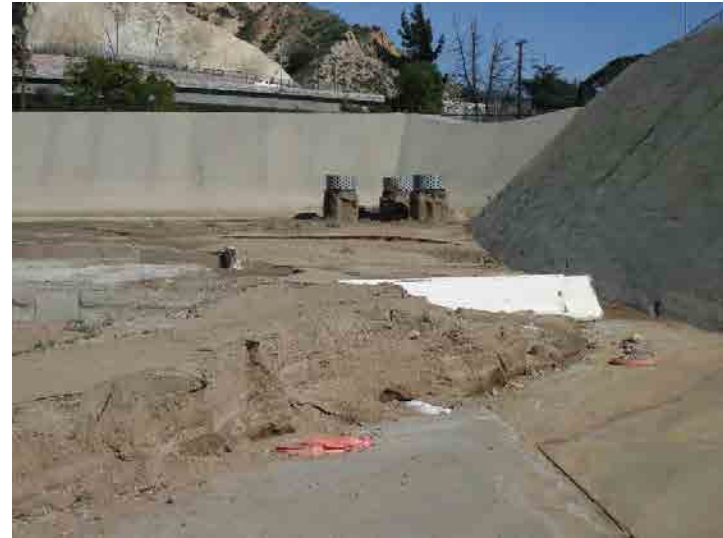
Photo 242: Terminal Basin: February 24, 2016
