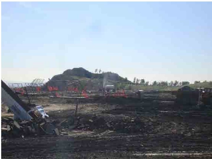
Photo 655: Site Working Area 1100am: March 9, 2016
