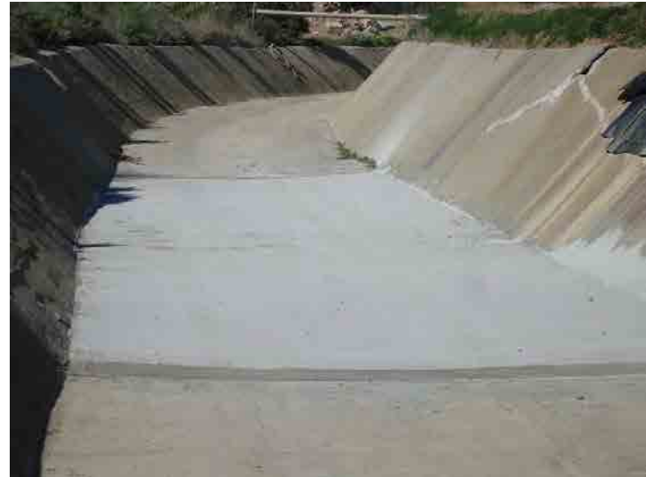
Photo 110: Westside Drainage Channel: February 24, 2016
