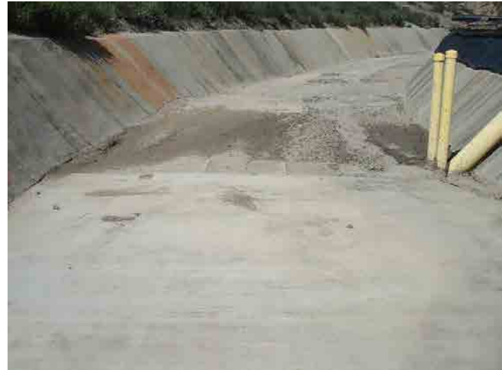
Photo 116: Westside Drainage Channel: March 9, 2016
