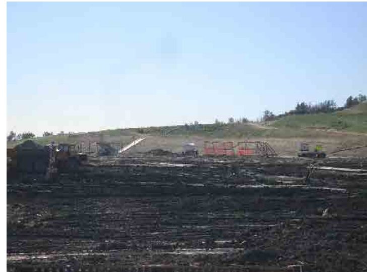
Photo 656: Site Working Area 1100am: March 9, 2016
