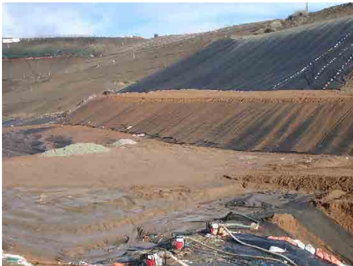
Photo 259: City Cell CC3B Construction: January 7, 2016
