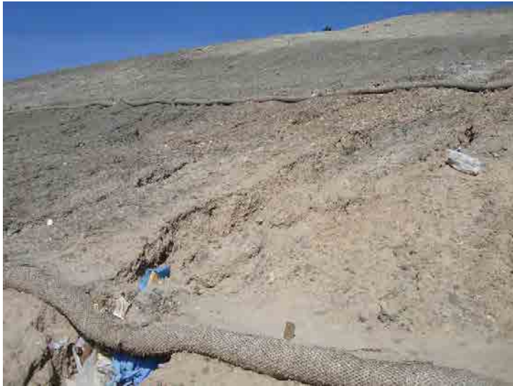
Photo 349: County South Facing Slope, Inert Waste Exposed: February 24, 2016
