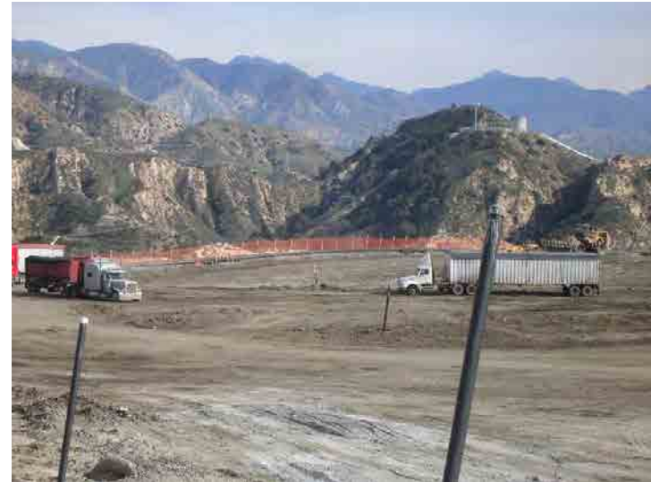
Photo 630: Site Working Area 200 pm: January 27, 2016
