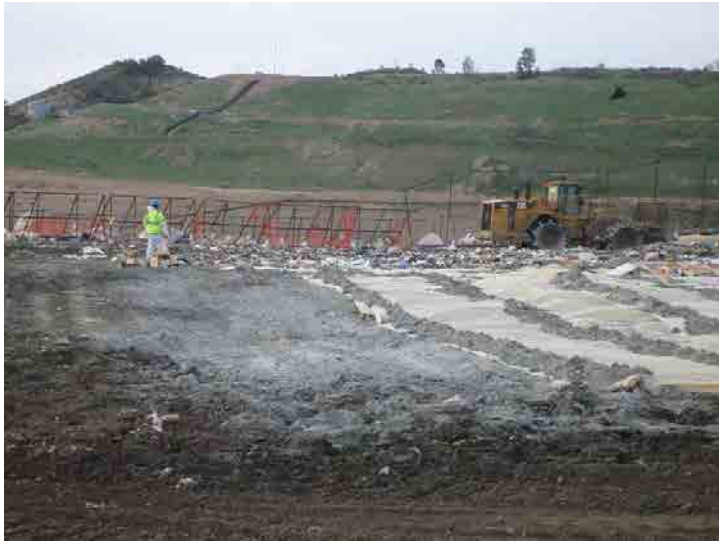
Photo 609: Site Working Area 830-930 am: January 27, 2016
