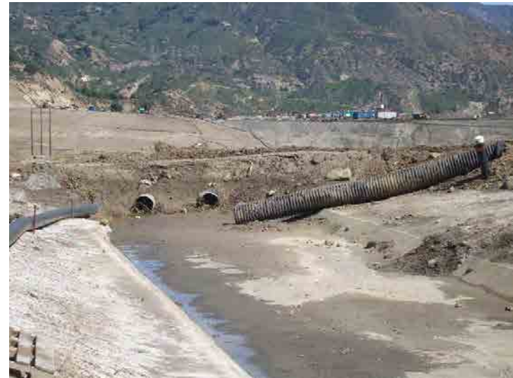
Photo 32: Basin A Outlet: March 9, 2016
