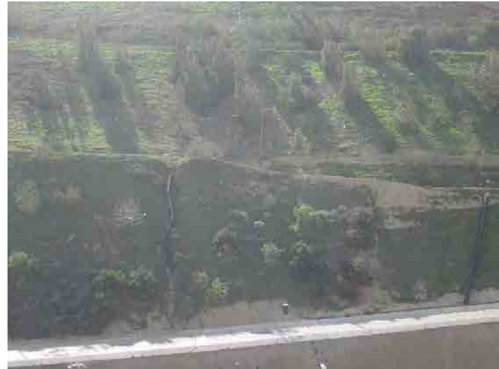
Photo 318: Main Access Road: January 27, 2016
