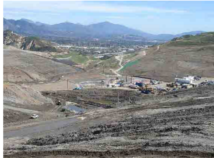
Photo 64: Site Grading South of Basin A: March 9, 2016
