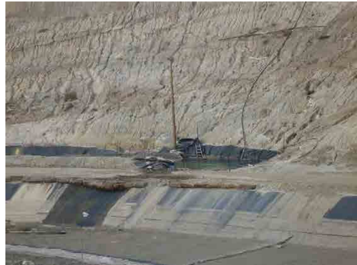
Photo 84: City Lined Drainage Lift Area: January 27, 2016
