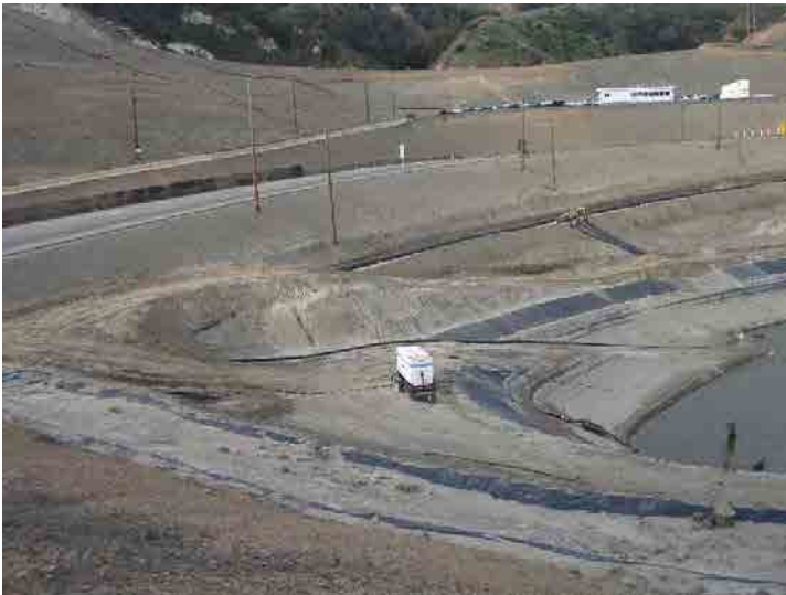
Photo 83: City Lined Drainage Lift Area: January 27, 2016
