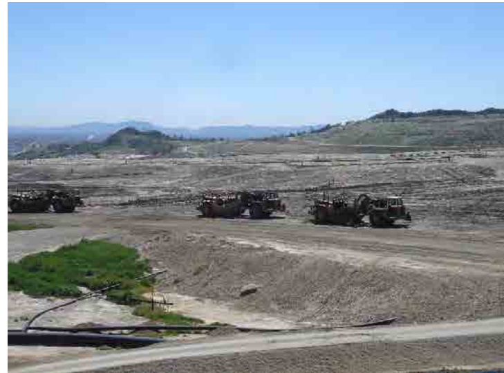
Photo 176: Site County Top Deck: March 23, 2016
