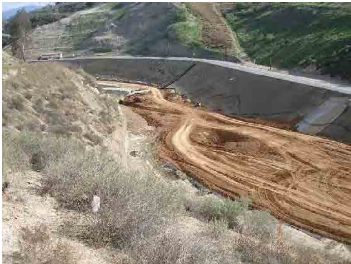
Photo 275: City Cell CC3B Construction: January 27, 2016
