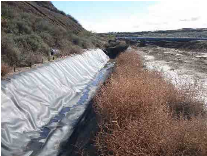
Photo 135: Basin D Outlet Channel: January 7, 2016
