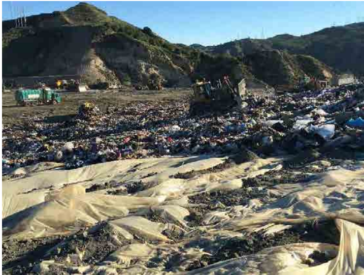
Photo 673: Site Working Area 800am: March 23, 2016
