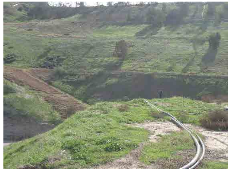
Photo 312: Main Access Road: January 27, 2016
