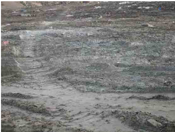
Photo 619: Site Working Area 830-930 am: January 27, 2016
