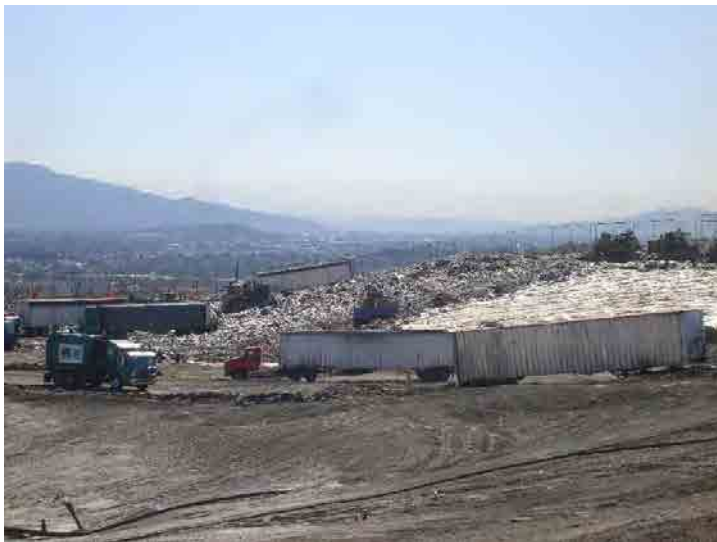
Photo 643: Site Working Area 1200am: February 24, 2016
