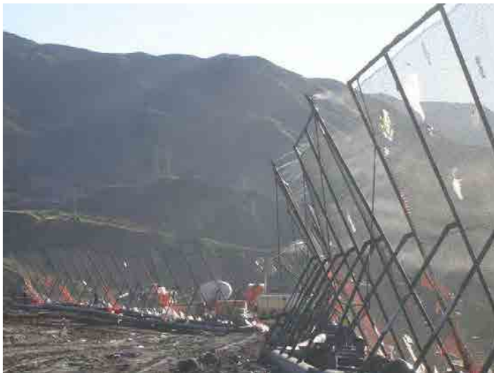
Photo 675: Site Working Area 800am: March 23, 2016
