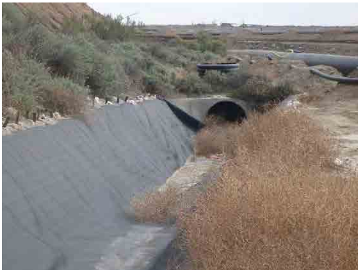
Photo 139: Basin D Outlet Channel: January 27, 2016
