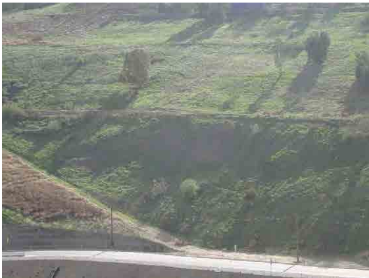
Photo 315: Main Access Road: January 27, 2016
