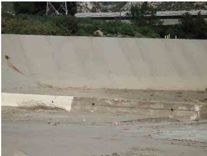
Photo 243: Terminal Basin: February 24, 2016
