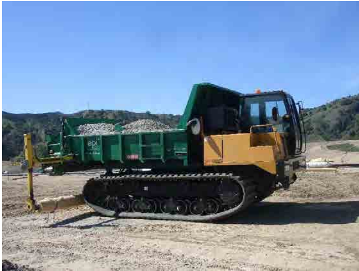
Photo 645: Site Working Area 1200am: February 24, 2016
