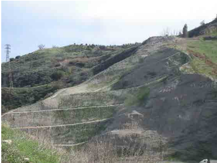
Photo 313: Main Access Road: January 27, 2016
