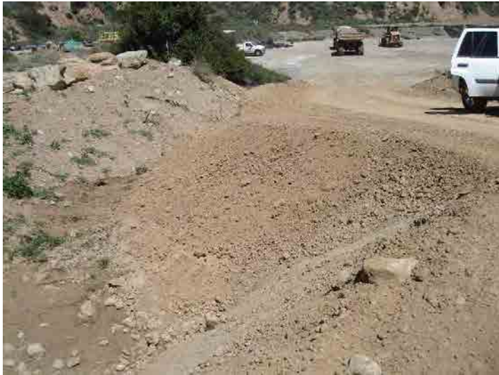
Photo 129: Hillside Drainage into Basin D: March 23, 2016
