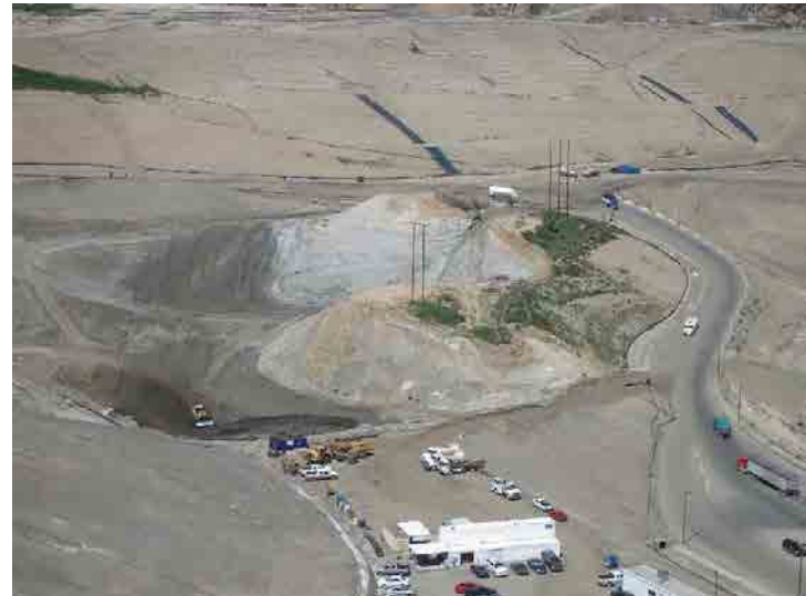
Photo 72: Site Grading South of Basin A: March 23, 2016
