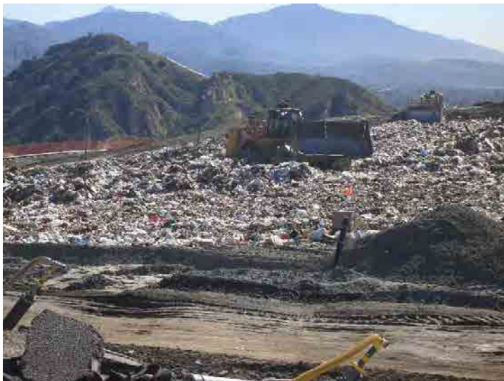
Photo 651: Site Working Area 1100am: March 9, 2016
