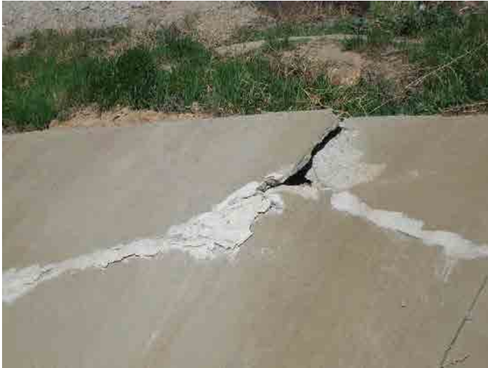
Photo 113: Westside Drainage Channel: February 24, 2016
