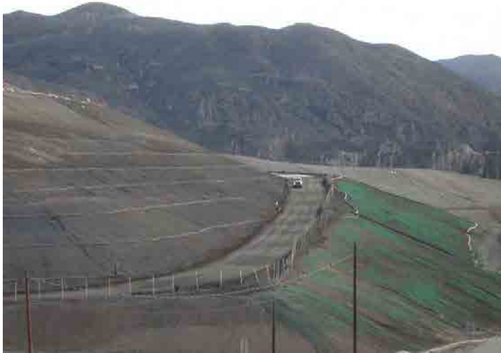
Photo 605: Site Working Area 830-930 am: January 27, 2016
