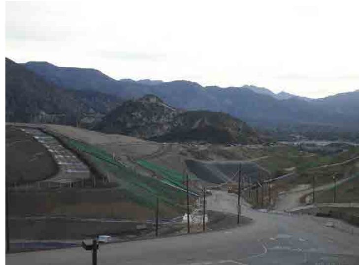
Photo 342: City Slope Erosion Control: January 27, 2016
