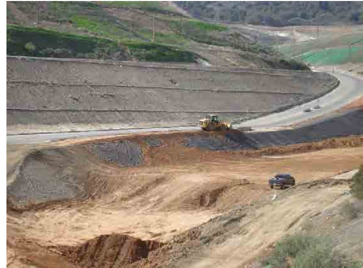
Photo 270: City Cell CC3B Construction: January 27, 2016
