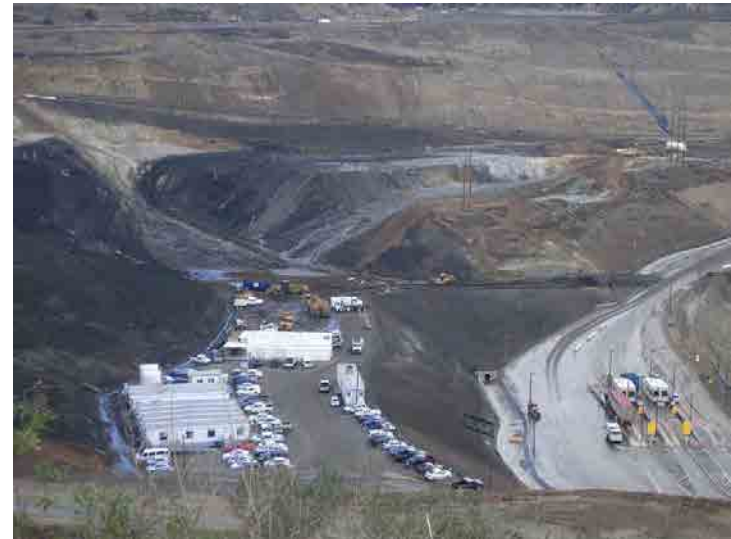
Photo 44: Site Grading South of Basin A: January 7, 2016
