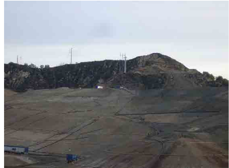
Photo 606: Site Working Area 830-930 am: January 27, 2016
