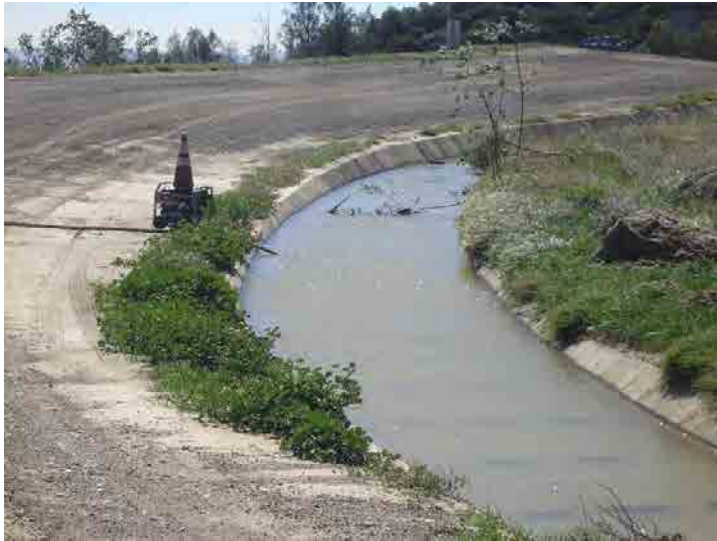
Photo 413: City Deck B Drainage Channel: March 9, 2016
