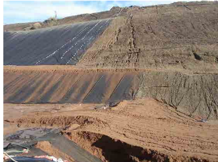
Photo 260: City Cell CC3B Construction: January 7, 2016
