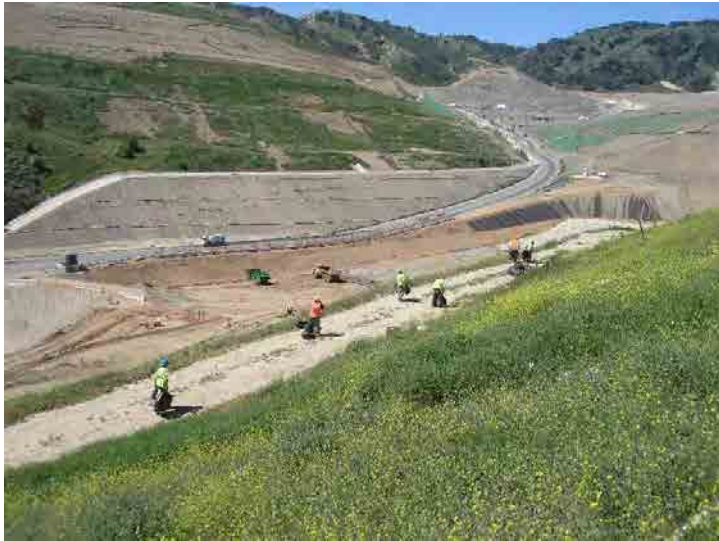
Photo 329: Main Access Road: March 23, 2016
