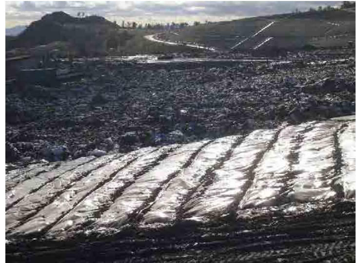
Photo 594: Site Working Area 1100 am: January 7, 2016
