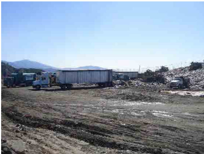
Photo 639: Site Working Area 1100am: February 24, 2016
