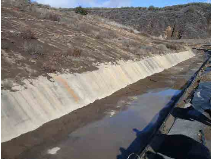
Photo 101: Westside Drainage Channel: January 7, 2016
