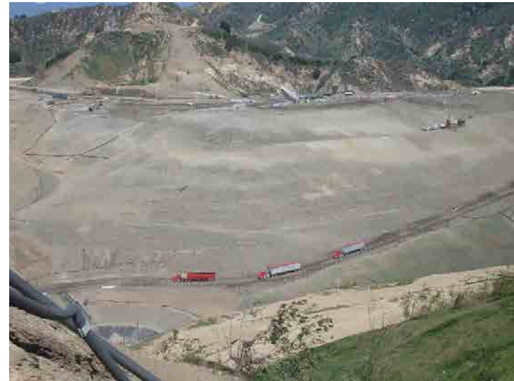
Photo 680: Site Working Area 100 pm: March 23, 2016
