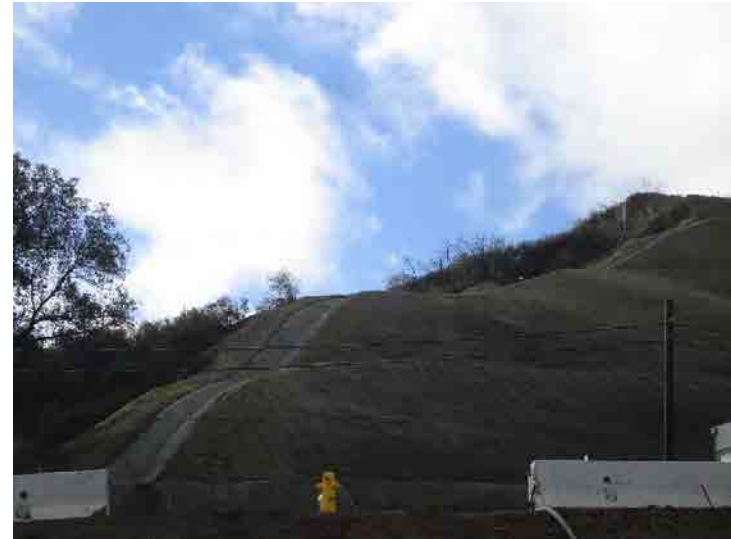
Photo 302: City South Access Road Drainage Control: January 7, 2016
