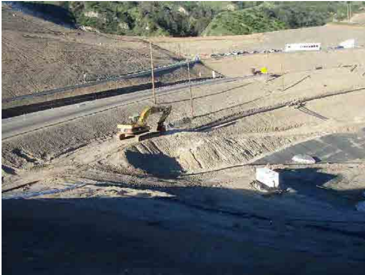
Photo 301: City South Access Road Drainage Control: January 7, 2016
