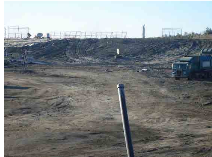
Photo 662: Site Working Area 800am: March 23, 2016
