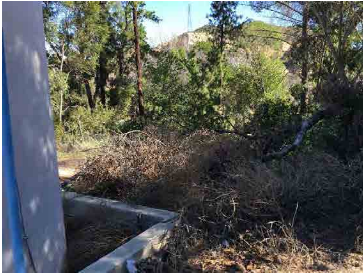
Photo 501: Leachate Treatment Facility: February 24, 2016
