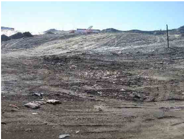
Photo 647: Site Working Area 1200am: February 24, 2016
