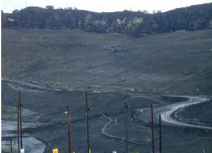
Photo 571: Haul Road to Working Face: January 7, 2016
