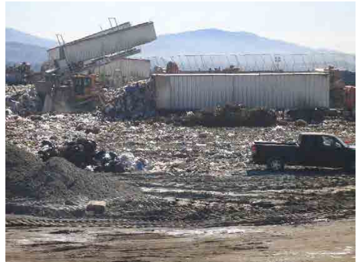
Photo 652: Site Working Area 1100am: March 9, 2016
