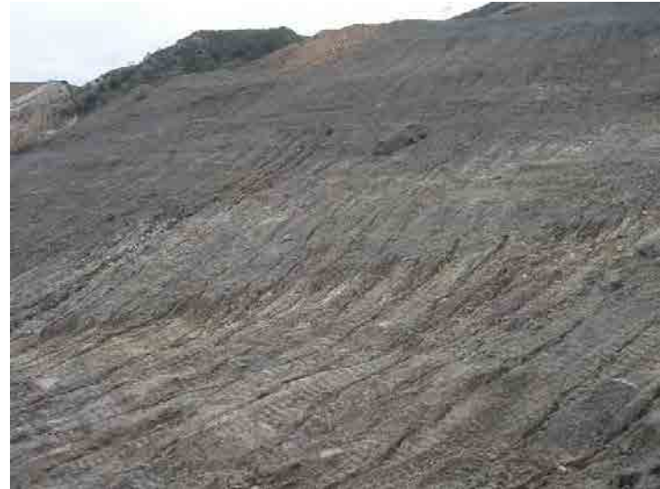
Photo 52: Site Grading South of Basin A: January 27, 2016
