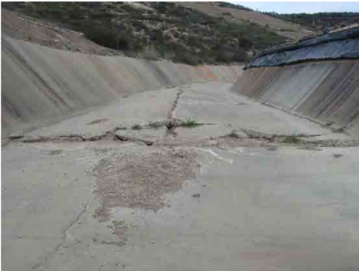
Photo 103: Westside Drainage Channel: January 27, 2016
