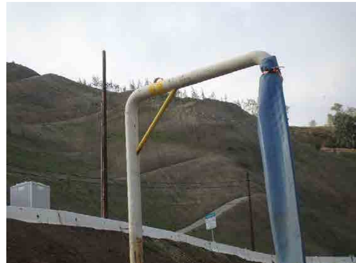
Photo 304: City South Access Road Drainage Control: January 7, 2016
