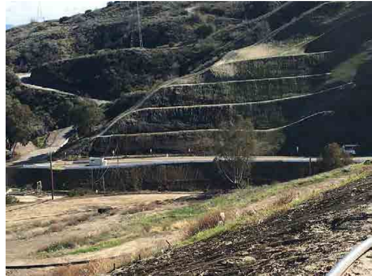
Photo 306: City South Access Road Drainage Control: January 7, 2016
