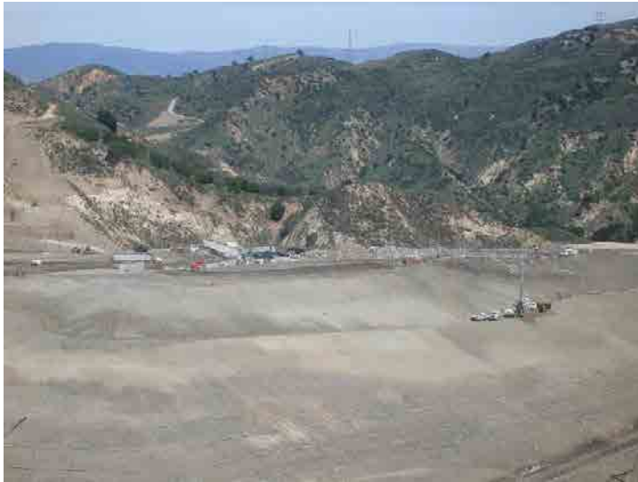
Photo 681: Site Working Area 100 pm: March 23, 2016
