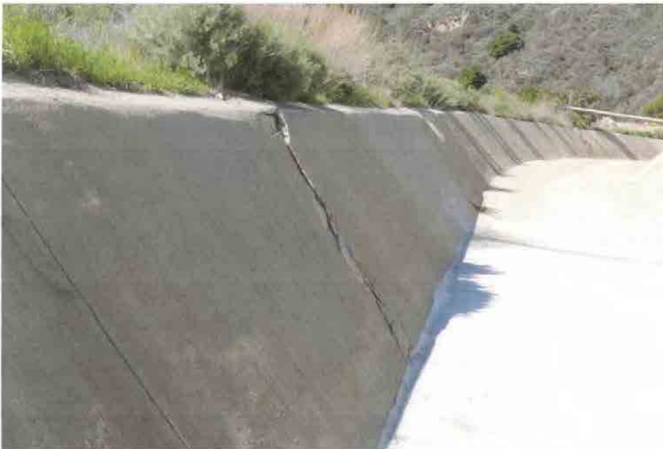
Photo 2: Crack on side wall channel between Basin A and Basin D
