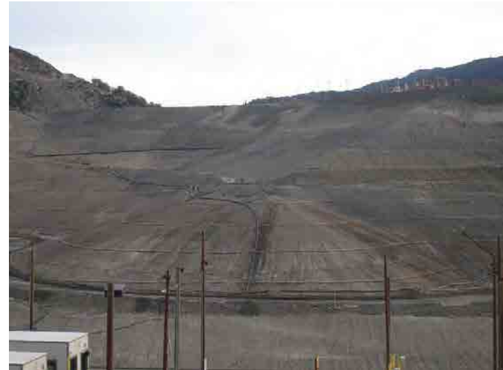
Photo 340: City Slope Erosion Control: January 27, 2016
