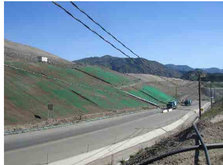
Photo 360: City Slope Erosion Control: February 24, 2016
