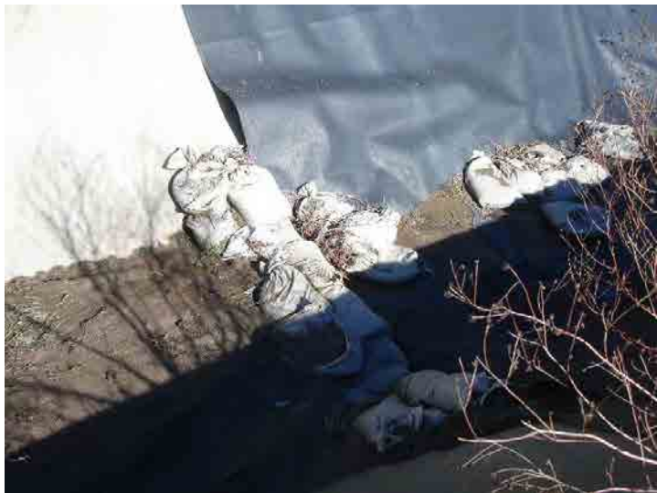
Photo 131: Basin D Outlet Channel: January 7, 2016
