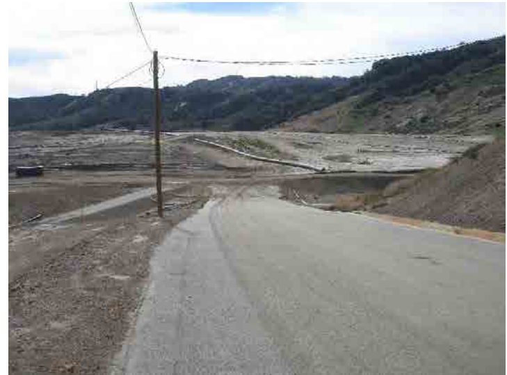
Photo 168: County Top Deck: January 27, 2016
