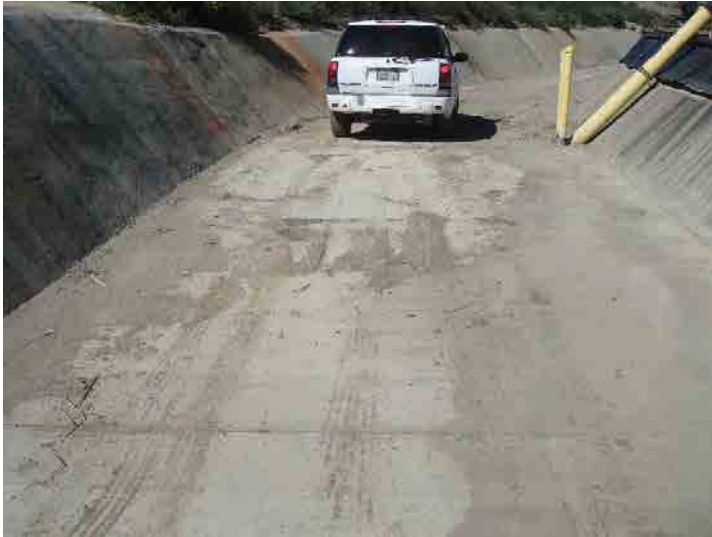
Photo 109: Westside Drainage Channel: February 24, 2016
