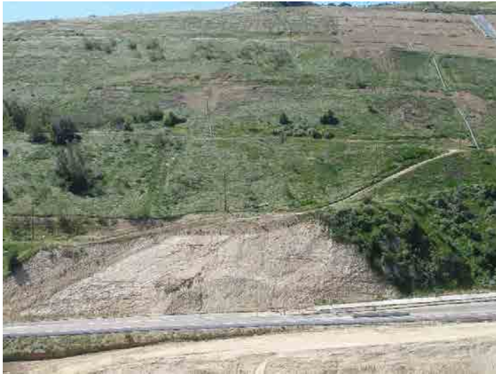
Photo 325: Main Access Road: March 23, 2016
