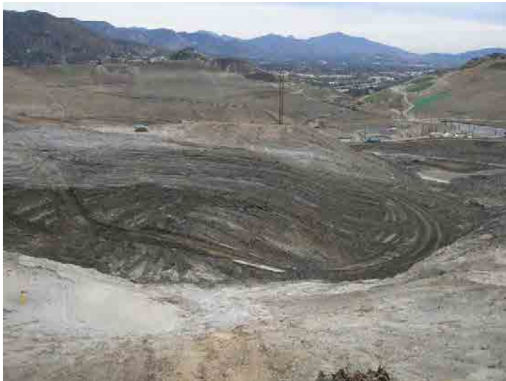
Photo 55: Site Grading South of Basin A: January 27, 2016
