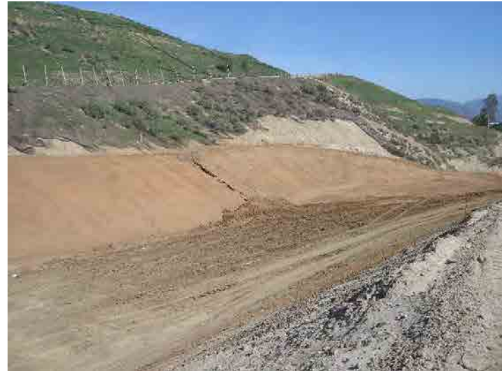
Photo 286: City Cell CC3B Construction: February 24, 2016
