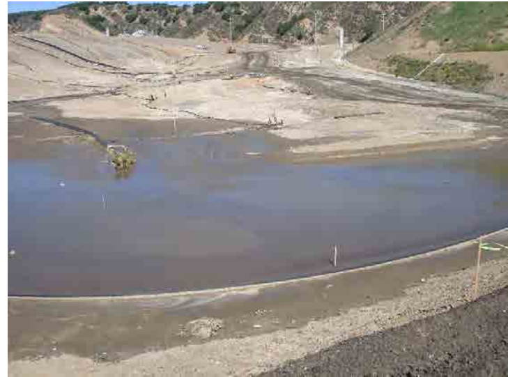
Photo 366: Ponding on City Top Deck: March 9, 2016
