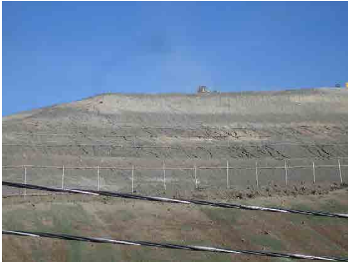
Photo 637: Site Working Area 1100am: February 24, 2016
