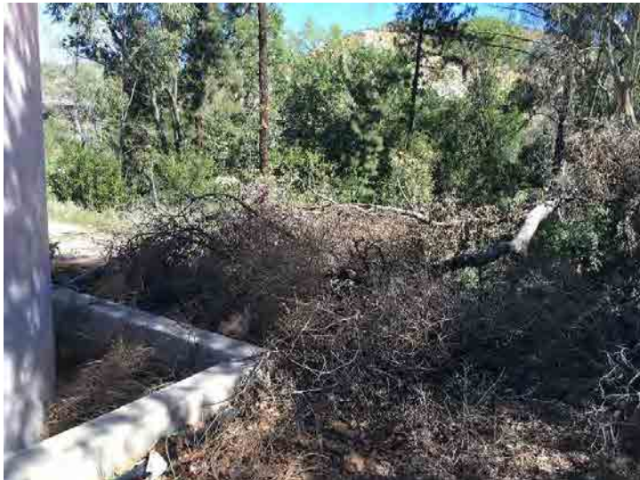
Photo 503: Leachate Treatment Facility: March 9, 2016
