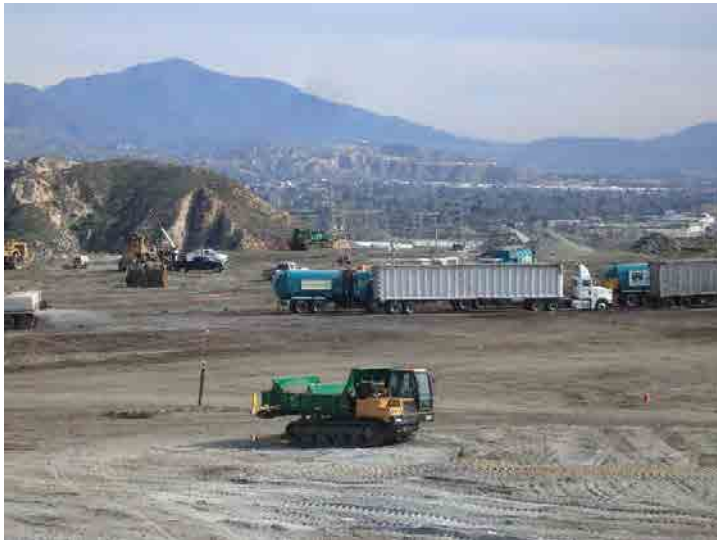
Photo 631: Site Working Area 200 pm: January 27, 2016
