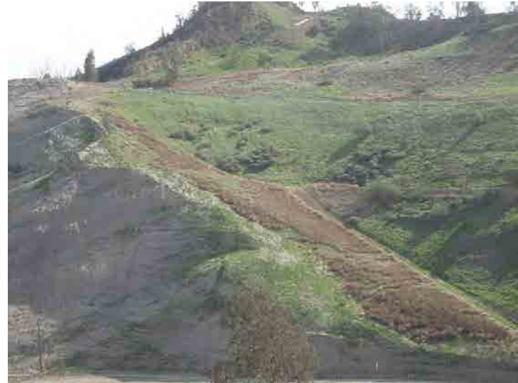
Photo 314: Main Access Road: January 27, 2016
