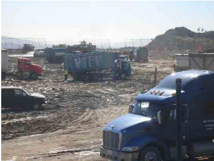
Photo 653: Site Working Area 1100am: March 9, 2016
