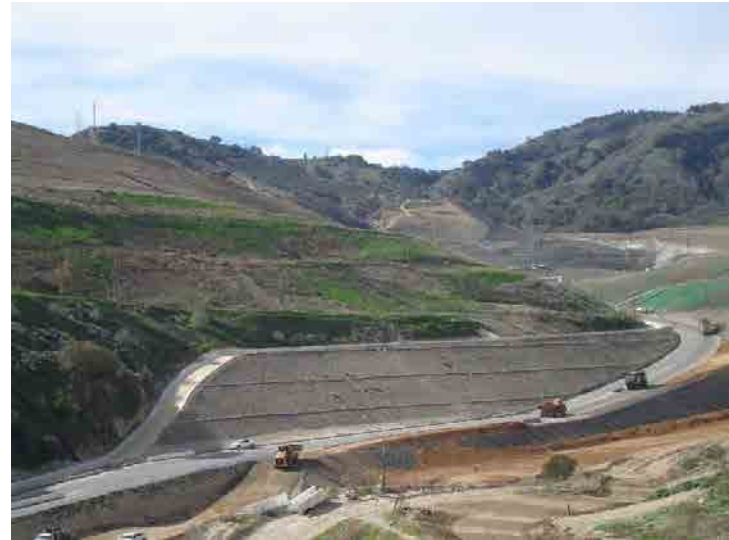
Photo 268: City Cell CC3B Construction: January 27, 2016
