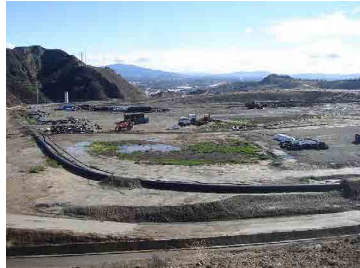
Photo 160: County Top Deck: January 7, 2016
