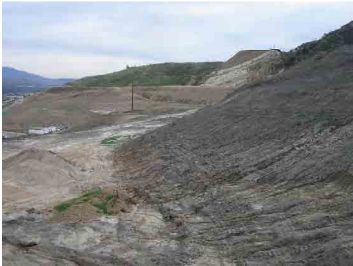
Photo 51: Site Grading South of Basin A: January 27, 2016
