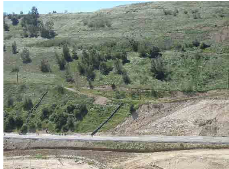
Photo 324: Main Access Road: March 23, 2016
