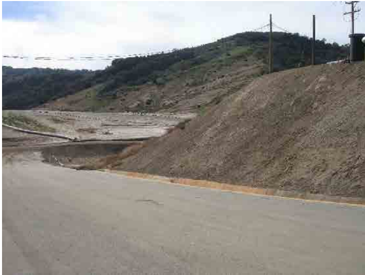
Photo 169: County Top Deck: January 27, 2016
