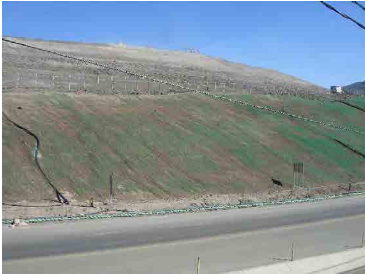
Photo 361: City Slope Erosion Control: February 24, 2016
