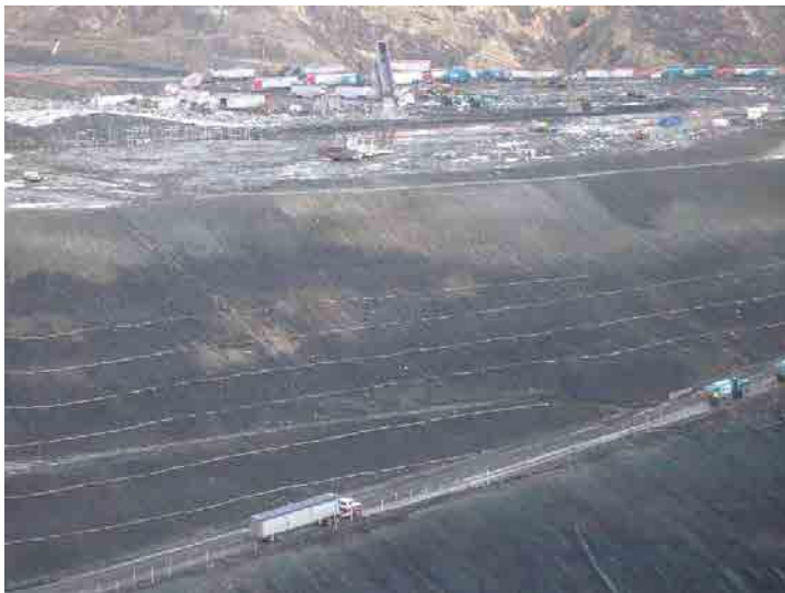
Photo 599: Site Working Area 200 pm: January 7, 2016
