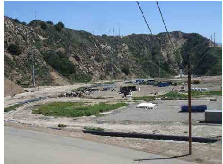
Photo 174: Site County Top Deck: March 23, 2016
