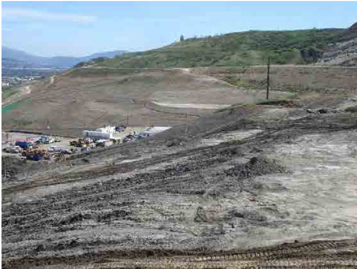
Photo 65: Site Grading South of Basin A: March 9, 2016
