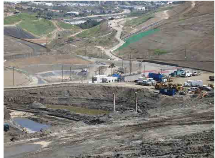
Photo 74: Oil Well Casings to be Abandoned: March 9, 2016
