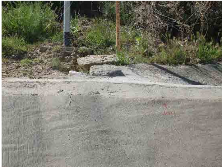
Photo 117: Westside Drainage Channel: March 9, 2016
