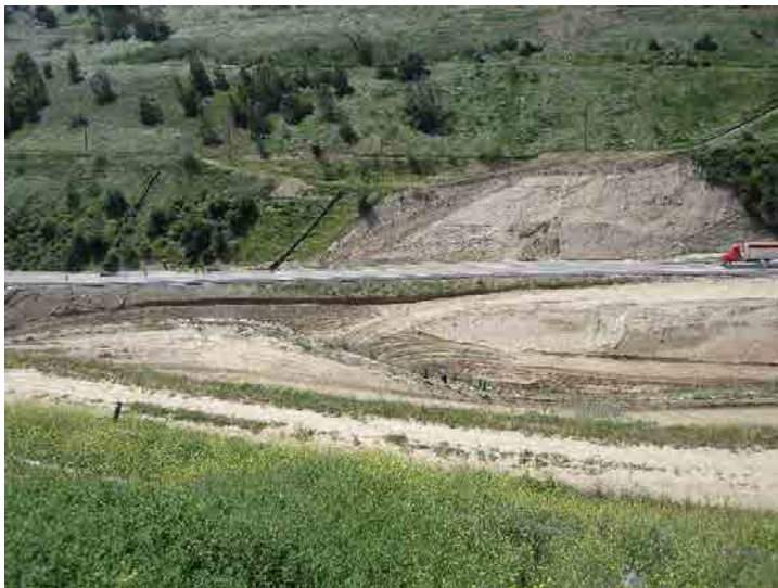
Photo 327: Main Access Road: March 23, 2016
