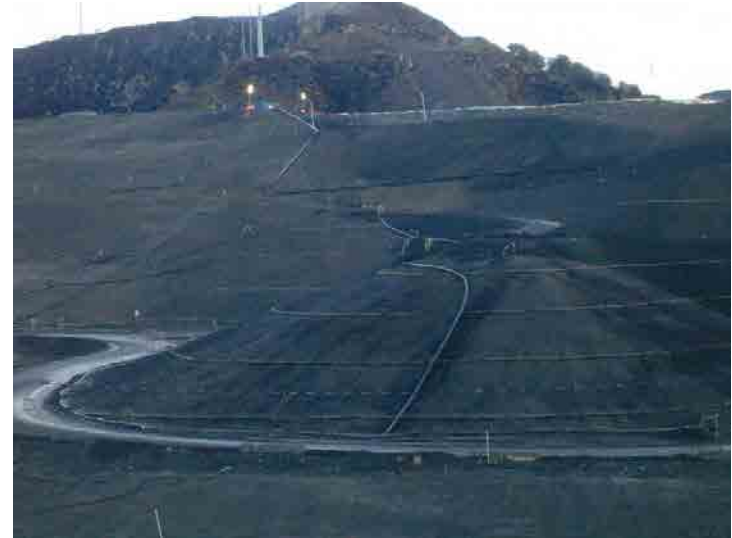
Photo 572: Haul Road to Working Face: January 7, 2016
