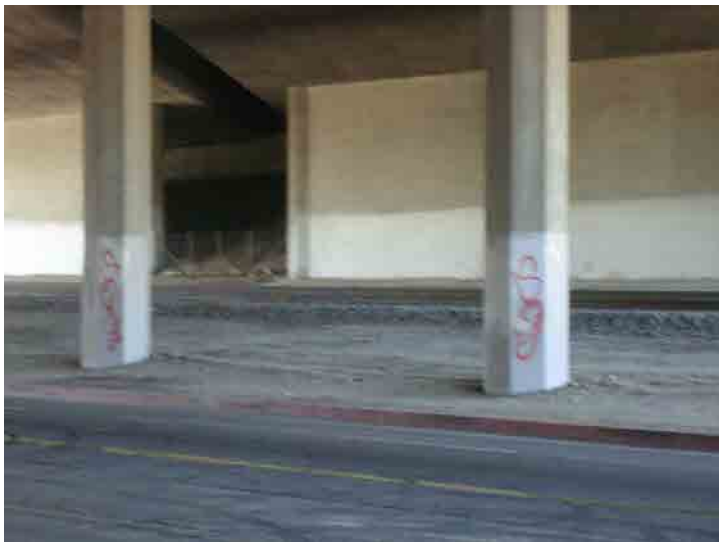
Photo 555: San Fernando Road Near I-5 Overpass: March 9, 2016
