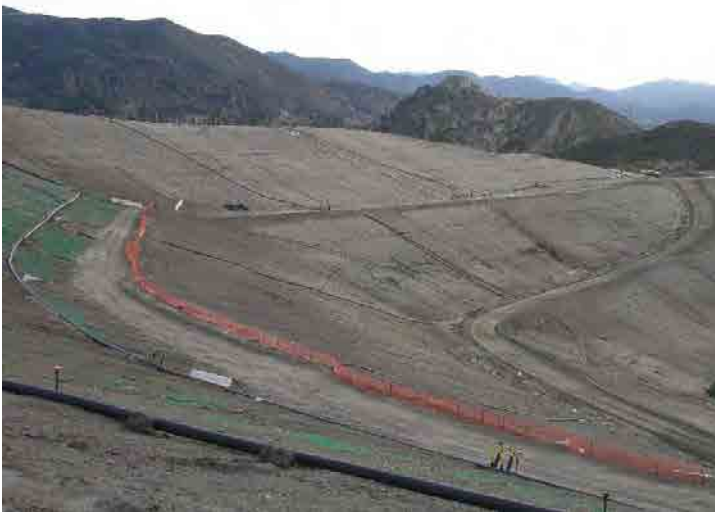
Photo 343: City Slope Erosion Control: January 27, 2016
