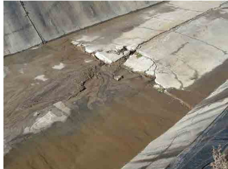
Photo 94: Westside Drainage Channel: January 7, 2016
