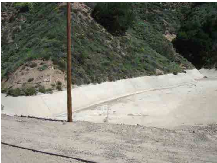
Photo 203: Basin B: March 23, 2016
