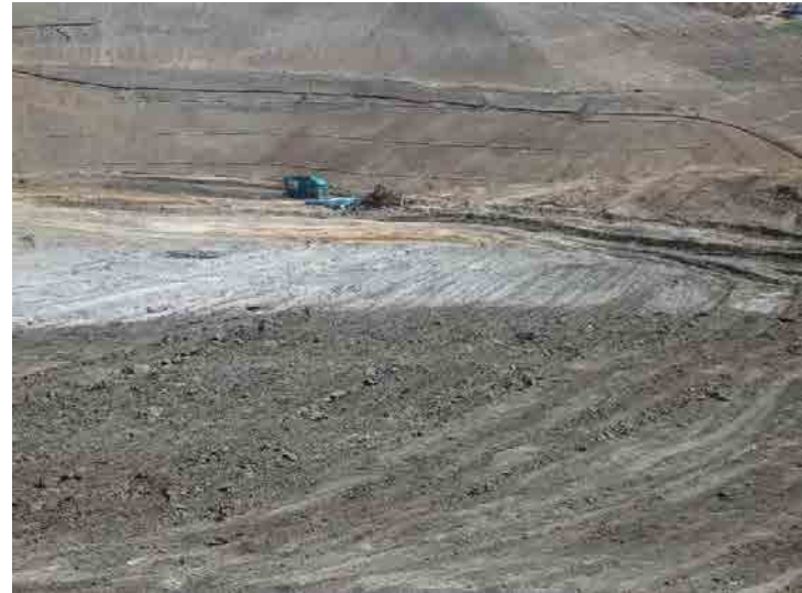
Photo 58: Site Grading South of Basin A: February 24, 2016
