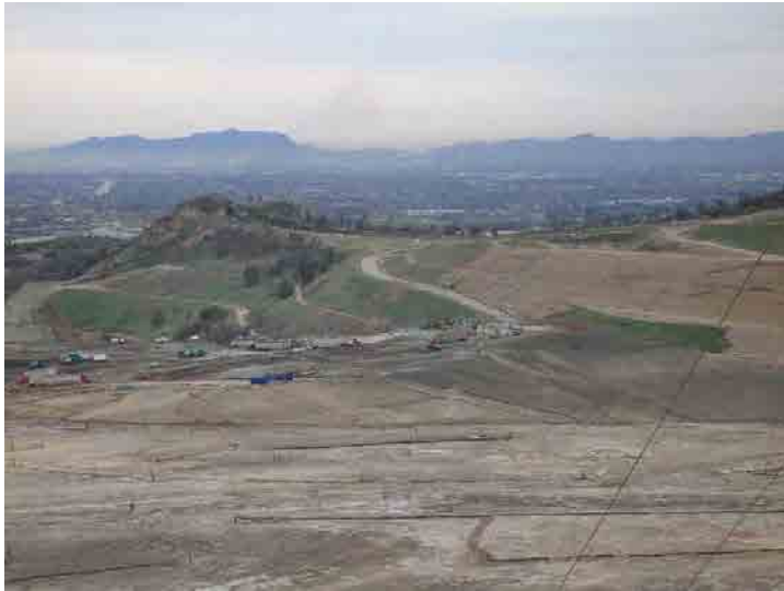
Photo 629: Site Working Area 12 noon: January 27, 2016
