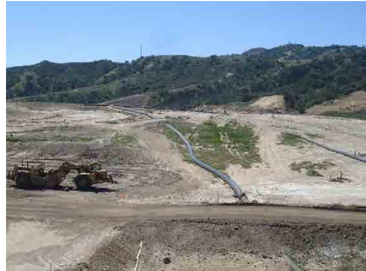
Photo 178: Site County Top Deck: March 23, 2016
