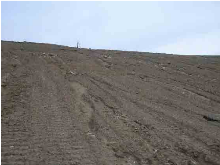
Photo 335: County South Slope Inert Waste Exposed: January 27, 2016
