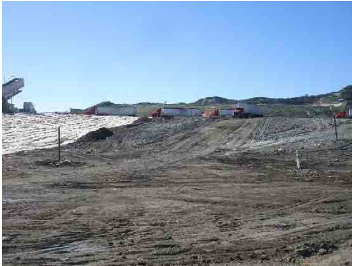
Photo 641: Site Working Area 1100am: February 24, 2016
