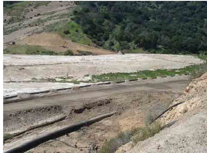
Photo 180: Site County Top Deck: March 23, 2016
