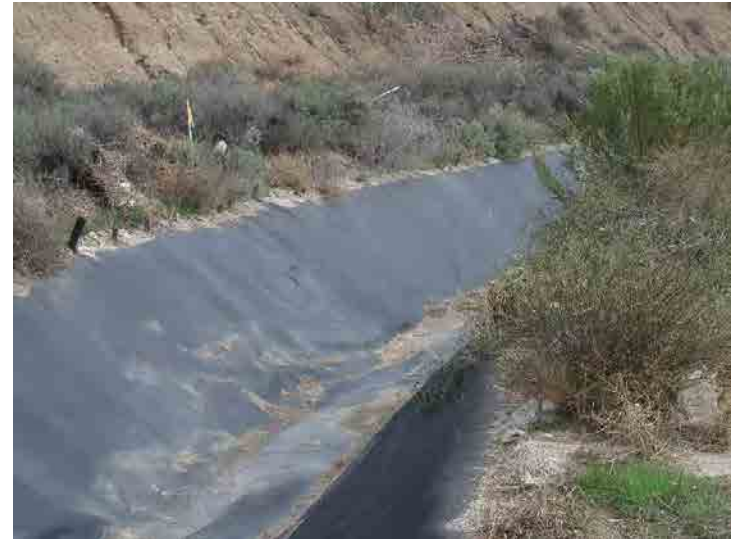
Photo 138: Basin D Outlet Channel: January 27, 2016
