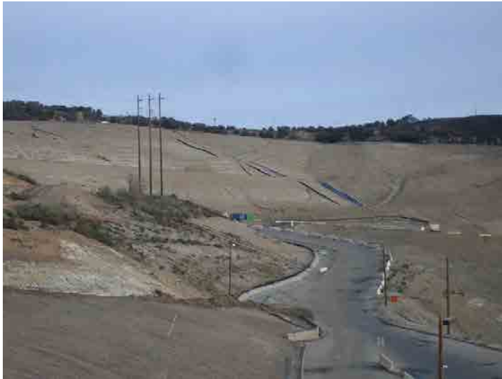
Photo 337: County South Slope Erosion Control: January 27, 2016
