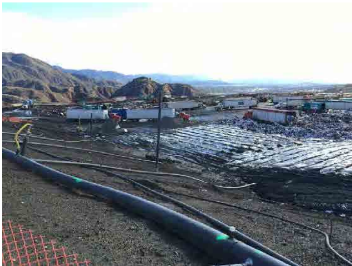
Photo 587: Site Working Area 1000 AM: January 7, 2016
