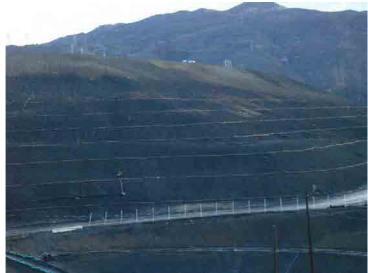
Photo 574: Haul Road to Working Face: January 7, 2016
