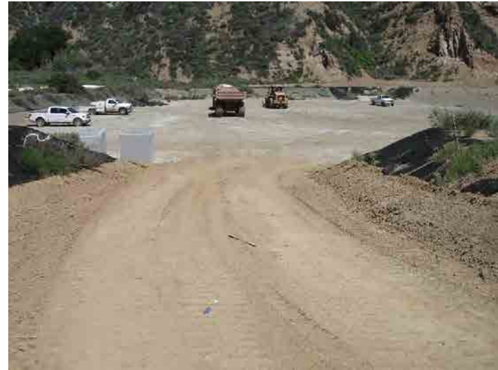
Photo 130: Hillside Drainage into Basin D: March 23, 2016
