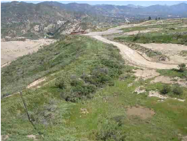
Photo 419: City Mitigation Deck A: March 23, 2016
