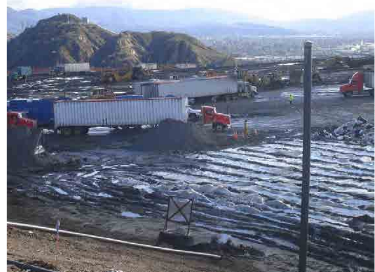
Photo 592: Site Working Area 1100 am: January 7, 2016
