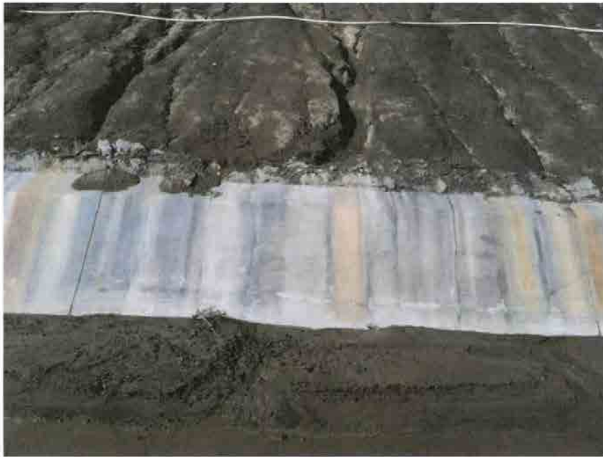
Photo 7: Sediment into channel between Basin A and Basin D
