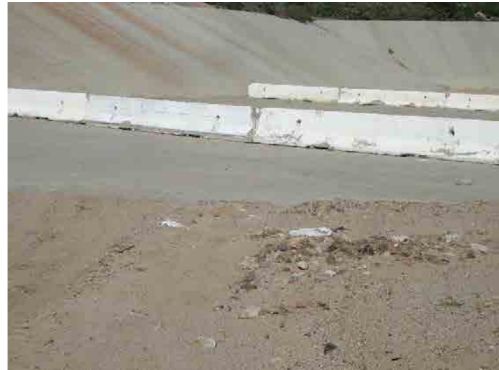
Photo 240: Terminal Basin: February 24, 2016
