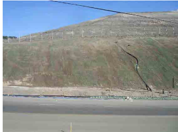
Photo 362: City Slope Erosion Control: February 24, 2016
