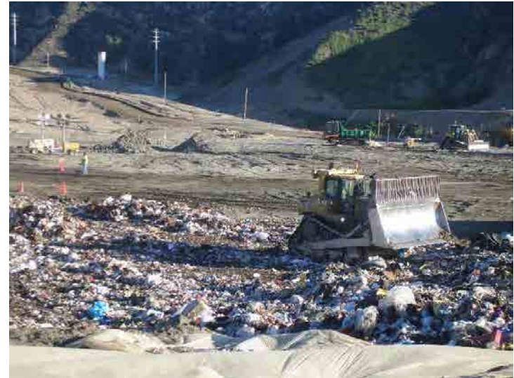
Photo 670: Site Working Area 800am: March 23, 2016
