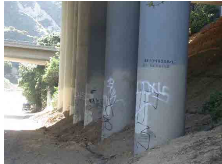
Photo 564: San Fernando Road Near I-5 Overpass: March 9, 2016
