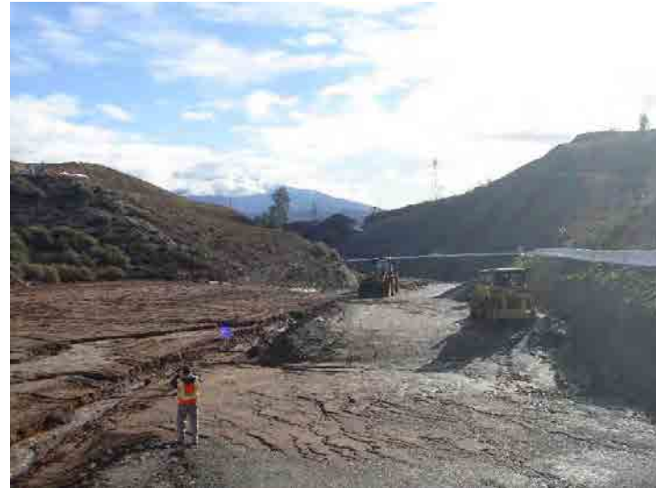
Photo 264: City Cell CC3B Construction: January 7, 2016
