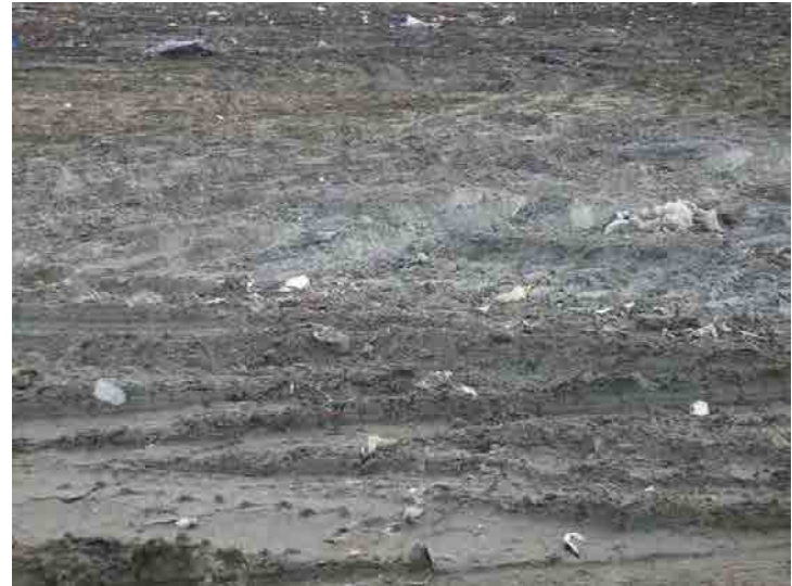
Photo 620: Site Working Area 830-930 am: January 27, 2016
