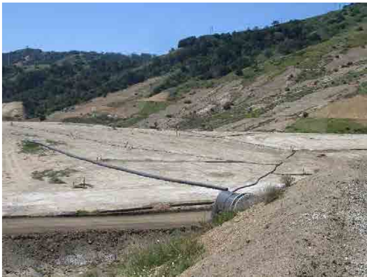
Photo 179: Site County Top Deck: March 23, 2016
