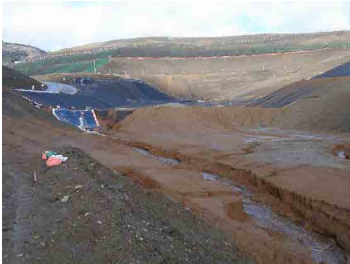
Photo 265: City Cell CC3B Construction: January 7, 2016
