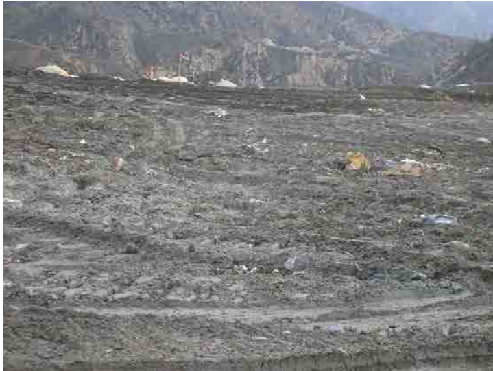
Photo 621: Site Working Area 830-930 am: January 27, 2016
