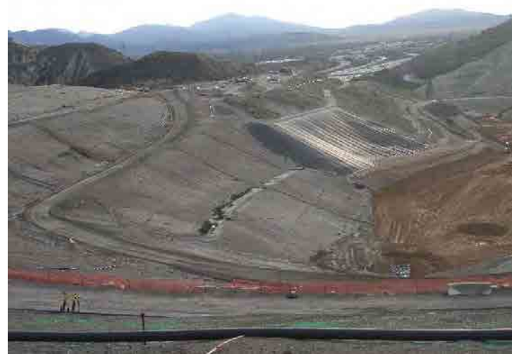
Photo 344: City Slope Erosion Control: January 27, 2016
