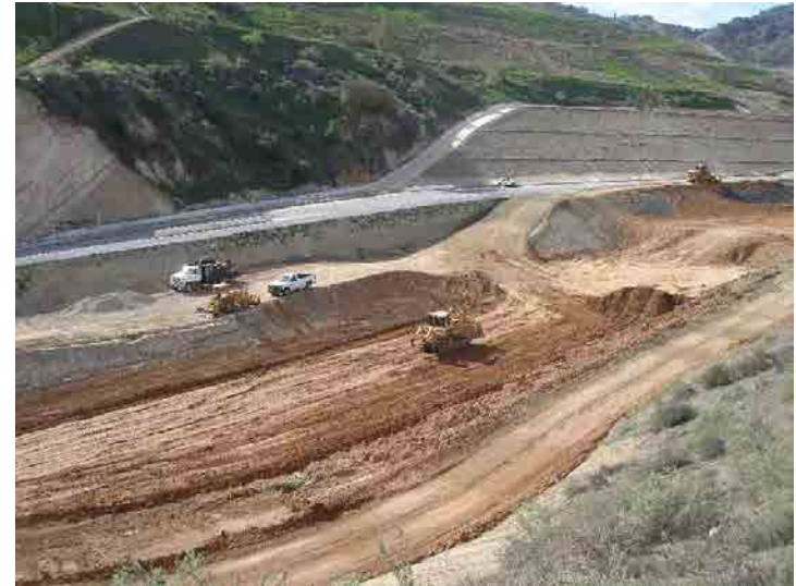
Photo 272: City Cell CC3B Construction: January 27, 2016
