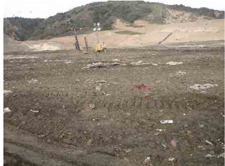
Photo 616: Site Working Area 830-930 am: January 27, 2016
