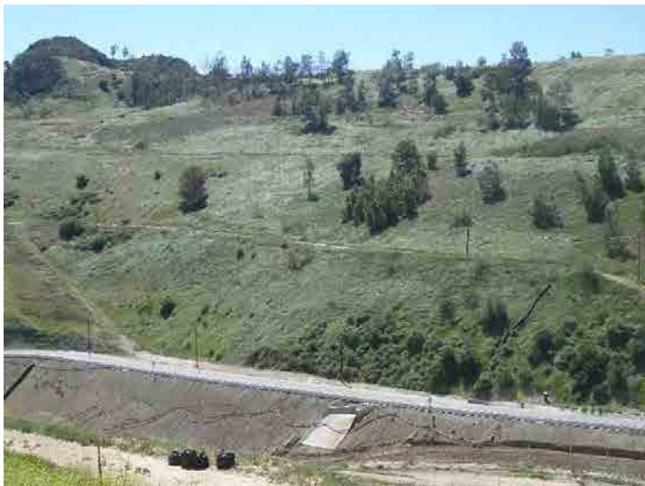
Photo 323: Main Access Road: March 23, 2016
