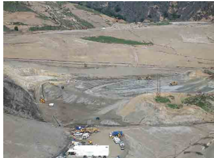
Photo 68: Site Grading South of Basin A: March 9, 2016
