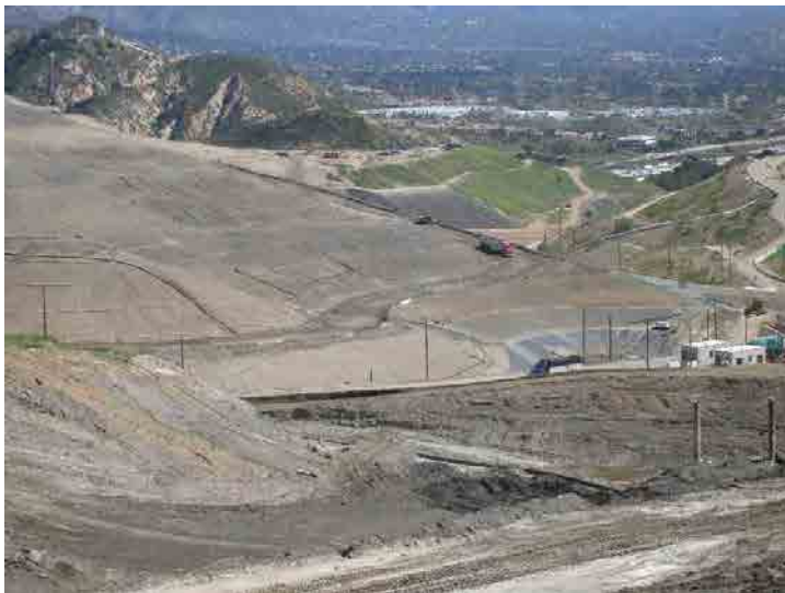
Photo 679: Site Working Area 100 pm: March 23, 2016
