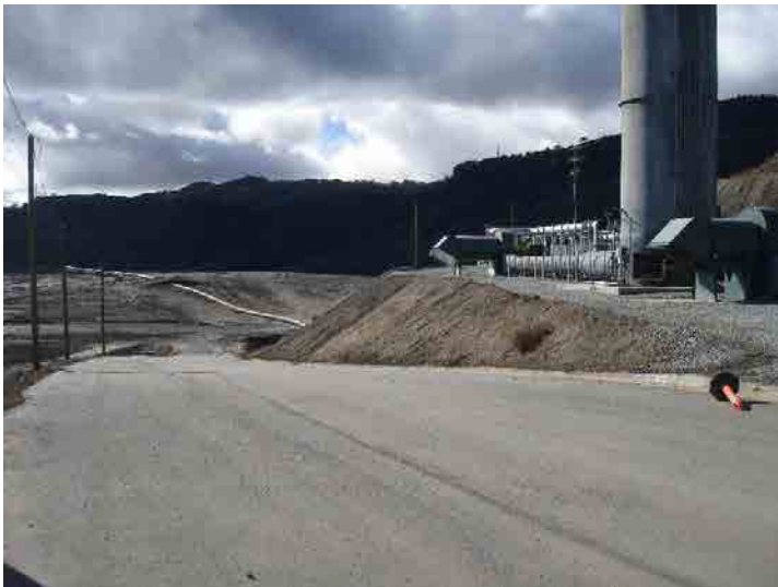
Photo 163: County Top Deck: January 7, 2016
