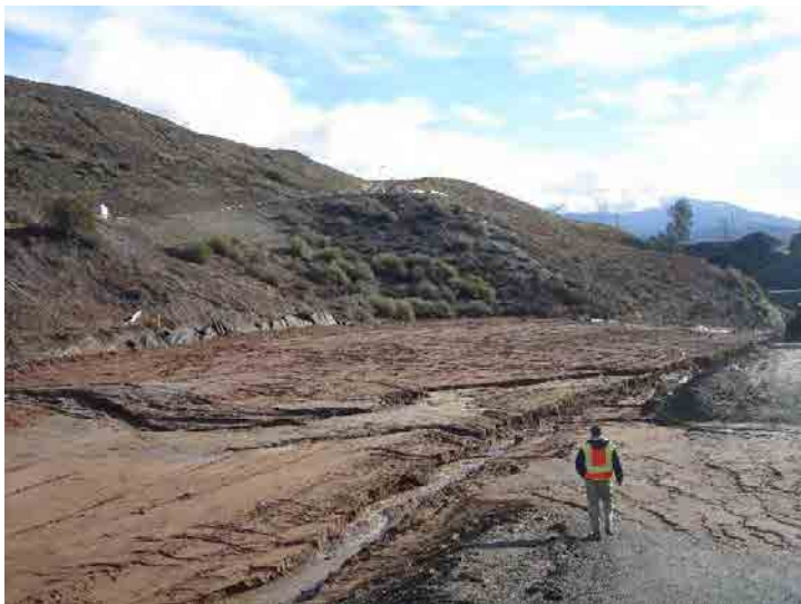
Photo 263: City Cell CC3B Construction: January 7, 2016
