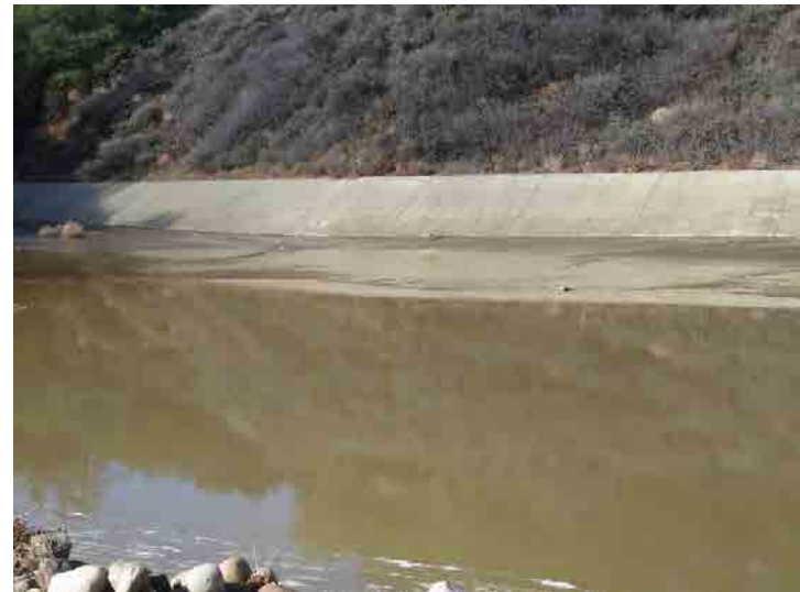
Photo 2: Basin A: January 7, 2016
