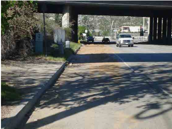
Photo 545: San Fernando Road Near I-5 Overpass: February 24, 2016
