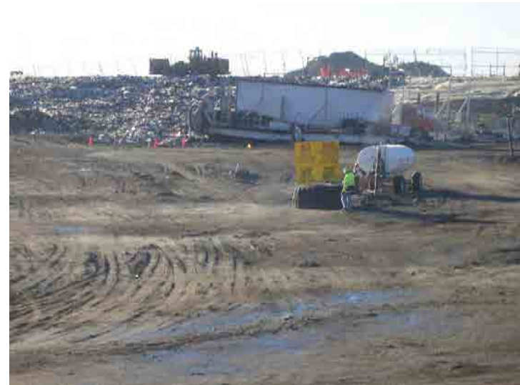
Photo 664: Site Working Area 800am: March 23, 2016
