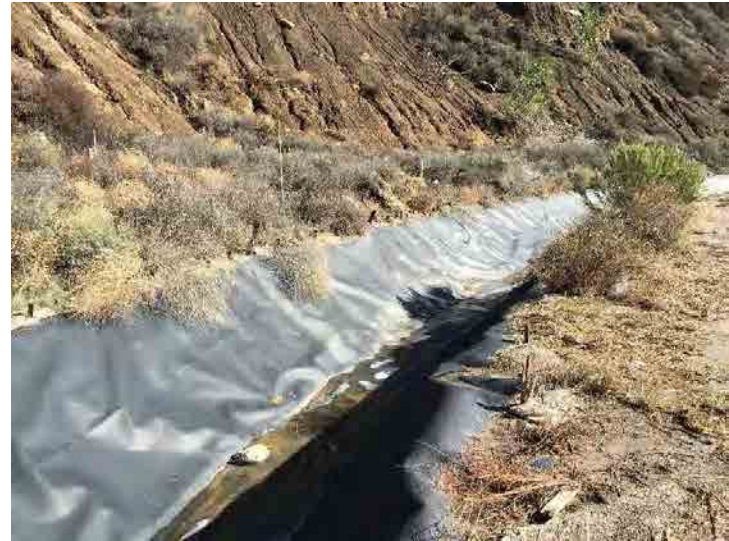
Photo 134: Basin D Outlet Channel: January 7, 2016
