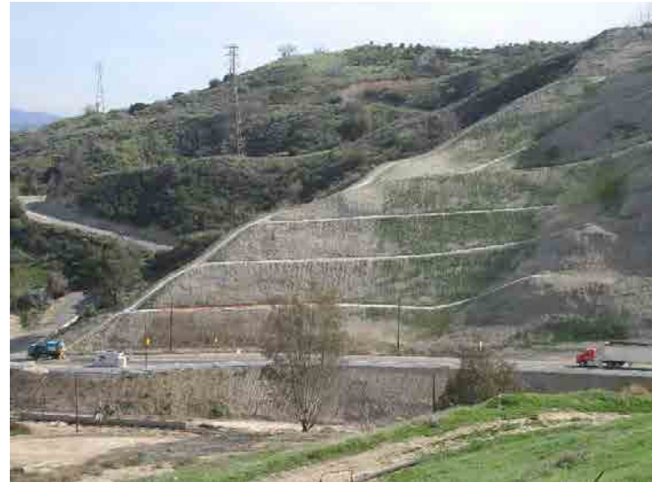
Photo 310: Main Access Road: January 27, 2016
