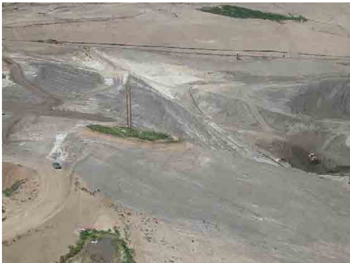
Photo 71: Site Grading South of Basin A: March 23, 2016
