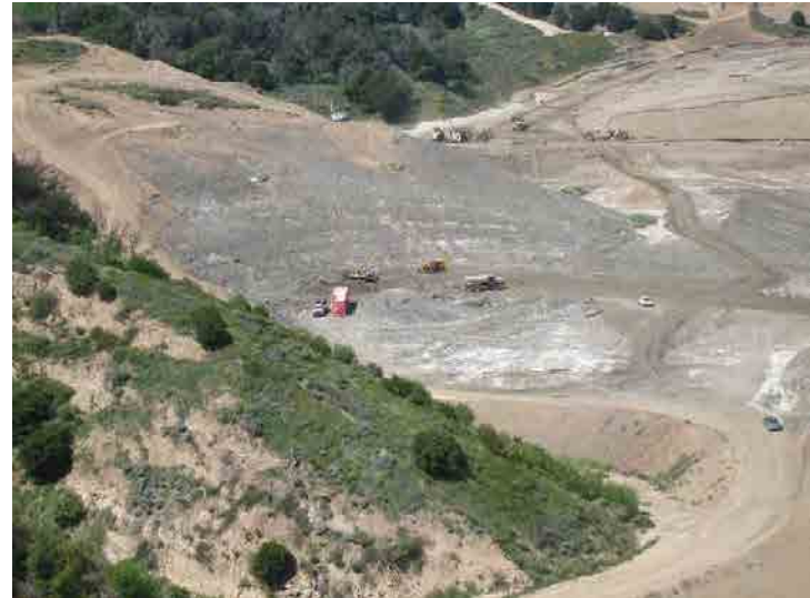
Photo 70: Site Grading South of Basin A: March 23, 2016
