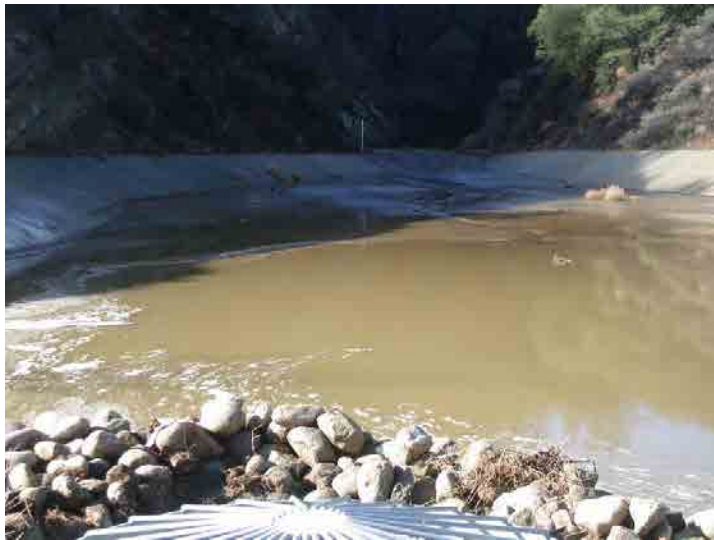
Photo 1: Basin A: January 7, 2016
