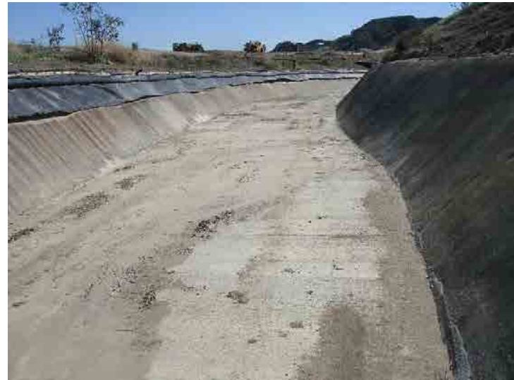
Photo 108: Westside Drainage Channel: February 24, 2016
