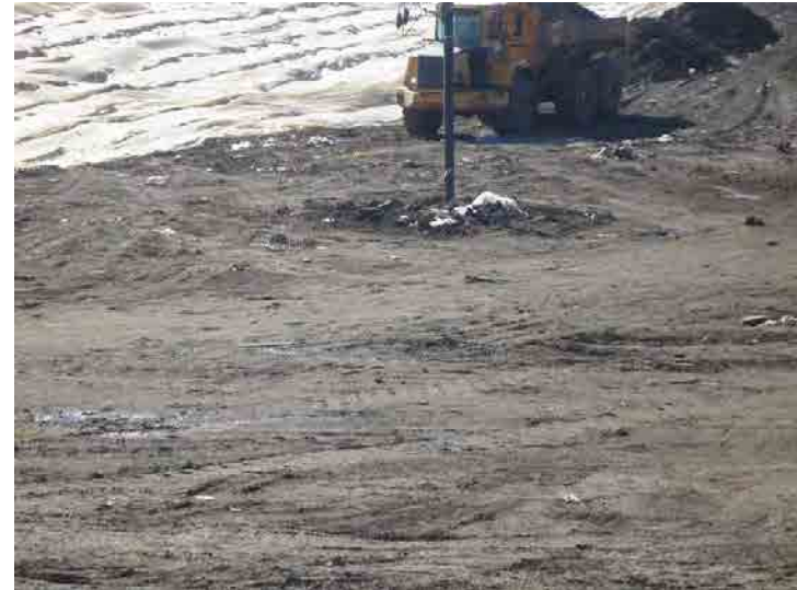
Photo 642: Site Working Area 1100am: February 24, 2016
