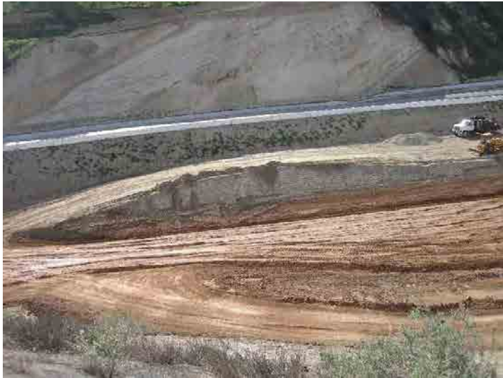
Photo 273: City Cell CC3B Construction: January 27, 2016
