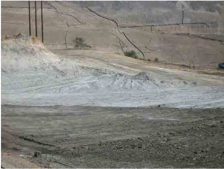
Photo 57: Site Grading South of Basin A: February 24, 2016
