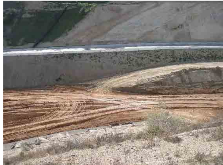
Photo 278: City Cell CC3B Construction: January 27, 2016
