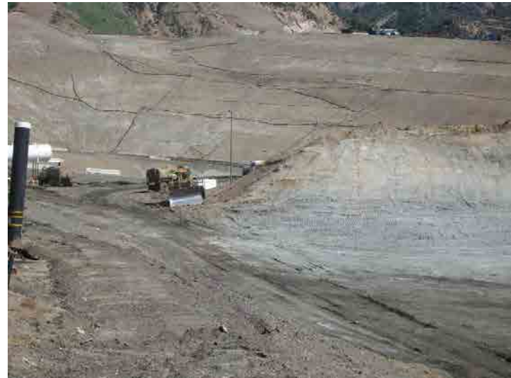
Photo 56: Site Grading South of Basin A: February 24, 2016
