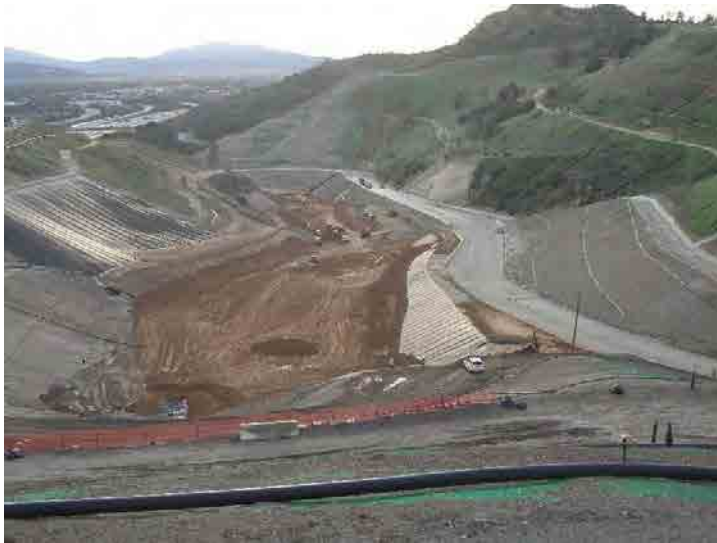
Photo 345: City Slope Erosion Control: January 27, 2016
