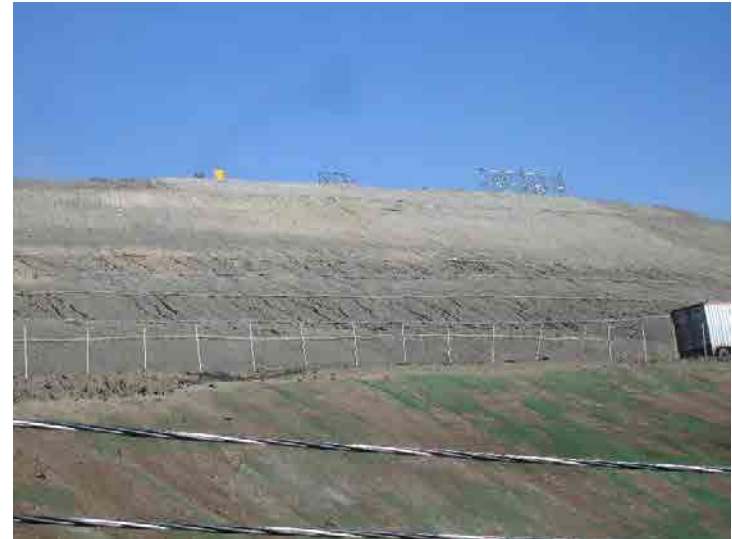
Photo 638: Site Working Area 1100am: February 24, 2016
