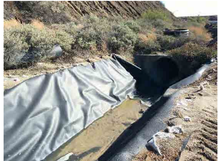
Photo 136: Basin D Outlet Channel: January 7, 2016
