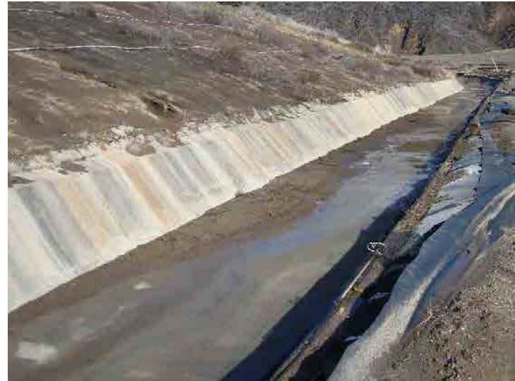
Photo 98: Westside Drainage Channel: January 7, 2016
