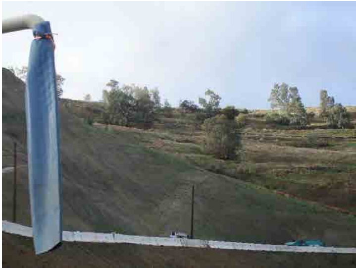
Photo 305: City South Access Road Drainage Control: January 7, 2016
