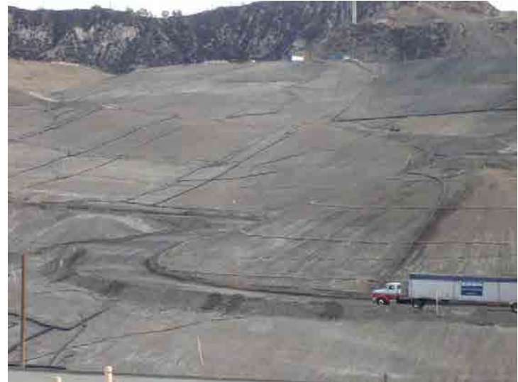
Photo 602: Site Working Area 830-930 am: January 27, 2016
