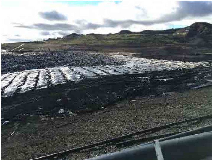
Photo 589: Site Working Area 1000 AM: January 7, 2016
