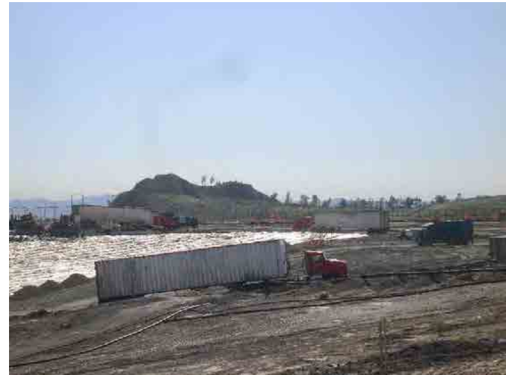
Photo 644: Site Working Area 1200am: February 24, 2016
