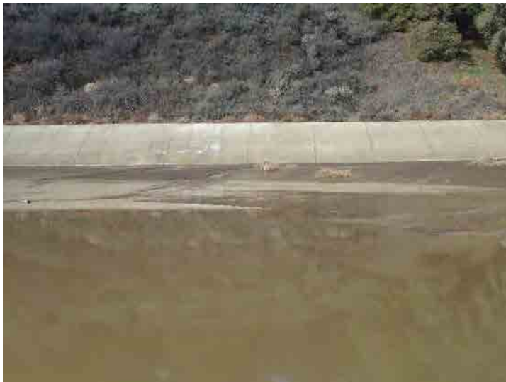
Photo 3: Basin A: January 7, 2016
