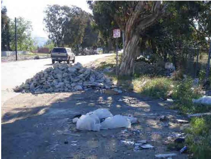
Photo 557: San Fernando Road Near I-5 Overpass: March 23, 2016
