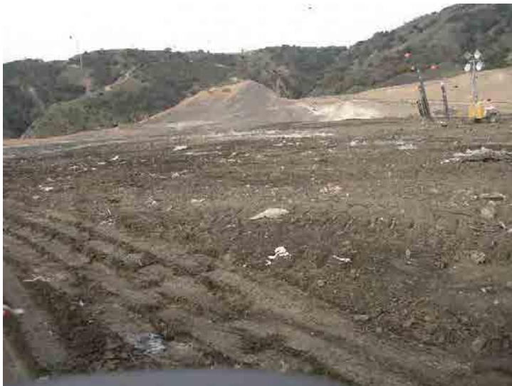
Photo 615: Site Working Area 830-930 am: January 27, 2016
