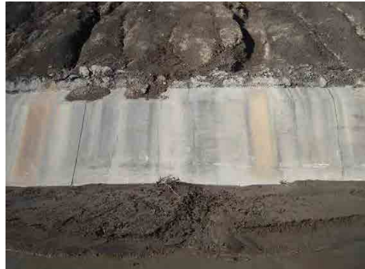
Photo 100: Westside Drainage Channel: January 7, 2016
