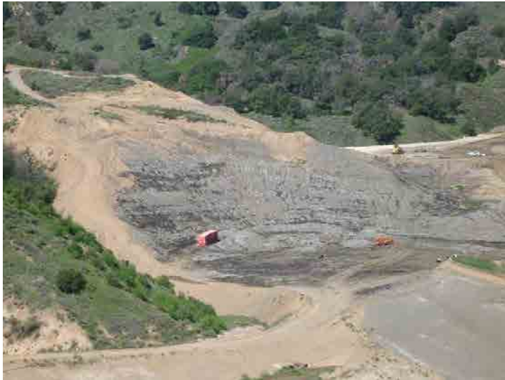
Photo 69: Site Grading South of Basin A: March 9, 2016
