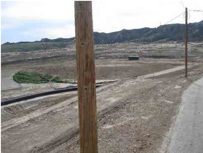
Photo 167: County Top Deck: January 27, 2016
