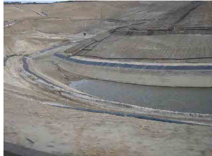
Photo 82: City Lined Drainage Lift Area: January 27, 2016
