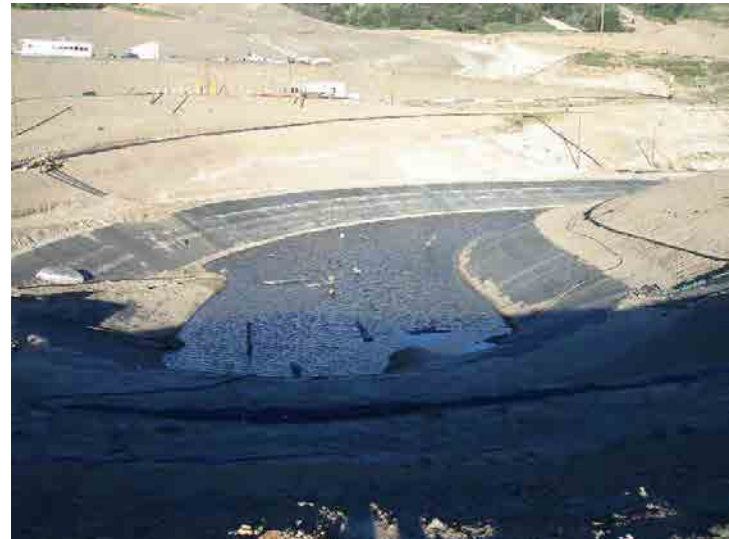
Photo 92: City Lined Drainage Lift Area: March 23, 2016
