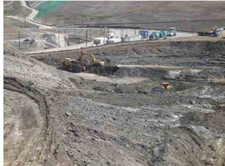
Photo 60: Site Grading South of Basin A: February 24, 2016
