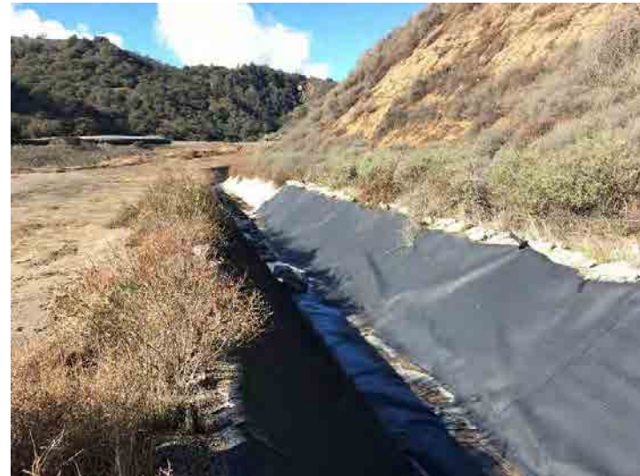
Photo 132: Basin D Outlet Channel: January 7, 2016
