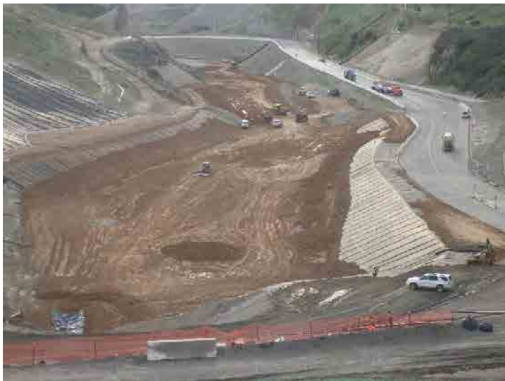
Photo 347: City Slope Erosion Control: January 27, 2016
