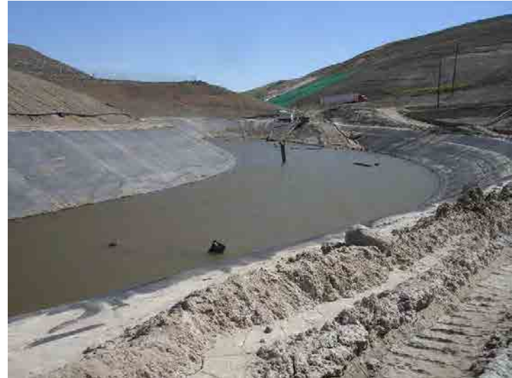
Photo 88: City Lined Drainage Lift Area: February 24, 2016
