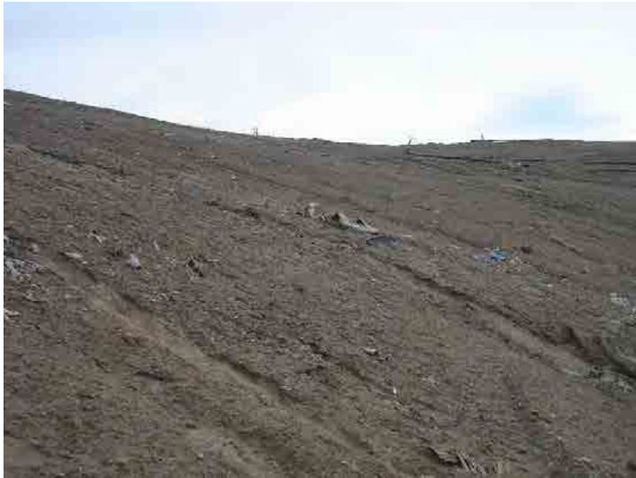
Photo 333: County South Slope Inert Waste Exposed: January 27, 2016
