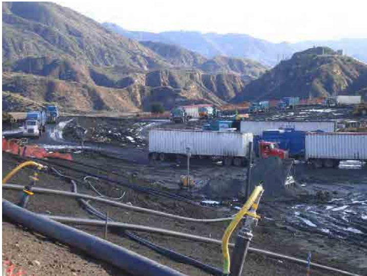
Photo 591: Site Working Area 1100 am: January 7, 2016
