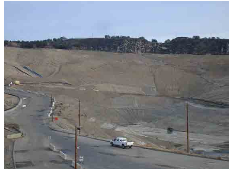
Photo 338: County South Slope Erosion Control: January 27, 2016
