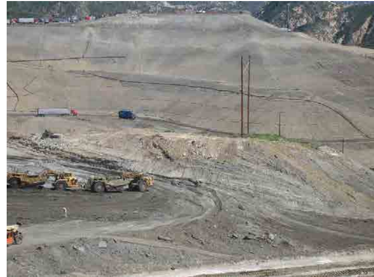
Photo 678: Site Working Area 100 pm: March 23, 2016
