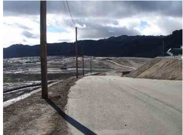
Photo 162: County Top Deck: January 7, 2016
