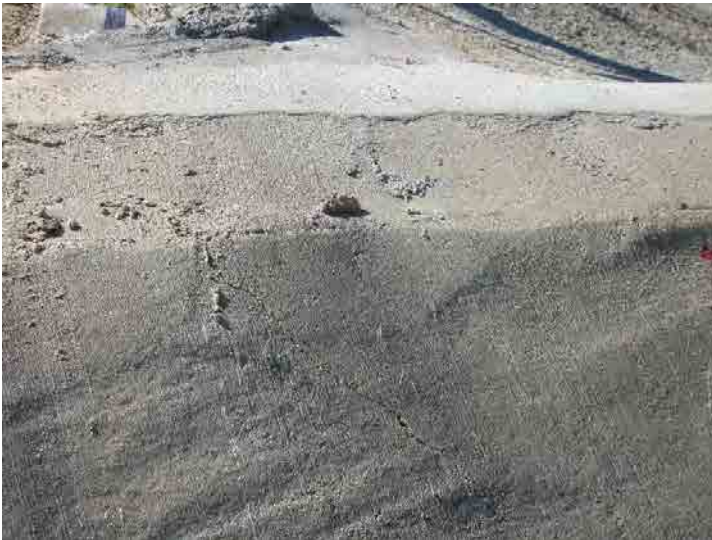
Photo 111: Westside Drainage Channel: February 24, 2016
