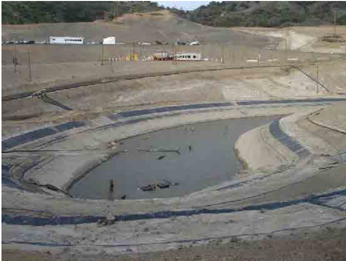
Photo 81: City Lined Drainage Lift Area: January 27, 2016
