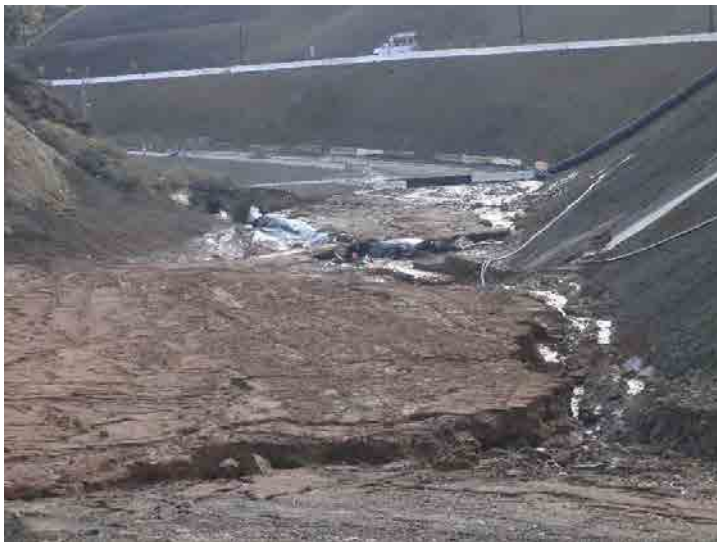
Photo 267: City Cell CC3B Construction: January 7, 2016
