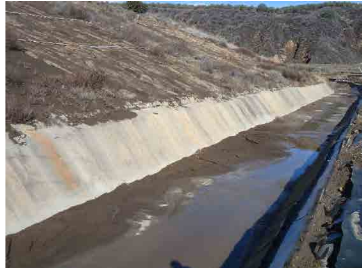
Photo 102: Westside Drainage Channel: January 7, 2016
