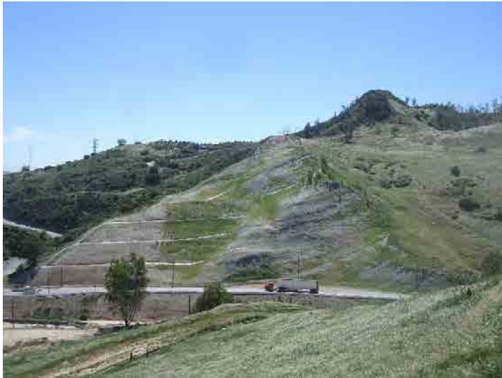
Photo 321: Main Access Road: March 23, 2016
