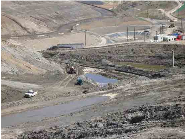
Photo 73: Oil Well Casings to be Abandoned: March 9, 2016
