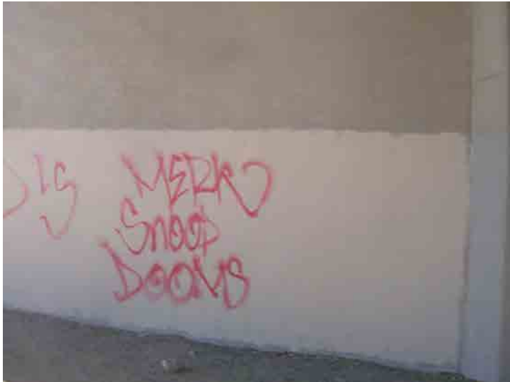
Photo 547: San Fernando Road Near I-5 Overpass: February 24, 2016
