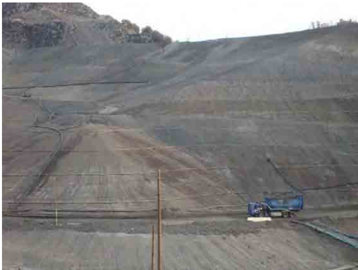
Photo 603: Site Working Area 830-930 am: January 27, 2016
