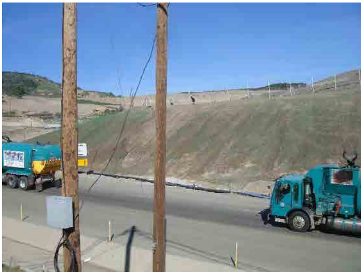
Photo 363: City Slope Erosion Control: February 24, 2016
