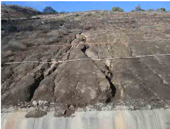
Photo 99: Westside Drainage Channel: January 7, 2016
