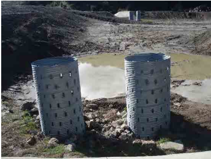
Photo 119: Basin D: January 7, 2016
