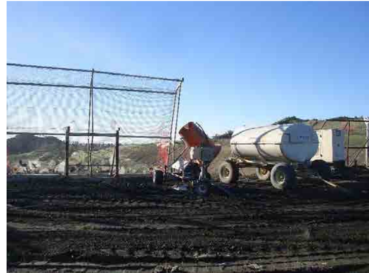
Photo 674: Site Working Area 800am: March 23, 2016
