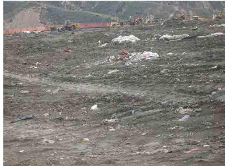
Photo 624: Site Working Area 830-930 am: January 27, 2016
