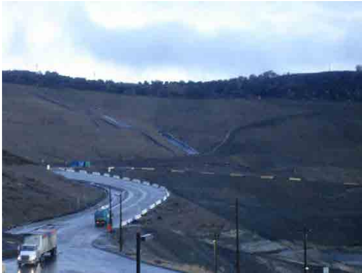
Photo 569: Haul Road to Working Face: January 7, 2016
