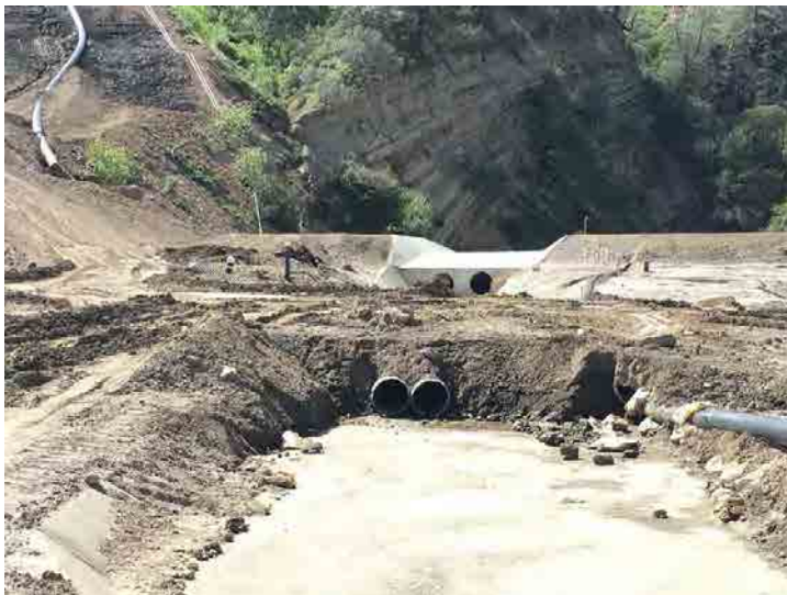
Photo 31: Basin A Outlet: March 9, 2016
