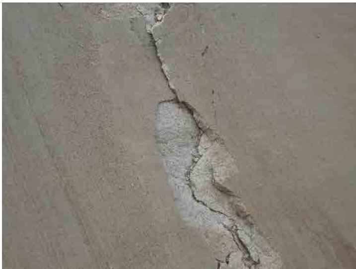
Photo 107: Westside Drainage Channel: January 27, 2016
