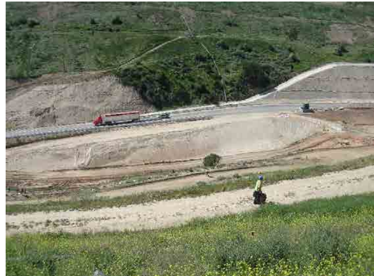
Photo 328: Main Access Road: March 23, 2016
