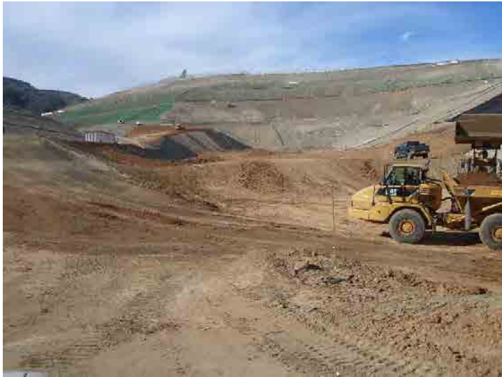
Photo 281: City Cell CC3B Construction: January 27, 2016
