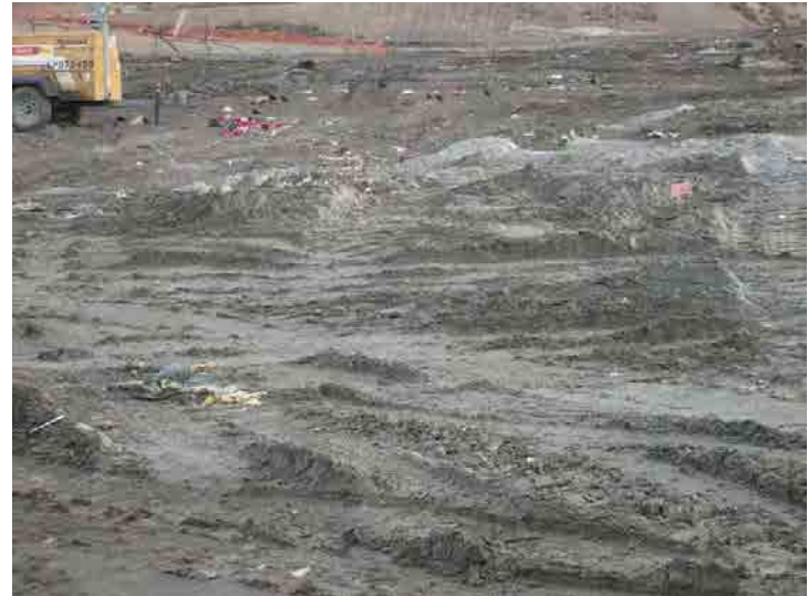
Photo 618: Site Working Area 830-930 am: January 27, 2016
