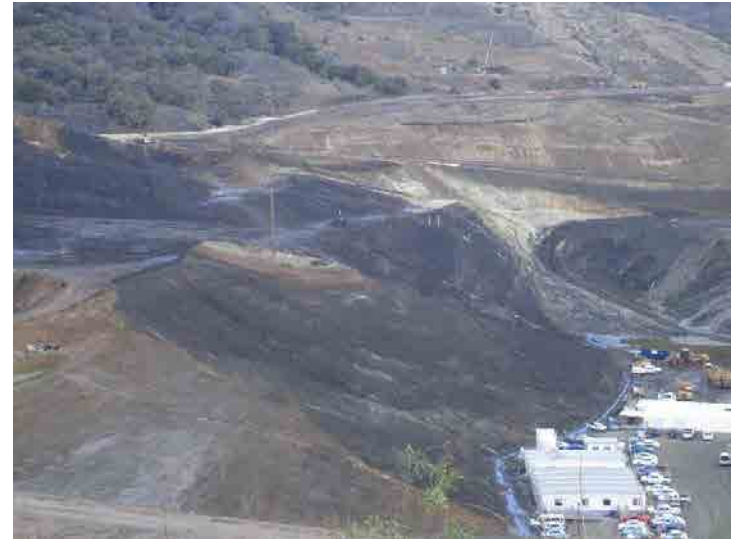
Photo 46: Site Grading South of Basin A: January 7, 2016
