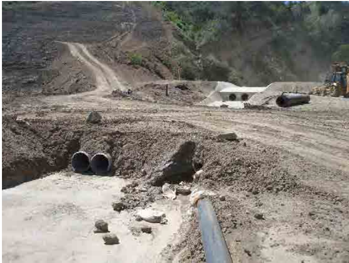
Photo 41: Basin A Outlet: March 23, 2016
