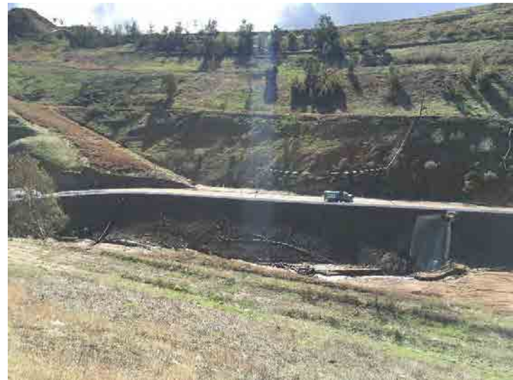
Photo 308: City South Access Road Drainage Control: January 7, 2016
