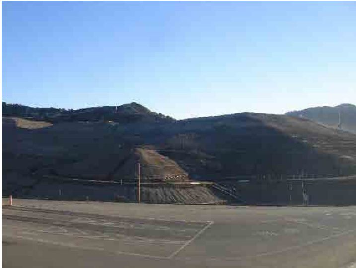
Photo 657: Site Working Area 800am: March 23, 2016
