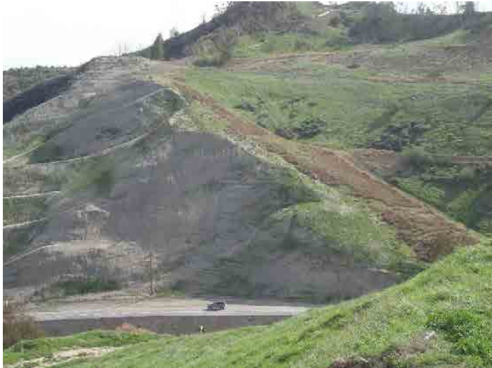
Photo 311: Main Access Road: January 27, 2016
