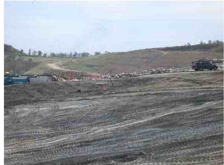
Photo 634: Site Working Area 200 pm: January 27, 2016
