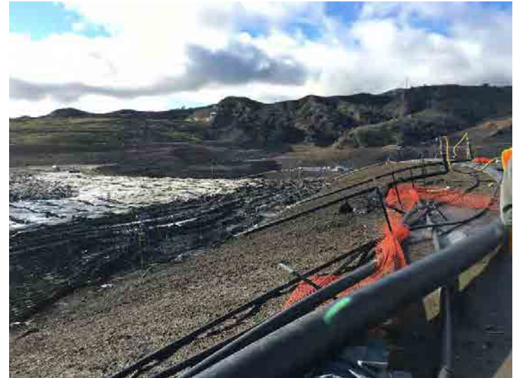
Photo 590: Site Working Area 1000 AM: January 7, 2016
