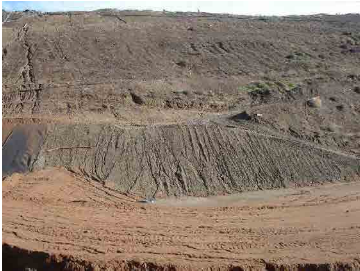
Photo 261: City Cell CC3B Construction: January 7, 2016
