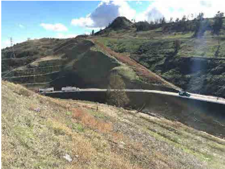
Photo 307: City South Access Road Drainage Control: January 7, 2016
