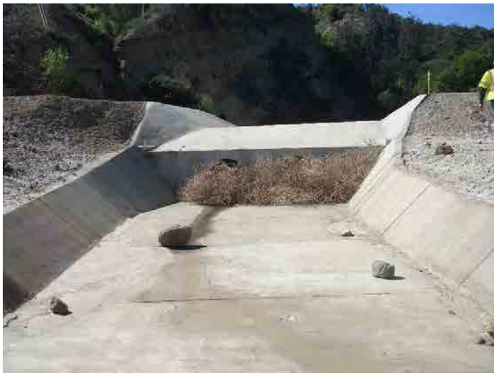
Photo 23: Basin A Outlet: February 24, 2016
