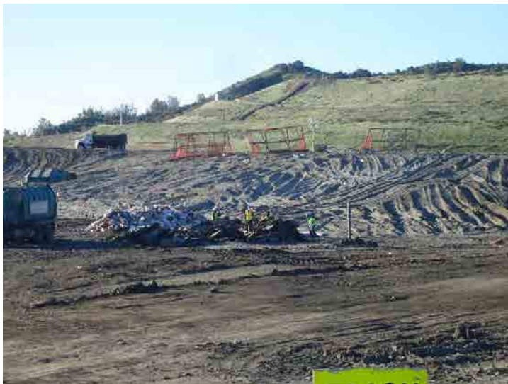
Photo 663: Site Working Area 800am: March 23, 2016
