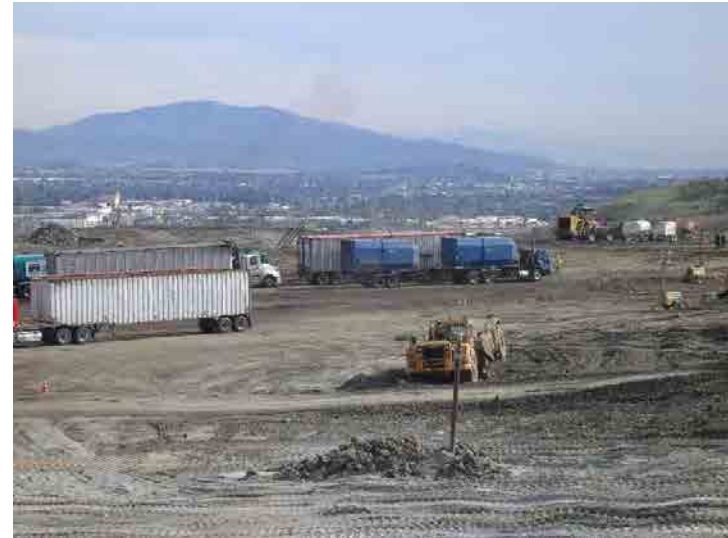
Photo 632: Site Working Area 200 pm: January 27, 2016
