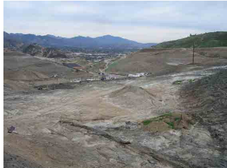
Photo 50: Site Grading South of Basin A: January 27, 2016
