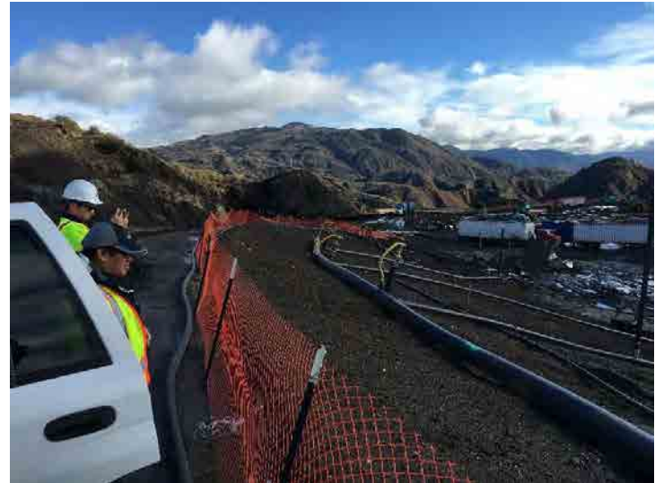
Photo 586: Site Working Area 1000 AM: January 7, 2016
