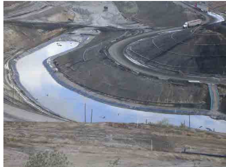
Photo 76: City Lined Drainage Lift Area: January 7, 2016
