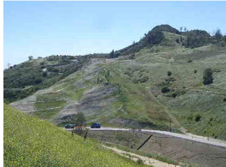
Photo 322: Main Access Road: March 23, 2016
