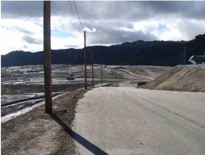
Photo 161: County Top Deck: January 7, 2016
