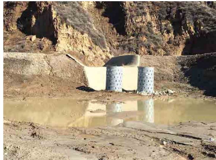
Photo 120: Basin D: January 7, 2016
