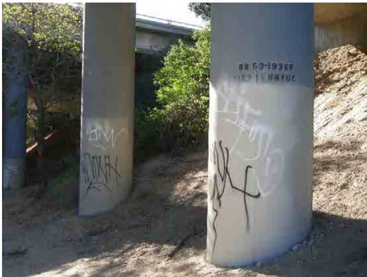
Photo 563: San Fernando Road Near I-5 Overpass: March 23, 2016
