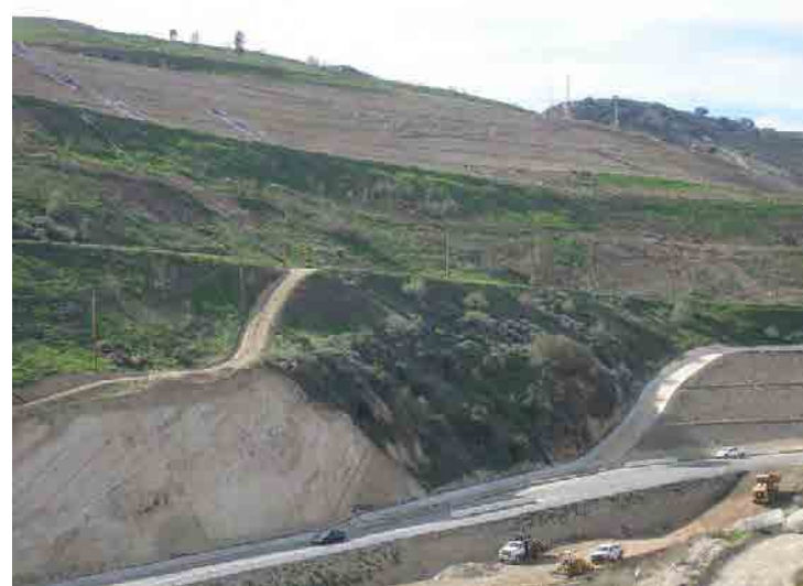
Photo 320: Main Access Road: January 27, 2016
