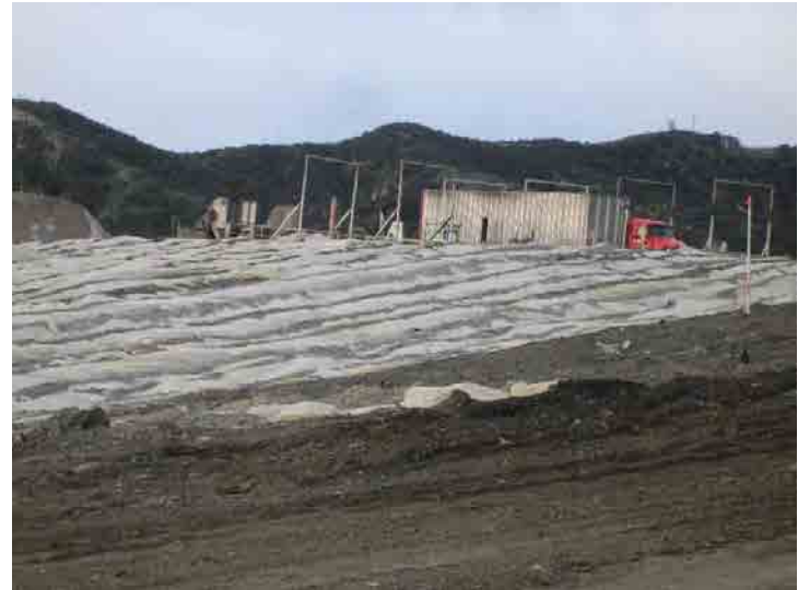
Photo 612: Site Working Area 830-930 am: January 27, 2016
