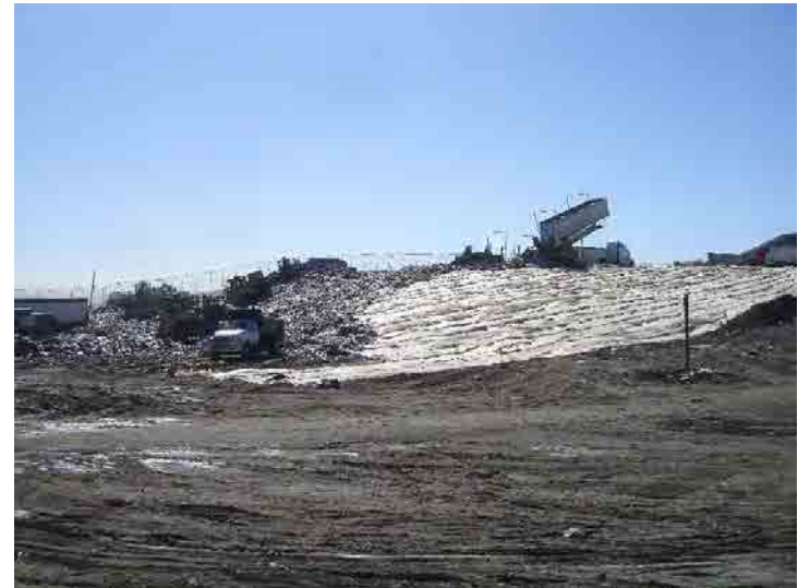
Photo 640: Site Working Area 1100am: February 24, 2016
