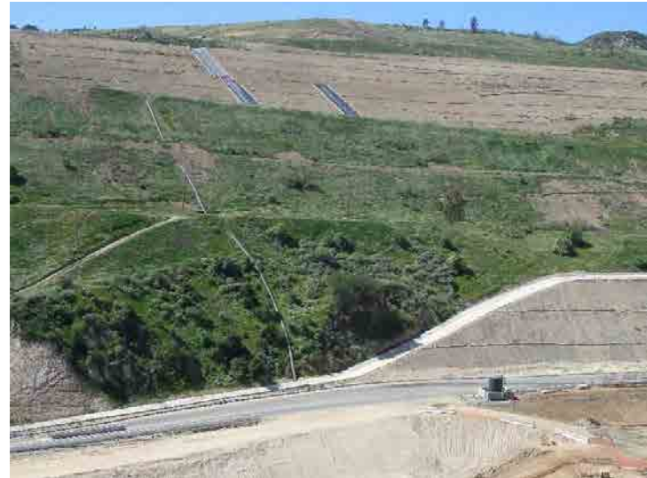
Photo 326: Main Access Road: March 23, 2016
