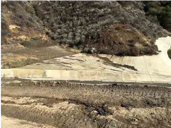
Photo 181: Inlet to Basin B: January 7, 2016
