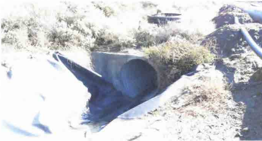
Photo 10: Geomembrane liner at entry to culvert near Flare 9-10 access road
