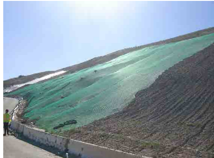
Photo 364: City Slope Erosion Control: February 24, 2016
