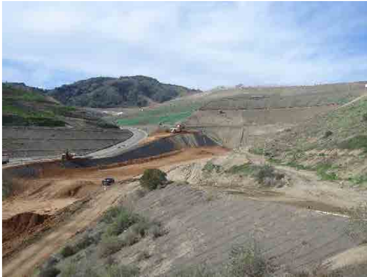
Photo 269: City Cell CC3B Construction: January 27, 2016
