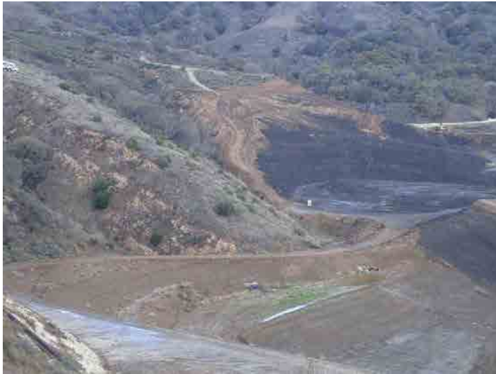
Photo 45: Site Grading South of Basin A: January 7, 2016
