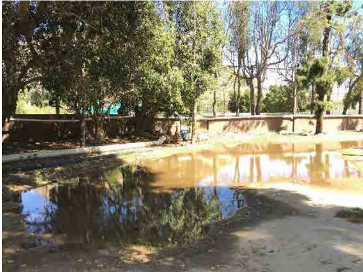
Photo 509: Sewer Deep Well Pump Area: March 9, 2016
