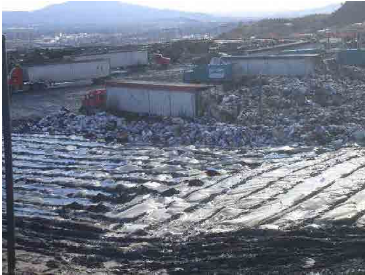
Photo 593: Site Working Area 1100 am: January 7, 2016
