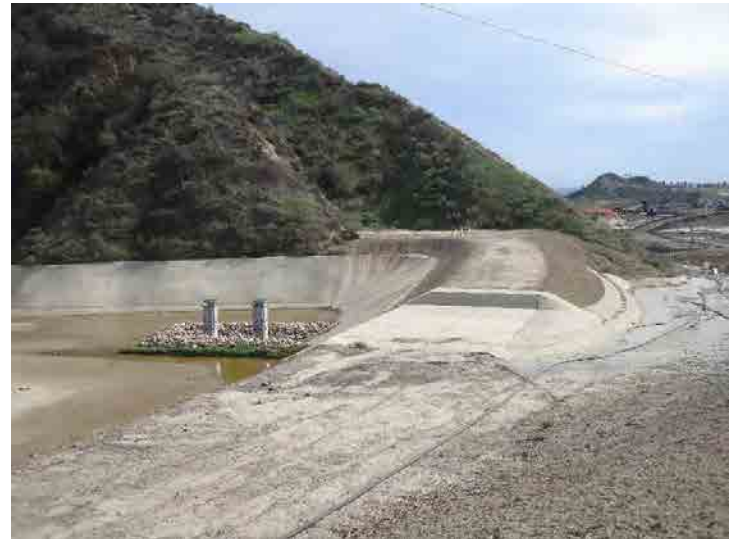
Photo 192: Basin B: January 27, 2016
