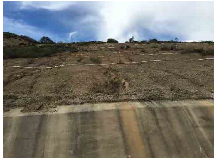
Photo 104: Westside Drainage Channel: January 27, 2016
