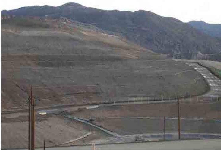
Photo 341: City Slope Erosion Control: January 27, 2016
