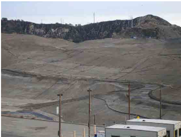
Photo 339: City Slope Erosion Control: January 27, 2016
