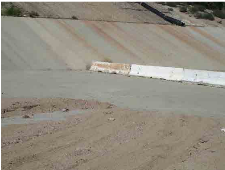
Photo 239: Terminal Basin: February 24, 2016
