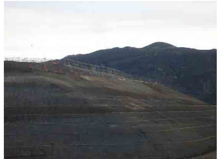
Photo 608: Site Working Area 830-930 am: January 27, 2016
