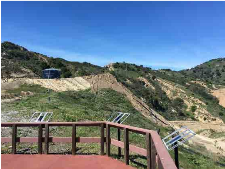
Photo 493: New Facility Water Tank: March 9, 2016
