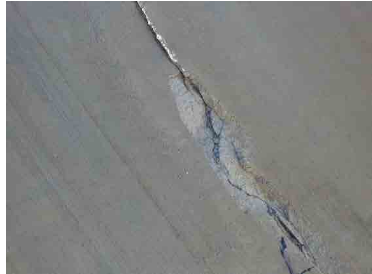
Photo 112: Westside Drainage Channel: February 24, 2016
