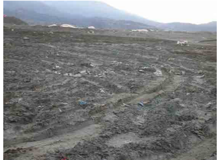
Photo 622: Site Working Area 830-930 am: January 27, 2016
