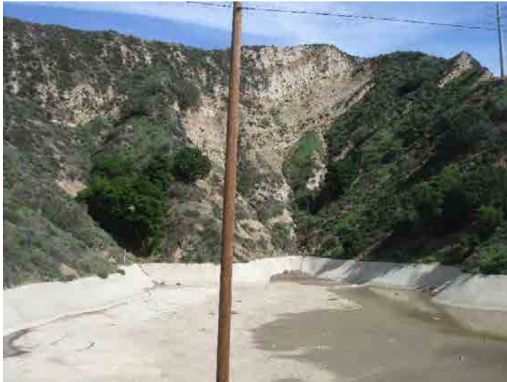
Photo 197: Basin B: March 9, 2016
