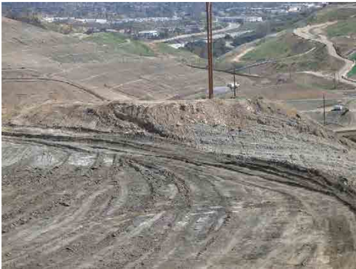
Photo 59: Site Grading South of Basin A: February 24, 2016
