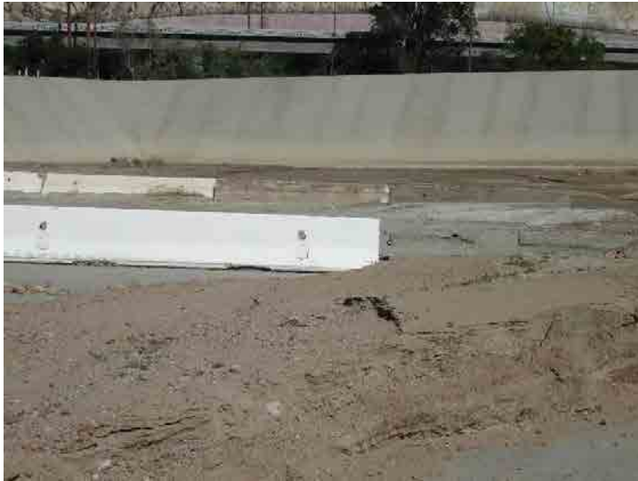
Photo 241: Terminal Basin: February 24, 2016
