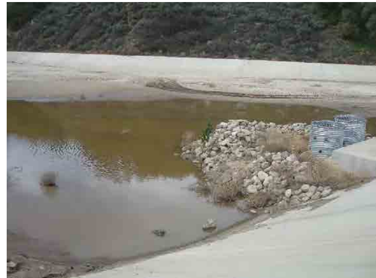
Photo 12: Basin A: January 27, 2015
