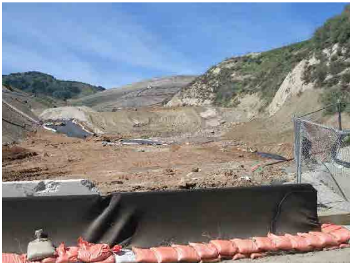
Photo 251: Drainage into Terminal Basin: March 9, 2016
