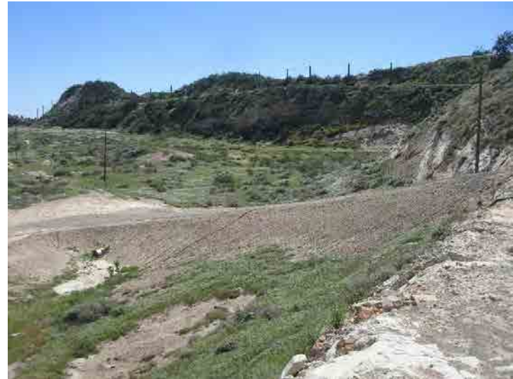
Photo 422: City Mitigation Deck A: March 23, 2016
