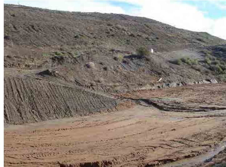
Photo 262: City Cell CC3B Construction: January 7, 2016
