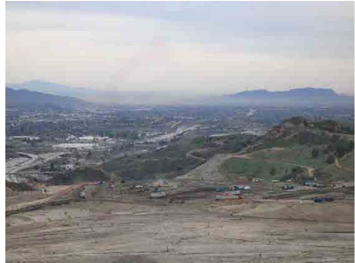
Photo 628: Site Working Area 12 noon: January 27, 2016
