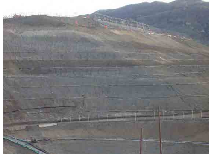
Photo 604: Site Working Area 830-930 am: January 27, 2016
