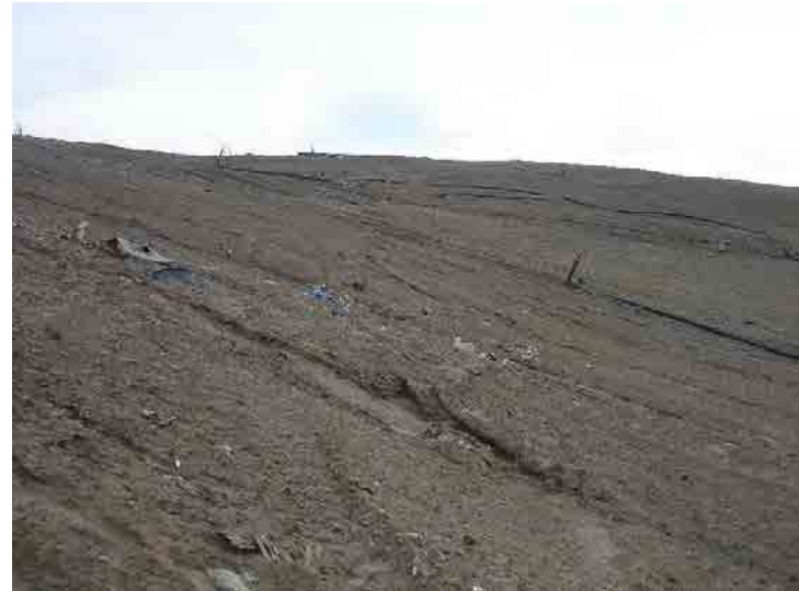
Photo 334: County South Slope Inert Waste Exposed: January 27, 2016
