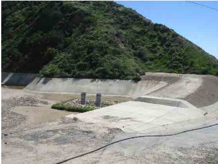
Photo 205: Basin B: March 23, 2016
