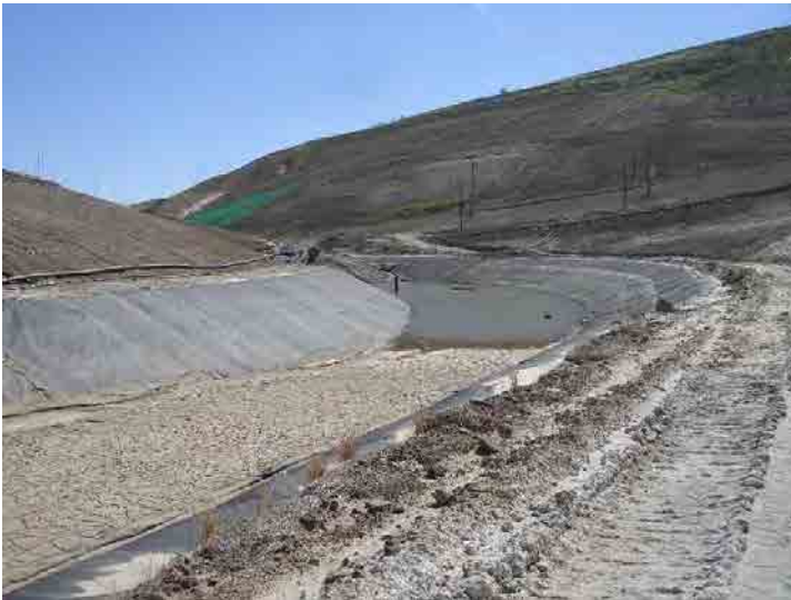
Photo 87: City Lined Drainage Lift Area: February 24, 2016
