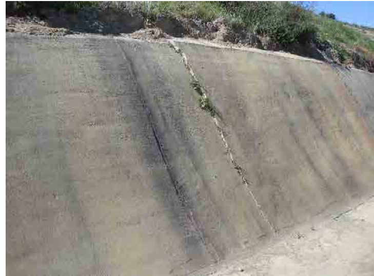
Photo 114: Westside Drainage Channel: February 24, 2016
