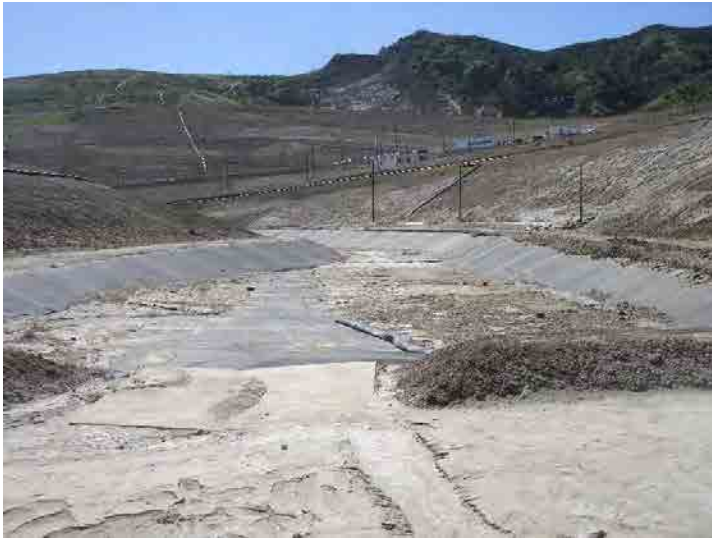
Photo 85: City Lined Drainage Lift Area: February 24, 2016
