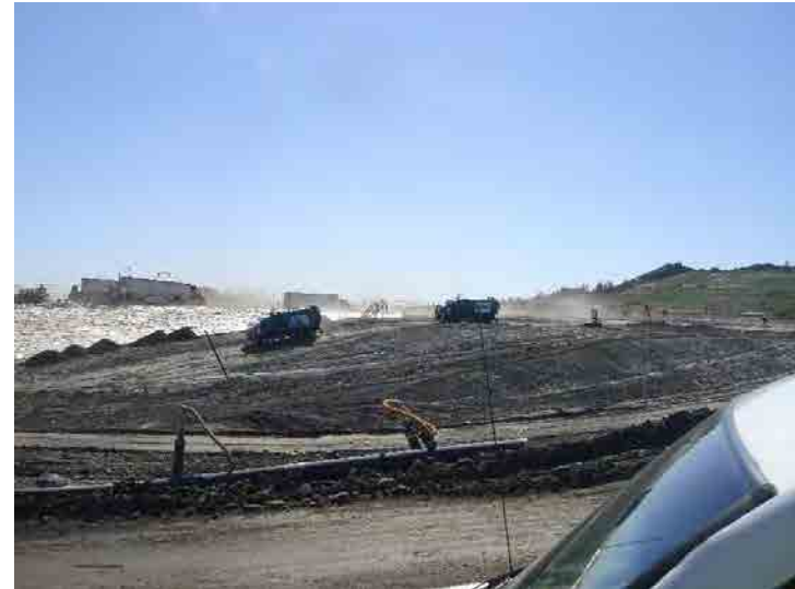
Photo 646: Site Working Area 1200am: February 24, 2016
