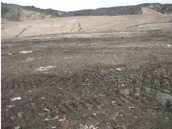
Photo 617: Site Working Area 830-930 am: January 27, 2016
