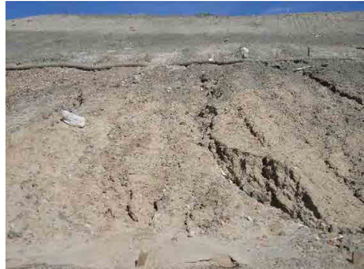
Photo 350: County South Facing Slope, Inert Waste Exposed: February 24, 2016
