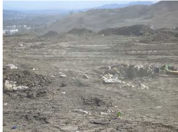
Photo 542: Site 12-2 pm: November 16, 2015
