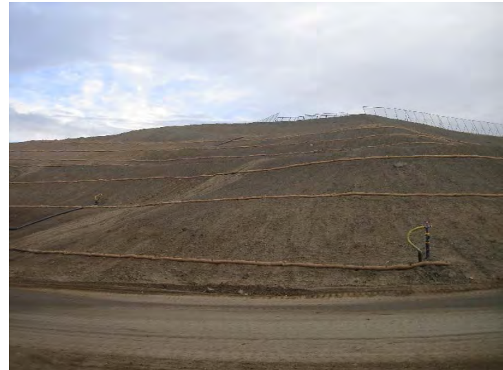
Photo 264: City Slope Erosion Control: October 28, 2015
