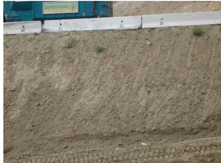
Photo 228: Main Access Road Slope: October 28, 2015
