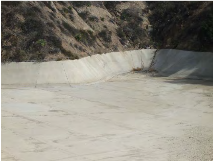
Photo 133: Basin B: October 28, 2015
