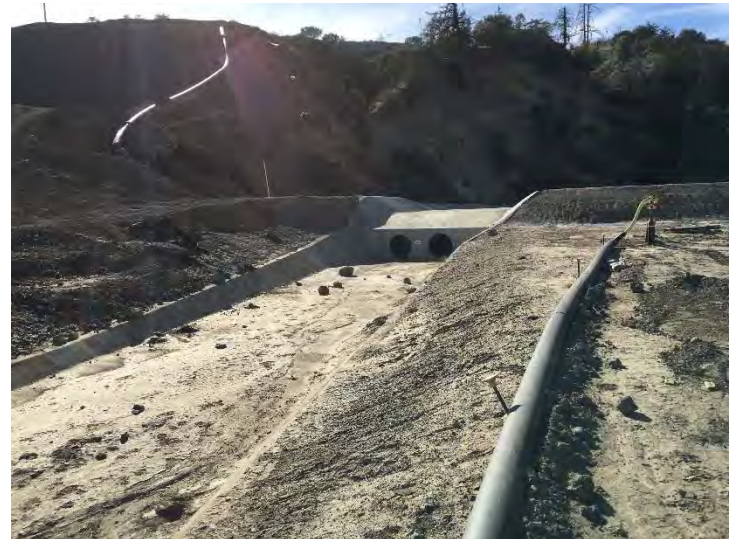
Photo 28: Basin A Drainage Channel: December 9, 2015
