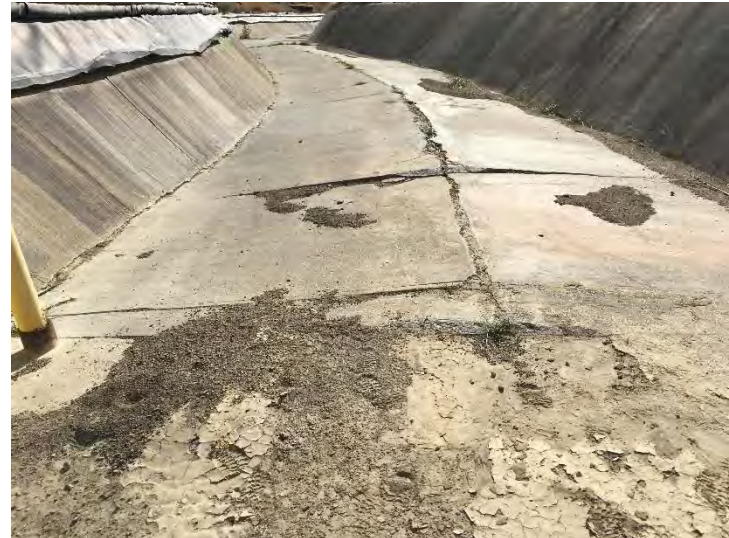
Photo 52: Westside Drainage Channel: December 9, 2015
