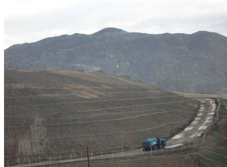
Photo 414: Site Working Area: October 28, 2015
