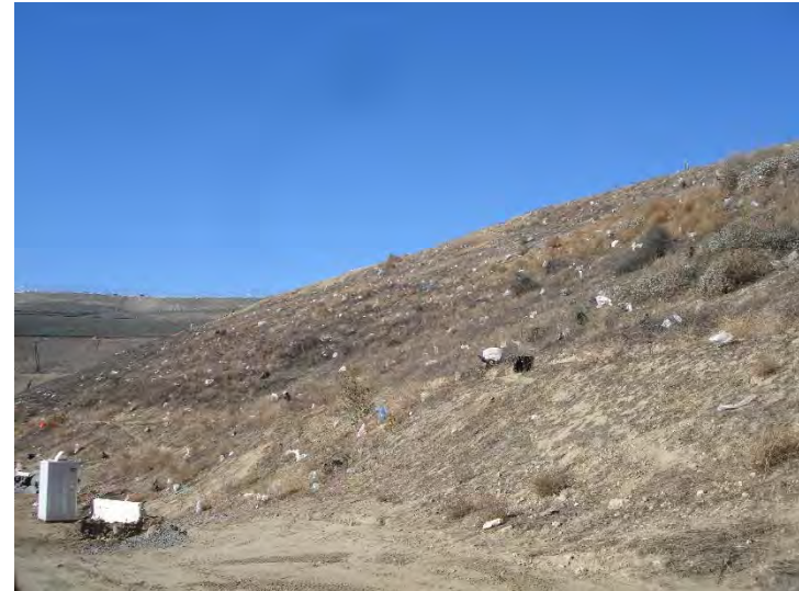
Photo 550: Site 12-2 pm: November 16, 2015
