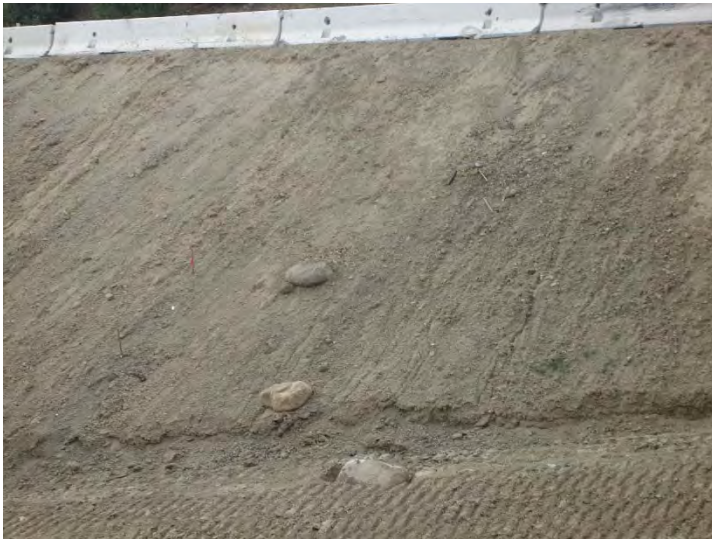
Photo 227: Main Access Road Slope: October 28, 2015
