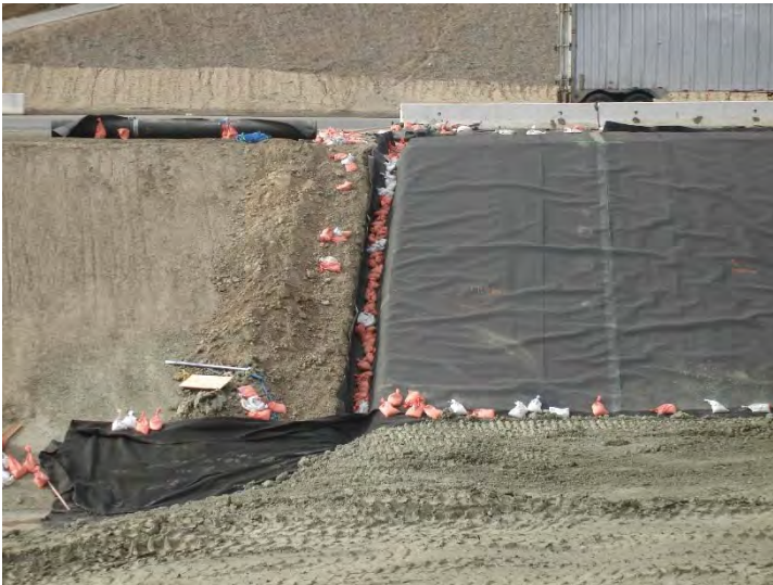
Photo 215: City Cell CC3B Construction: October 28, 2015
