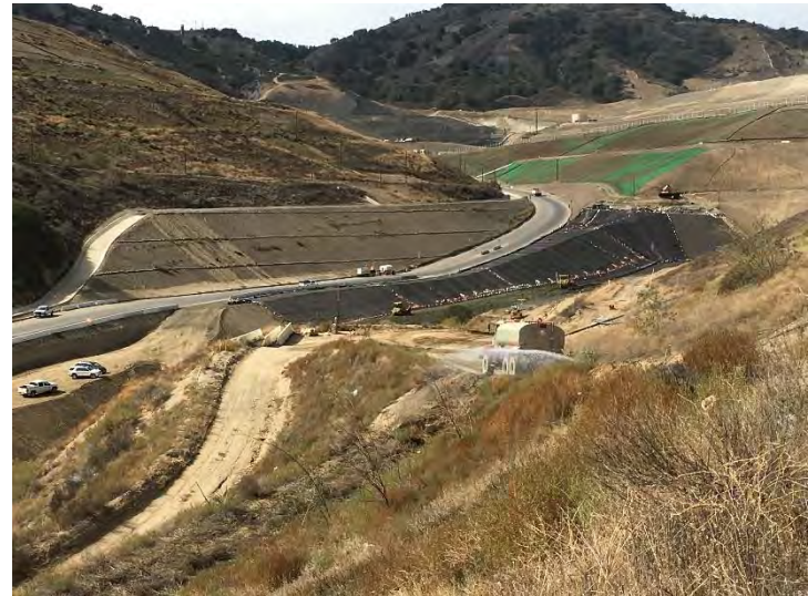
Photo 208: City Cell CC3B Construction: October 28, 2015
