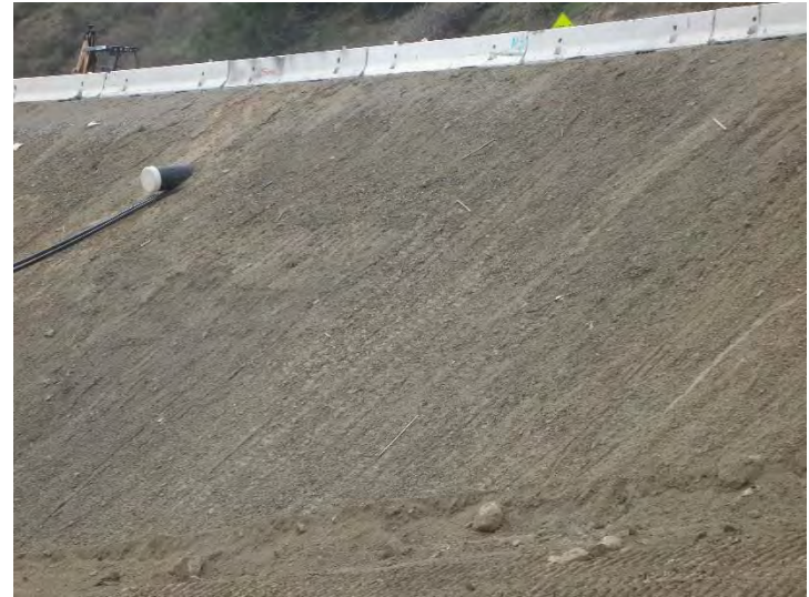
Photo 226: Main Access Road Slope: October 28, 2015
