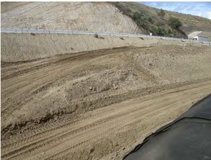
Photo 199: City Cell CC3B Construction: October 14 2015
