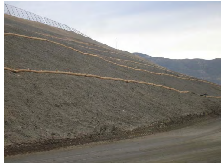
Photo 262: City Slope Erosion Control: October 28, 2015
