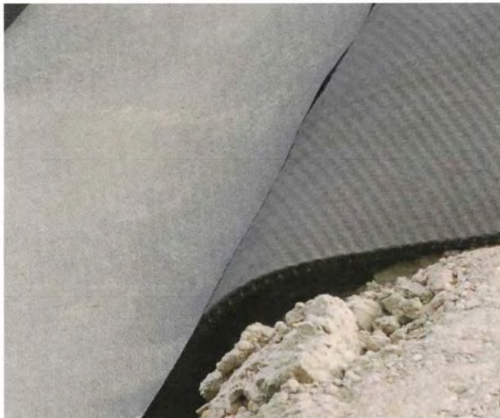
Photo 2: Geocomposite gas collection layer under liner
