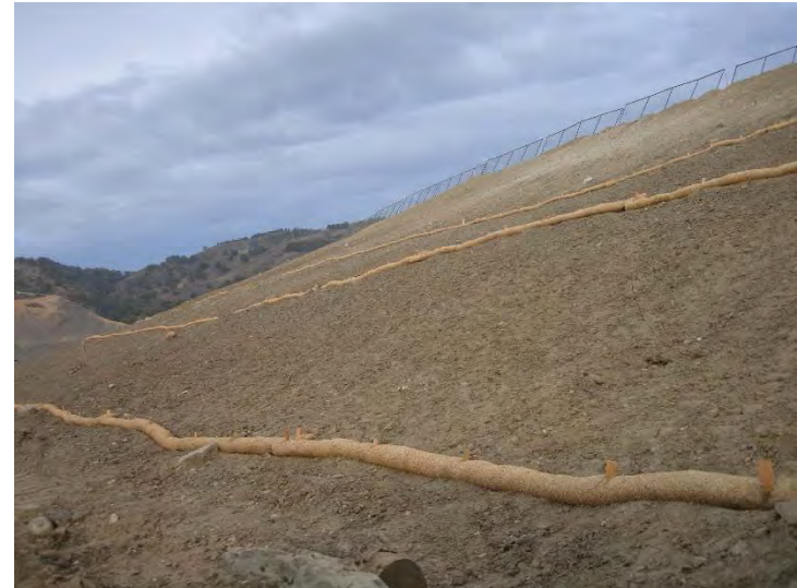
Photo 254: City Slope Erosion Control: October 28, 2015
