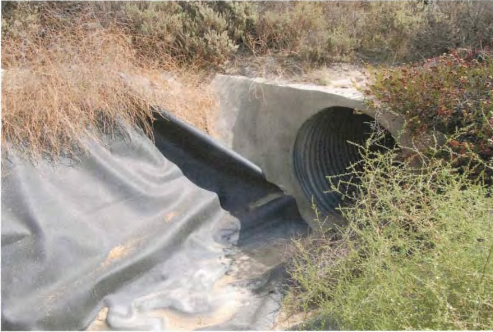
Photo 5: Geomembrane liner at entry to culvert near Flare 9-10 access road
