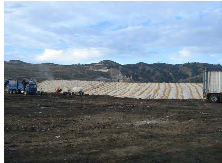
Photo 392: Site Working Area 7-8 am: October 14, 2015
