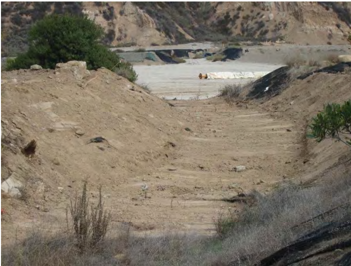
Photo 79: Native Hillside Drainage into Basin D: October 28, 2015
