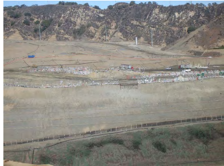
Photo 532: Site 11am-12pm: November 16, 2015
