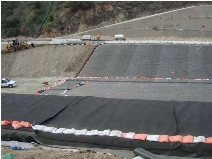
Photo 191: City Cell CC3B Construction: October 14 2015
