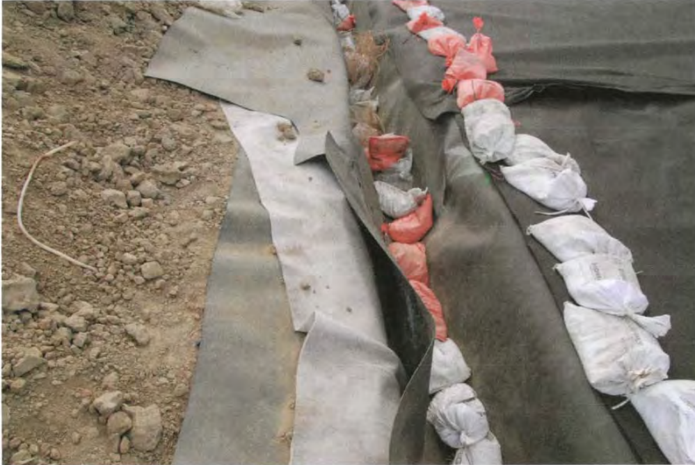
Photo 1: Liner system on slope
