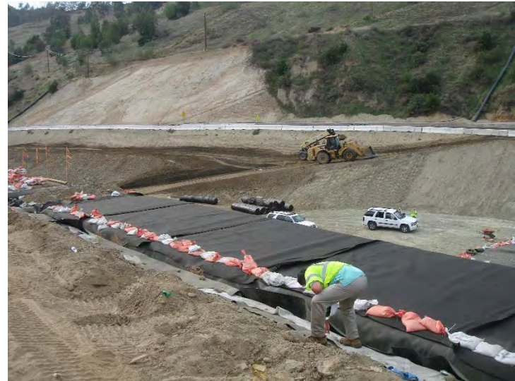
Photo 192: City Cell CC3B Construction: October 14 2015
