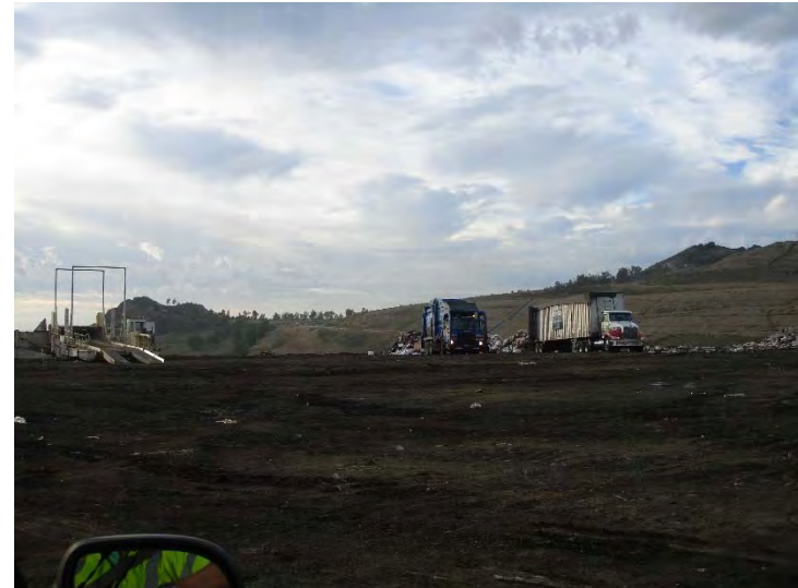
Photo 390: Site Working Area 7-8 am: October 14, 2015
