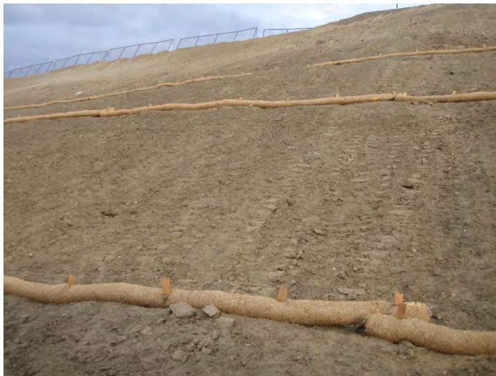
Photo 255: City Slope Erosion Control: October 28, 2015
