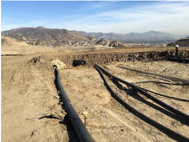
Photo 29: Basin A Drainage Channel: December 9, 2015
