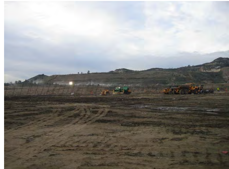
Photo 416: Site Working Area: October 28, 2015
