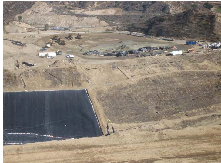
Photo 536: Site 11am-12pm: November 16, 2015
