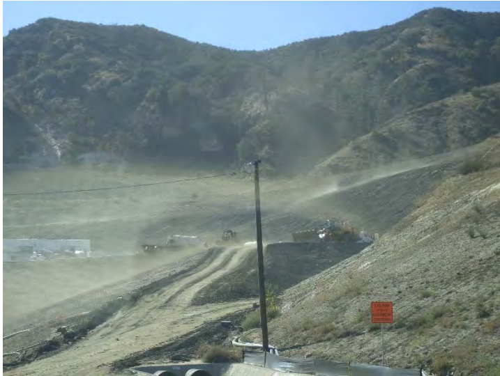
Photo 525: Site 11am-12pm: November 16, 2015
