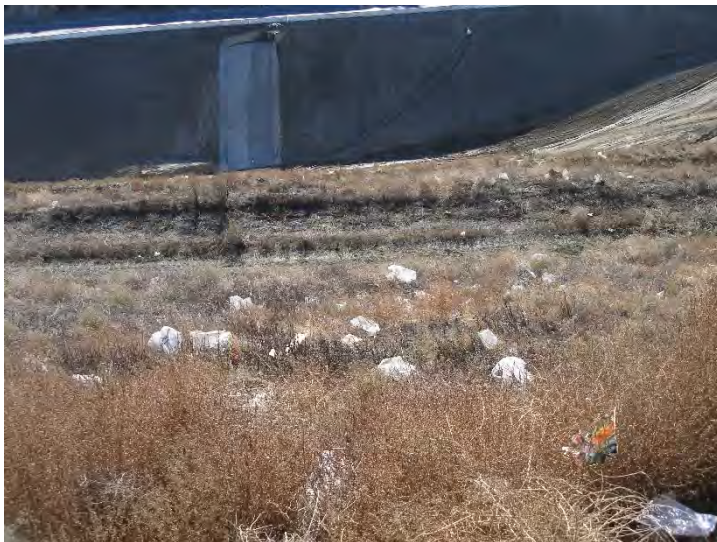
Photo 547: Site 12-2 pm: November 16, 2015
