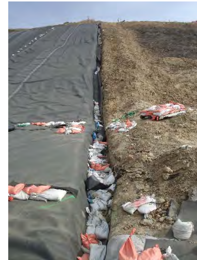
Photo 216: City Cell CC3B Construction: October 28, 2015
