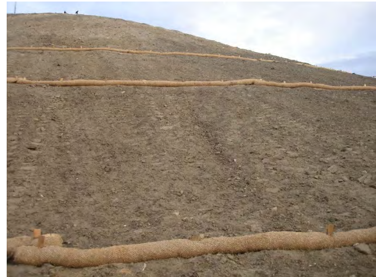
Photo 256: City Slope Erosion Control: October 28, 2015
