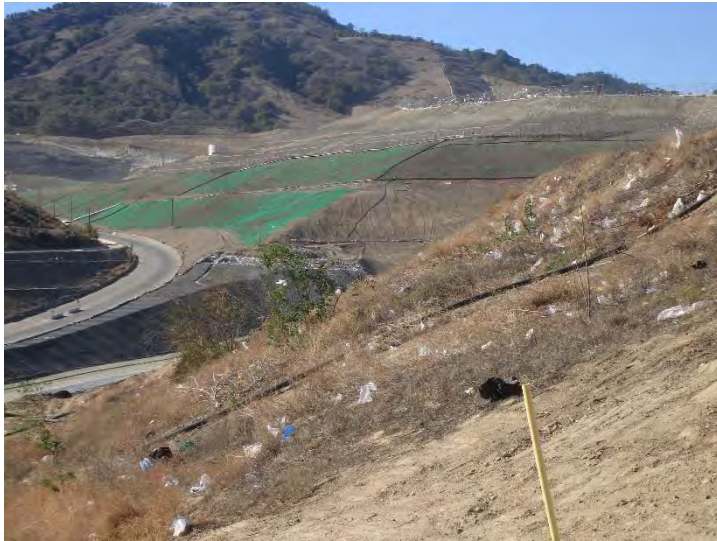
Photo 545: Site 12-2 pm: November 16, 2015
