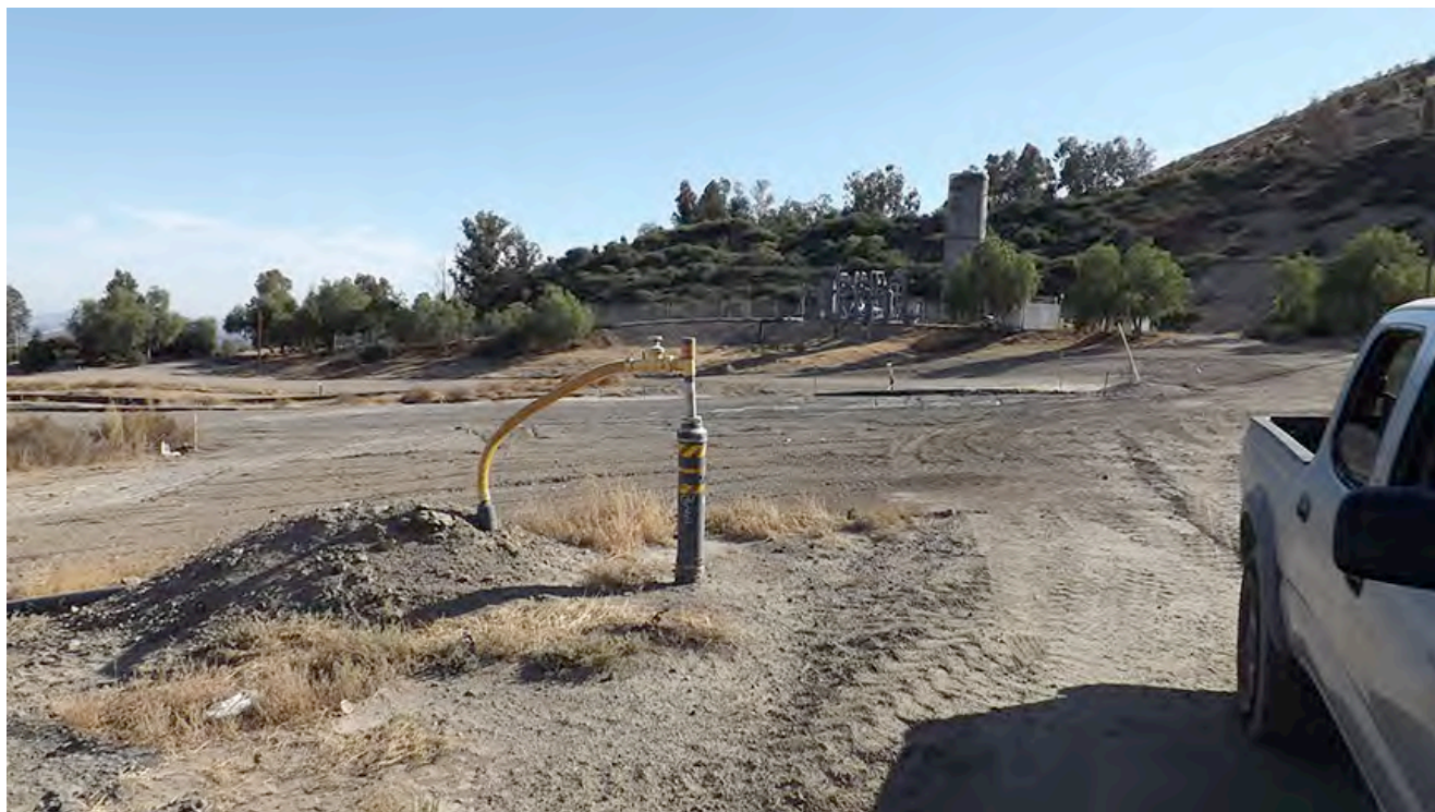
Existing gas valve at Deck B
