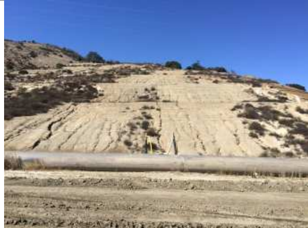
Photo 2. Facing west at the bare slope on the northern-half of the county-side mitigation area. Plant growth remains to be problematic due to erosion, a hard soil surface layer, and boron toxicity.
