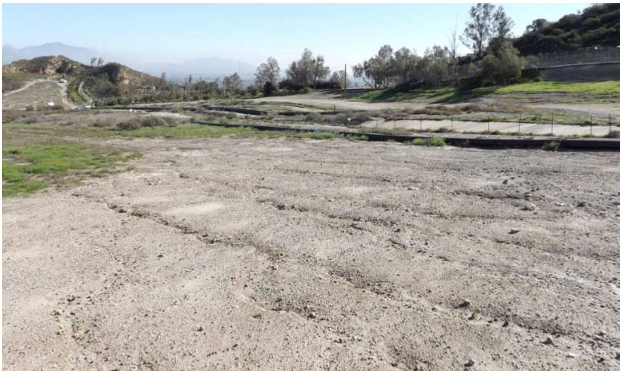
Deck B bare soil conditions with erosion
