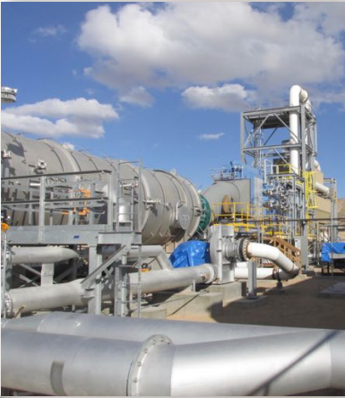
Thermal Oxidizer
