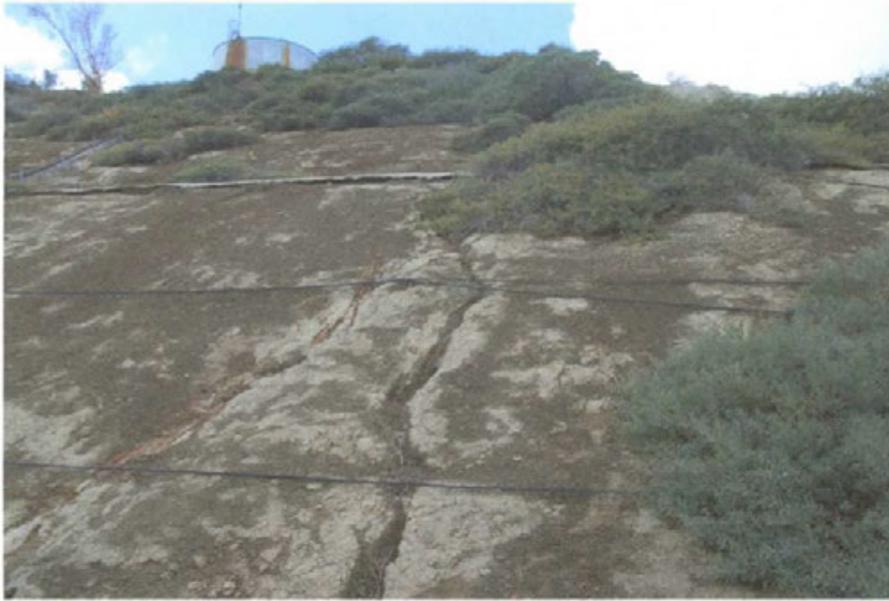
Photo 20: Undermined drainage channel on hillside near Flare 1
