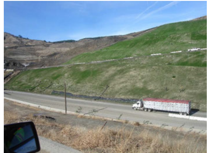
Photo 248: Closure Turf & Posi-Shell: January 10, 2018
