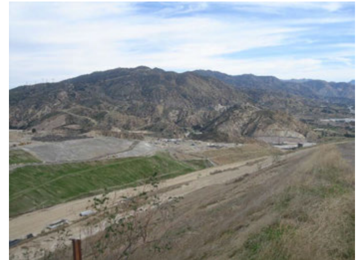
Photo 264: Closure Turf & Posi-Shell: January 30, 2018
