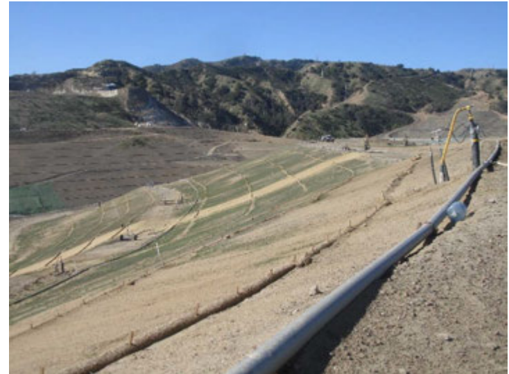
Photo 374: CC3B South Hydroseeded Slopes: February 20, 2018
