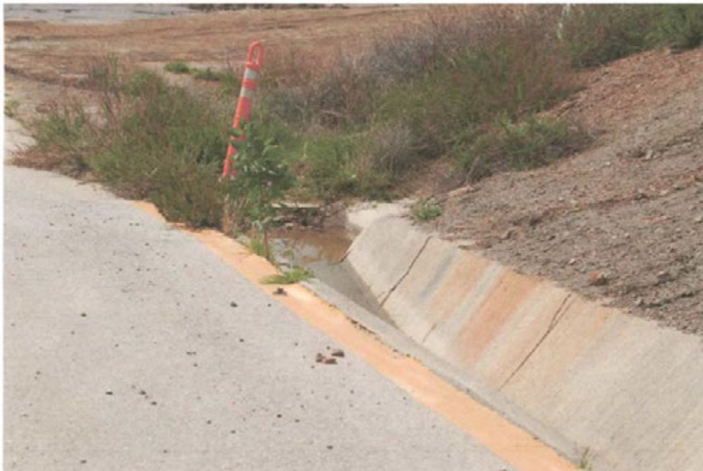
Photo 14: Blocked drainage ditch along access road to Flare 9-11
