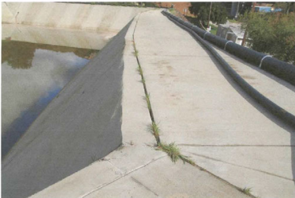
Photo 19: Gap between slabs at Terminal Basin
