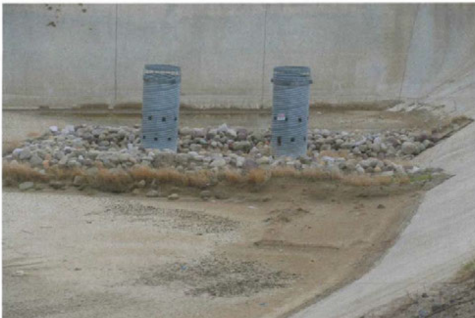
Photo 10: Sediments Accumulated in Basin B
