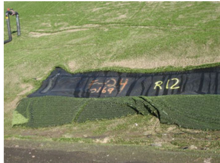
Photo 252: Closure Turf & Posi-Shell: January 10, 2018
