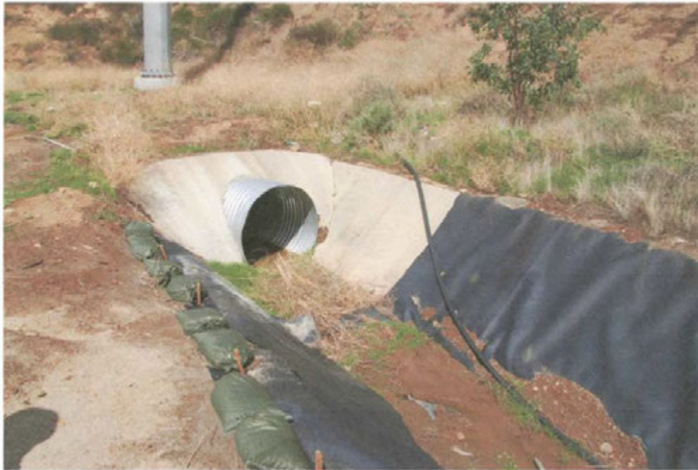
Photo 13: Sediment and debris on geomembrane lined channel between Basin B and Basin D
