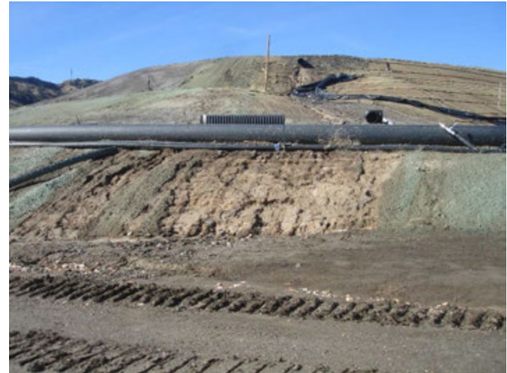
Photo 342: CC3B Slope Drainage Erosion: January 10, 2018
