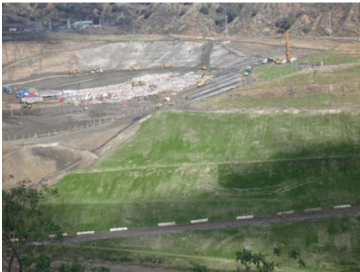
Photo 295: Posi-Shell and Closure Turf: March 14, 2018
