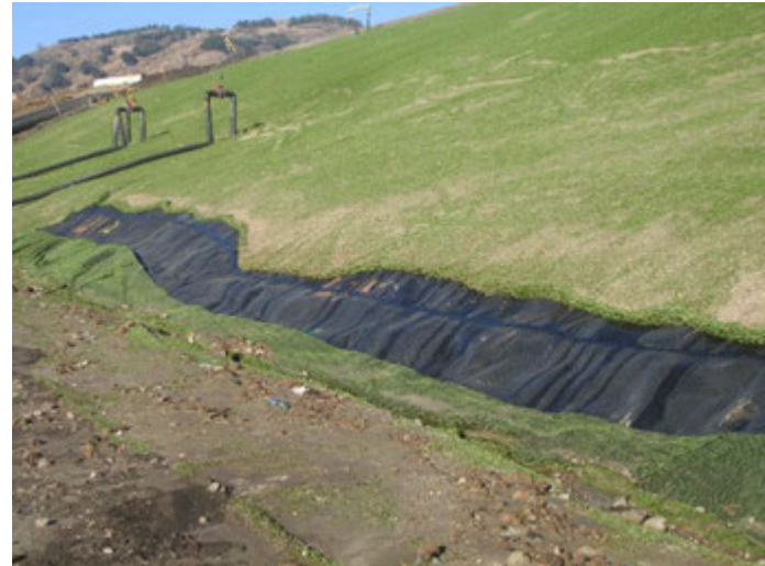
Photo 254: Closure Turf & Posi-Shell: January 10, 2018
