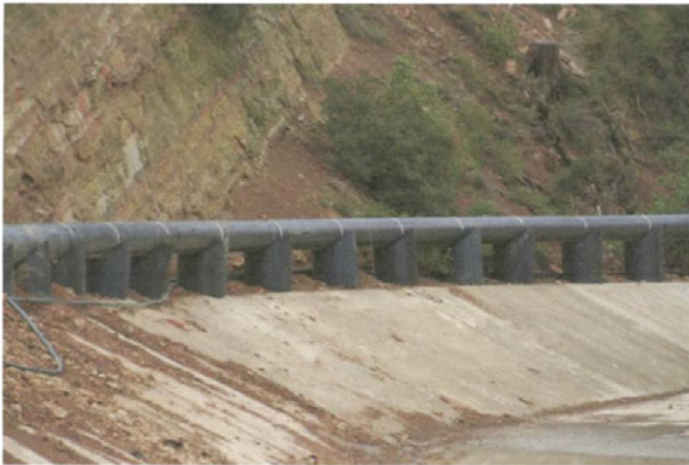
Photo 9: Leaning Supports of LFG Header to Flare 3 in Basin A
