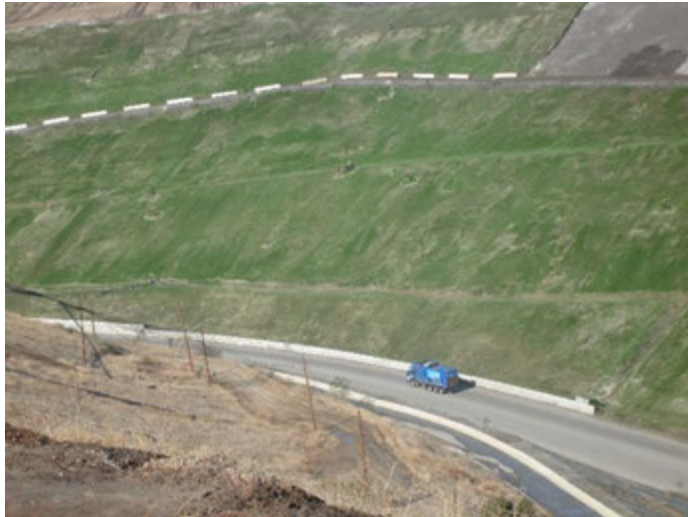
Photo 249: Closure Turf & Posi-Shell: January 10, 2018
