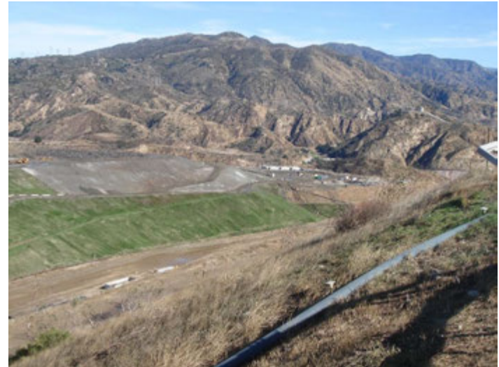
Photo 246: Closure Turf & Posi-Shell: January 10, 2018
