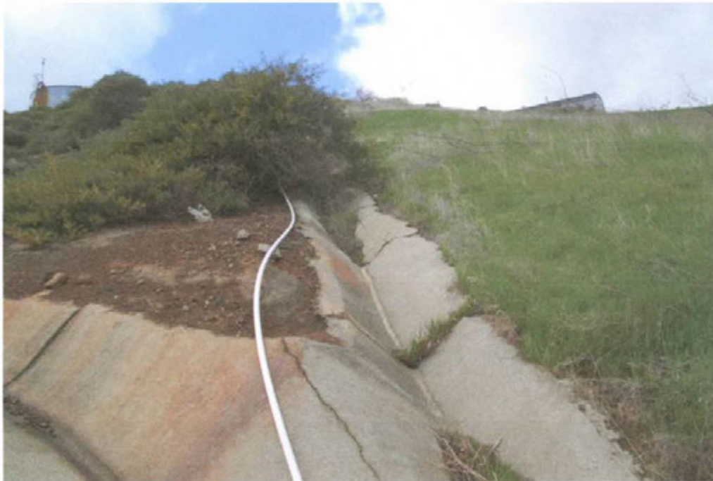
Photo 22: Cracks in drainage channel on hillside near Flare 1
