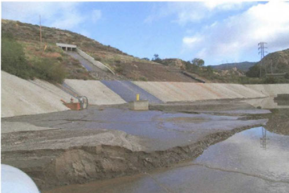
Photo 4: Sediments in Terminal Basin Upstream of Gabion Wall
