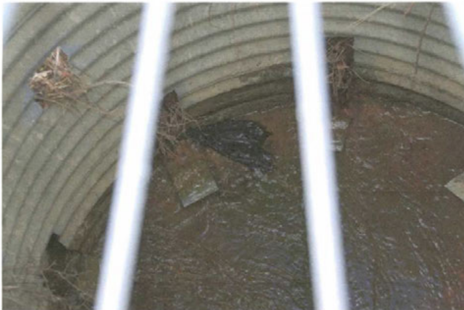
Photo 8: Stormwater Draining through Weepholes in Risers in Basin A
