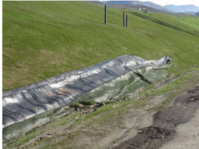
Photo 256: Closure Turf & Posi-Shell: January 10, 2018
