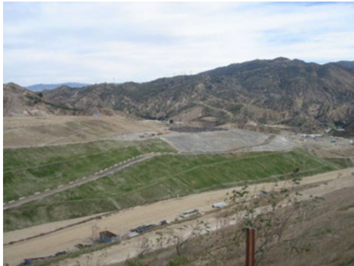
Photo 263: Closure Turf & Posi-Shell: January 30, 2018
