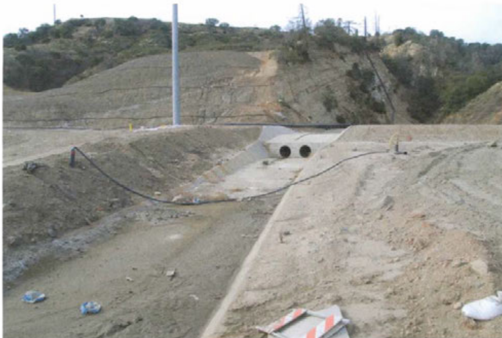
Photo 8: Cleaned up Drain Pipes of Basin A
