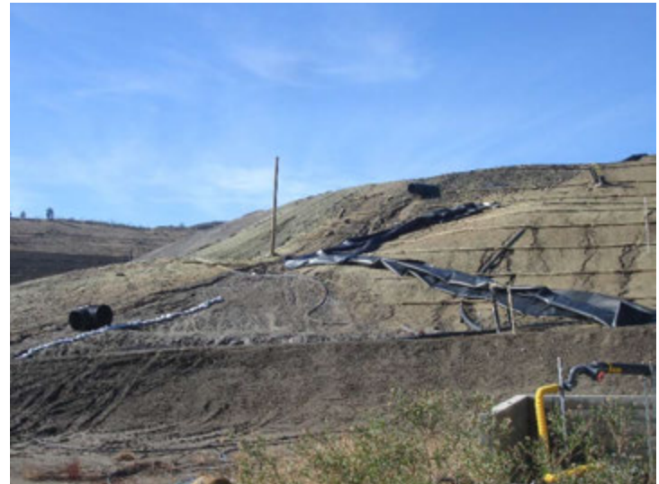
Photo 340: CC3B Slope Drainage Failure: January 10, 2018
