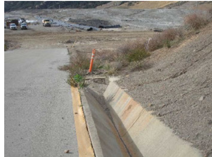
Photo 476: Plugged Drain at Flare 9-11 Access Road: January 30, 2018
