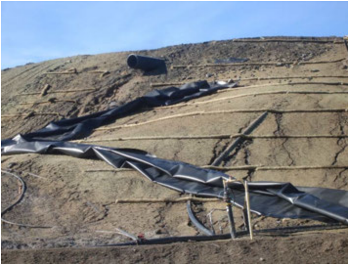
Photo 341: CC3B Slope Drainage Failure: January 10, 2018
