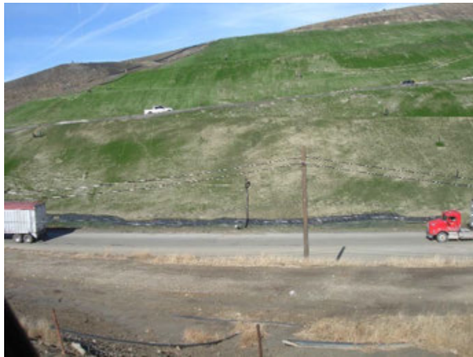
Photo 247: Closure Turf & Posi-Shell: January 10, 2018
