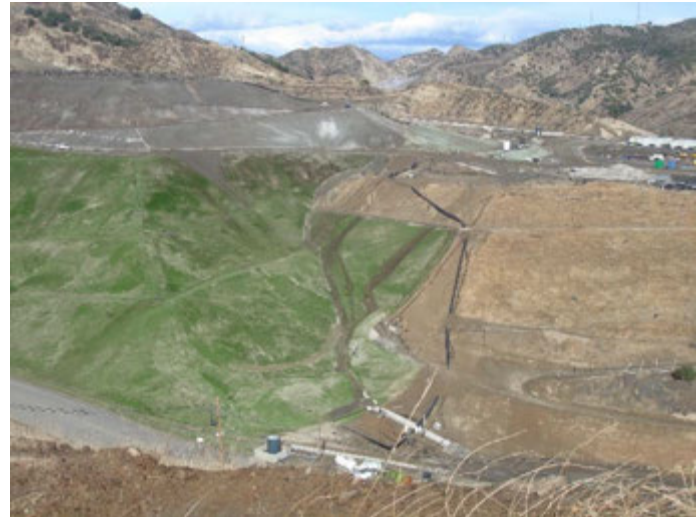
Photo 250: Closure Turf & Posi-Shell: January 10, 2018
