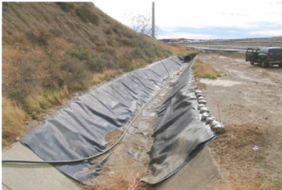
Photo 11: Repaired and Re-attached Geomembrane in Shotcrete Channel between Basin D and Access Road to Flare 9 and 10
