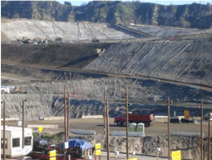
Photo 105: CC4A Part 1 with Posi Shell Slopes: March 29, 2018
