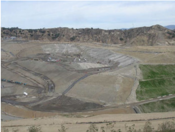
Photo 257: Closure Turf & Posi-Shell: January 30, 2018
