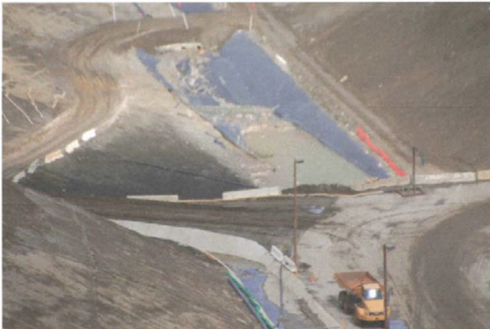
Photo 1 : Waste placement at Cell CC4
