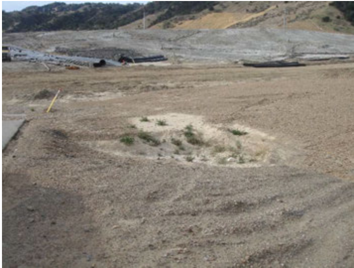
Photo 477: Plugged Drain at Flare 9-11 Access Road: January 30, 2018
