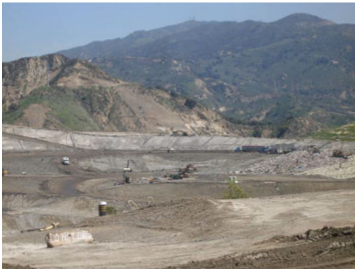
Photo 107: CC4A Part 1 with Posi Shell Slopes: March 29, 2018
