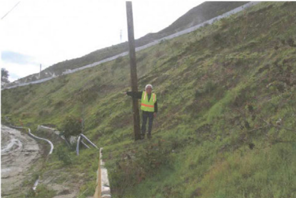
Photo 17: Sloughing and Tilted Utility Pole on Embankment of Main Access Road near Entrance of Terminal Basin
