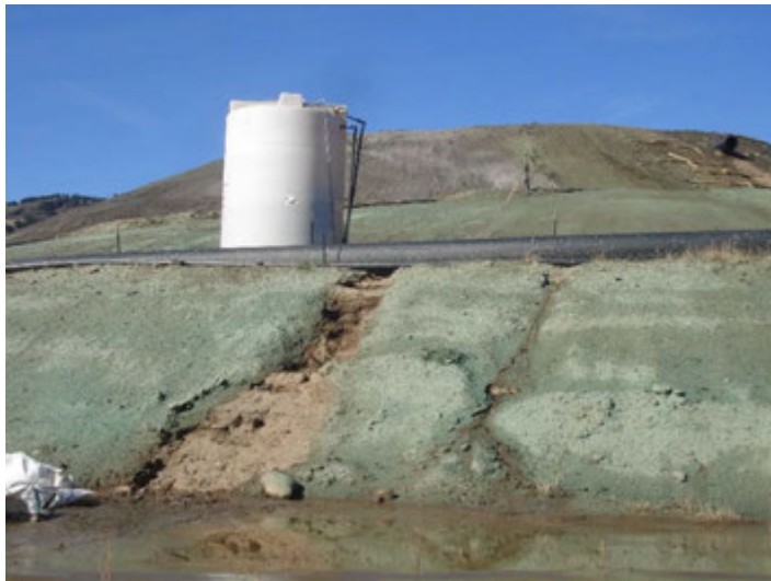
Photo 343: CC3B Slope Drainage Erosion: January 10, 2018
