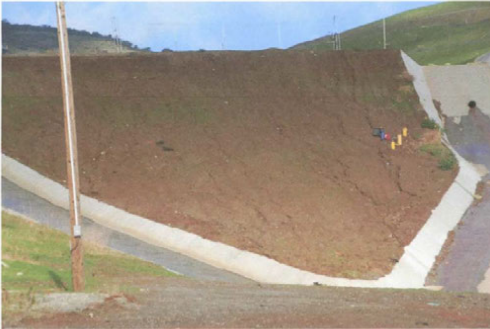
Photo 3: Erosion on upstream face of earthen basin embankment at Cell CC3
