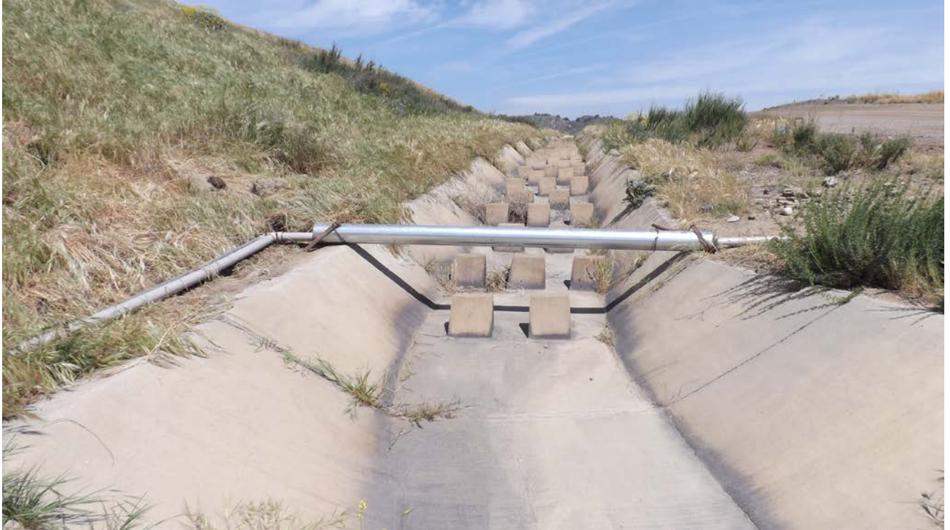
Irrigation mainline and galvanized sleeving over concrete drainage channel
