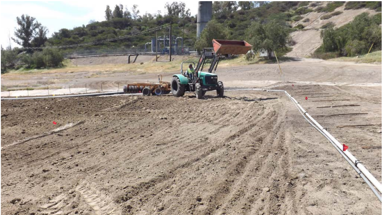
Disking of soils to loosen up compacted surface due to delay in construction and "crusting" of soil surface
