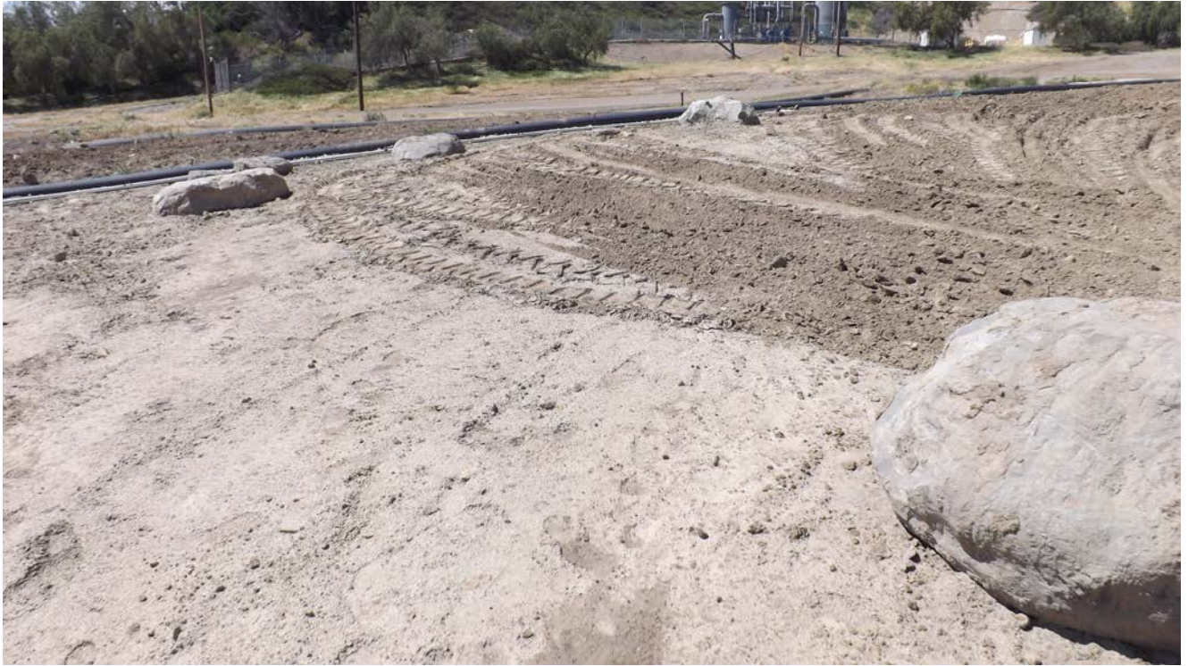
Boulder placement and area of deck to be loosened by disking
