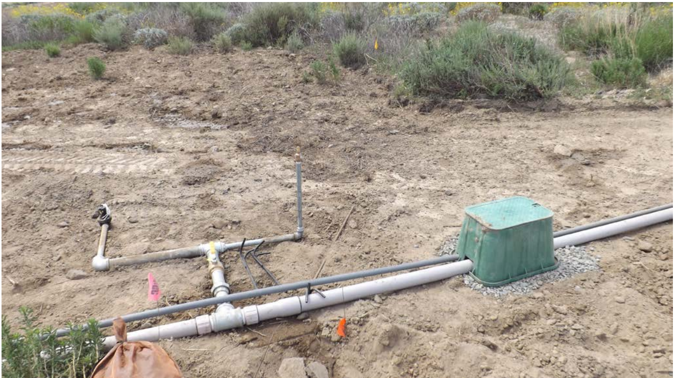
On-Grade Irrigation mainline and valve manifold and hose bid
