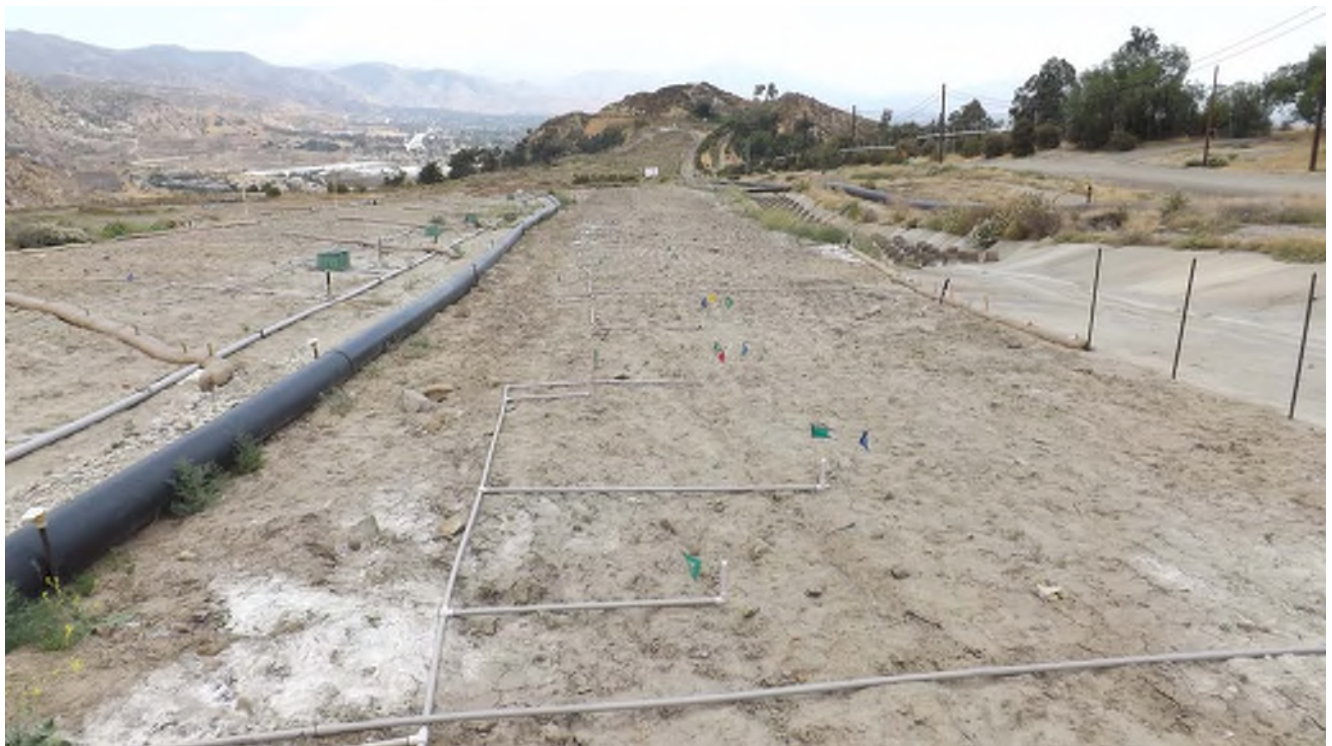
View east along drainage channel and on grade gas pipe. Irrigation laterals are installed.
