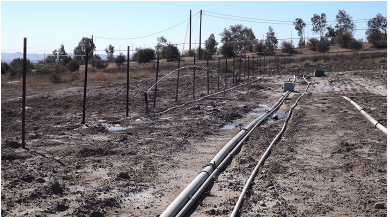
Irrigation was not properly working at time of visit. Appeared to be a pressure issue with radius throw only 1/3 of designed distance
