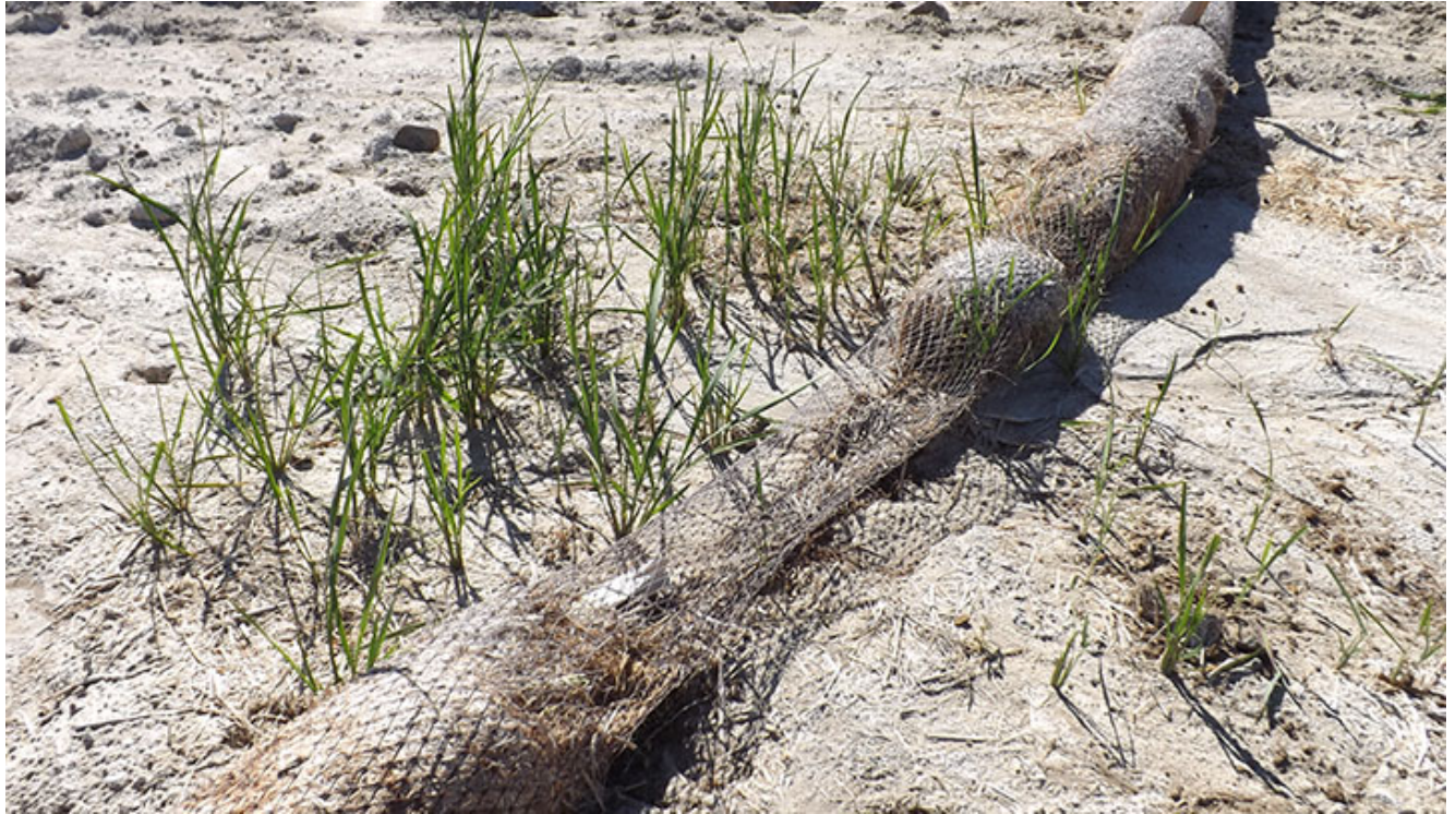
New grasses germinated at swale line (straw wattle repair needed in some areas)
