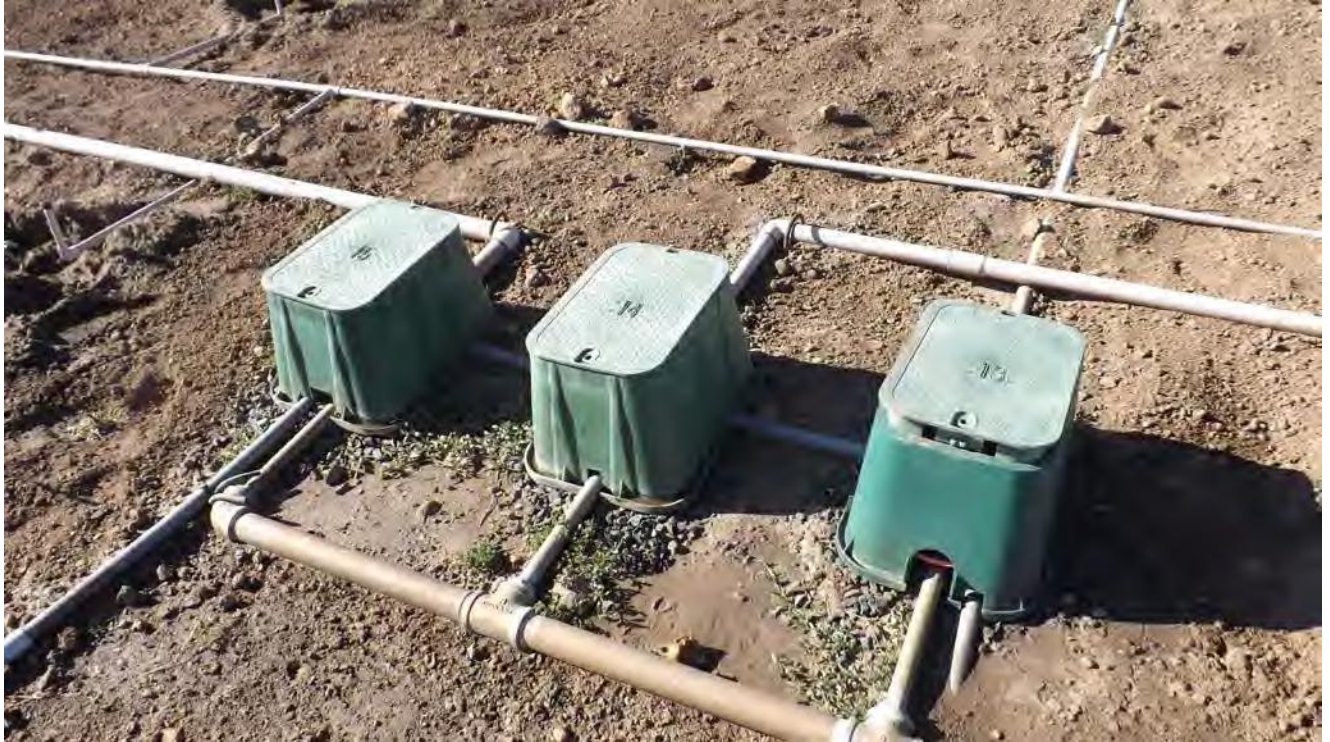
On-grade manifolded valves with branded valve numbering and staked laterals
