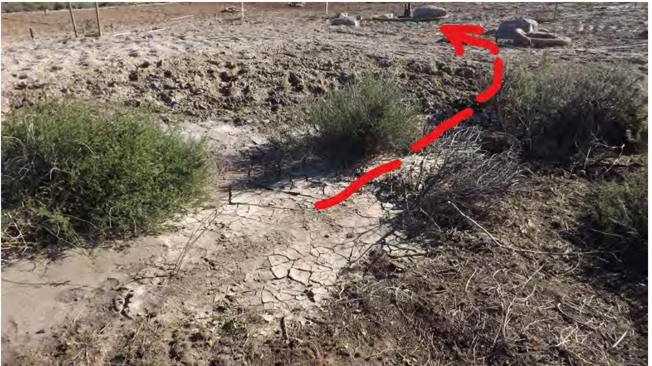
Low spot on deck where water is ponding. Contractor to provide positive drainage to the south-east and cut in swale as marked to link up with swale near boulders on other side.
