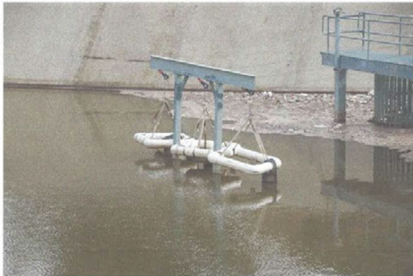
Photo 4: Raised skimmers at Terminal Basin
