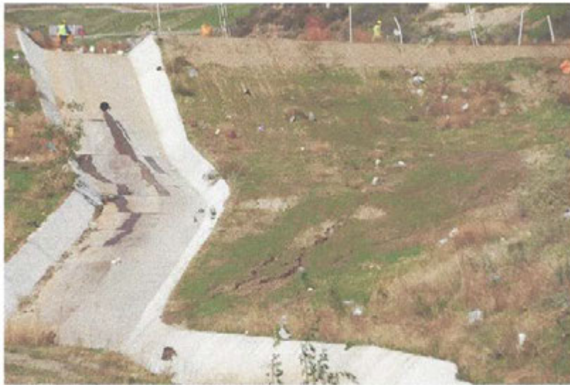
Photo 7: Erosion on slope of embankment for basin CC3
