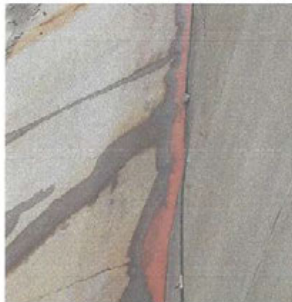
Photo 6: Reddish deposit form water seeping through weep holes at the bottom of the wall
