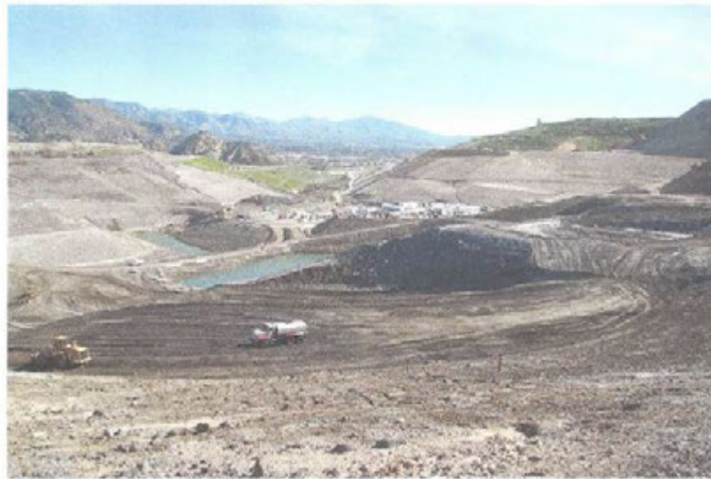
Photo 10: Water collected in temporary basin at toe of buttress
