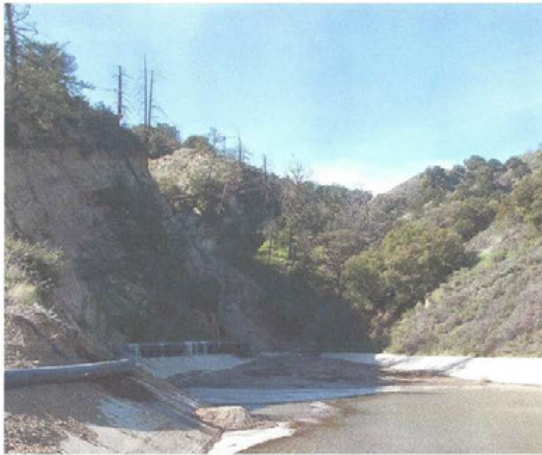
Photo 9: Sediments at back of Basin A
