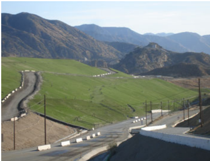
Photo 171: Posi-Shell and Closure Turf: January 22, 2019
