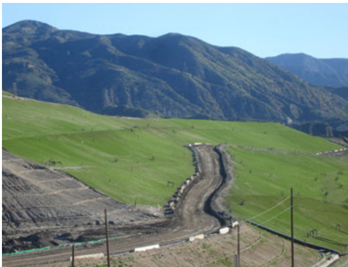
Photo 119: Posi-Shell and Closure Turf: January 22, 2019
