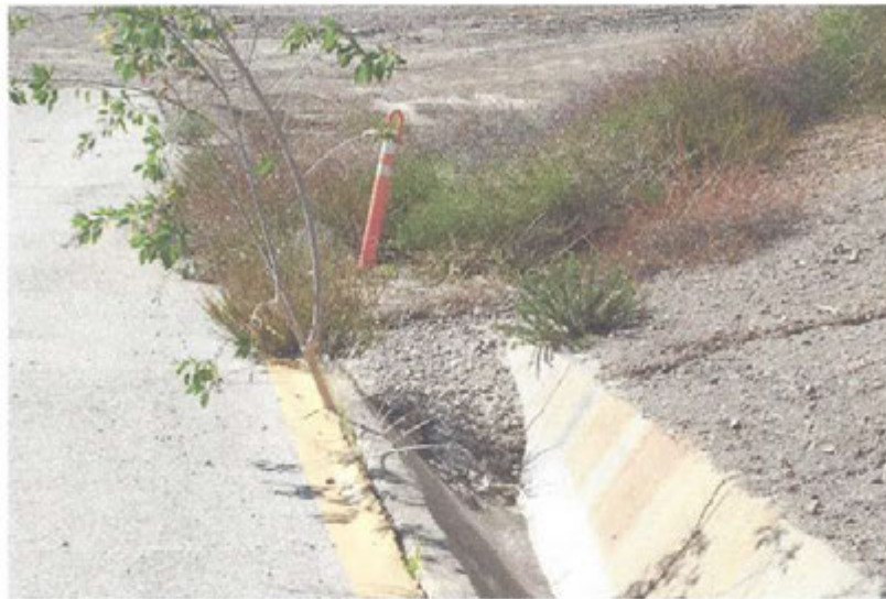
Photo 13: Sediments plugging drain at end of ditch along access road to Flares 9-11
