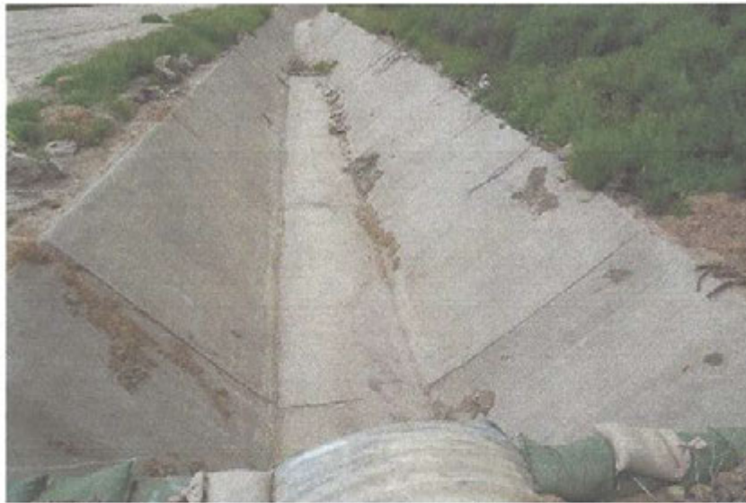
Photo 13: Reinstalled CMP in channel segment between Basin D and power pole
