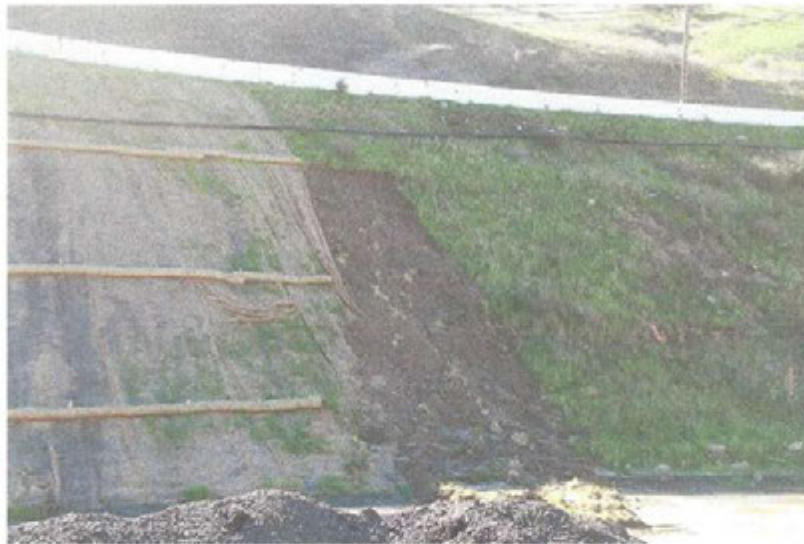
Photo 1: Soil sloughing on slope of embankment of main access road
