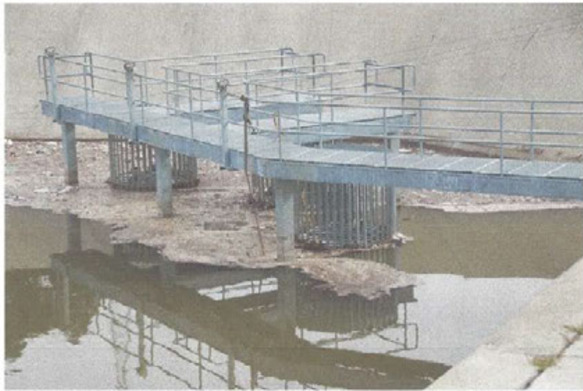
Photo 5: Water level and waste accumulation near decant towers at Terminal basin
