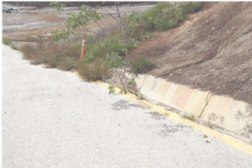
Photo 10: Sediments plugging drain at end of ditch along access road to Flares 9-11
