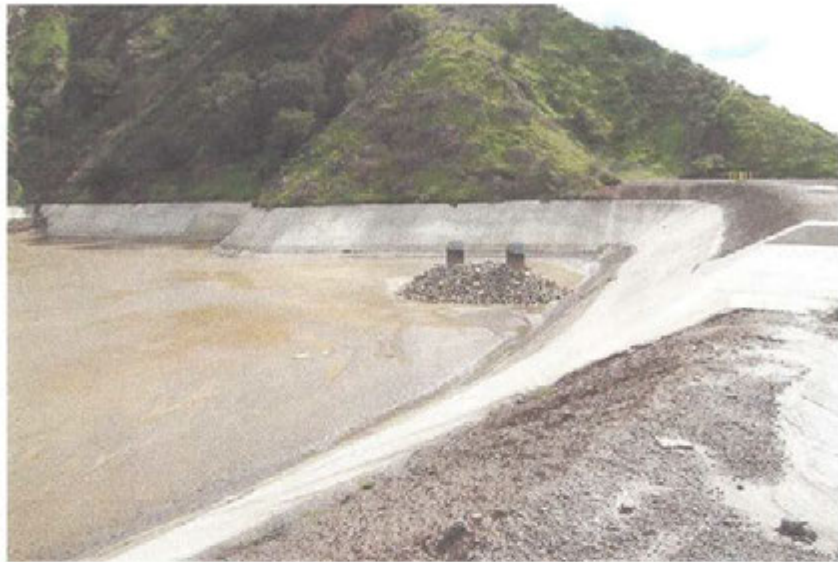
Photo 9: Sediment in basin B
