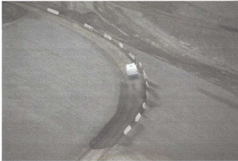
Figure 19: Moisture conditioning on roads
