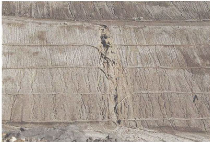
Figure 19: Deep erosion gully exposing refuse on slope of Cell CC3 Phase 3
