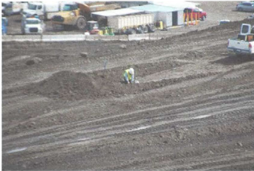
Figure 15: CQA monitoring of buttress
