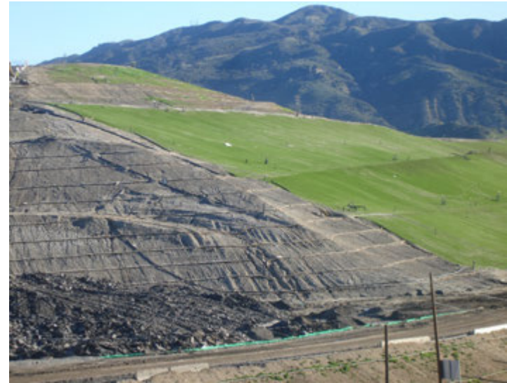
Photo 118: Posi-Shell and Closure Turf: January 22, 2019
