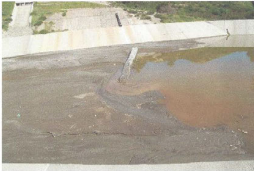
Photo 3: Sediment level in Terminal Basin
