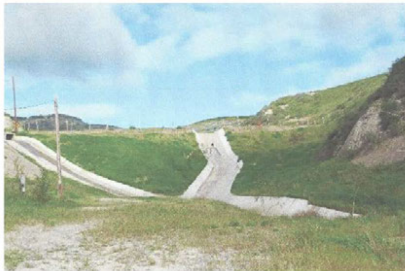
Photo 8: Vegetation covering erosion gullies on slope of embankment for earthen basin CC3
