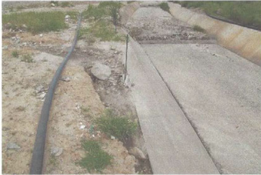
Photo 9: Erosion along edge of channels between Basin B and Terminal Basin and sediments trapped on gabion
