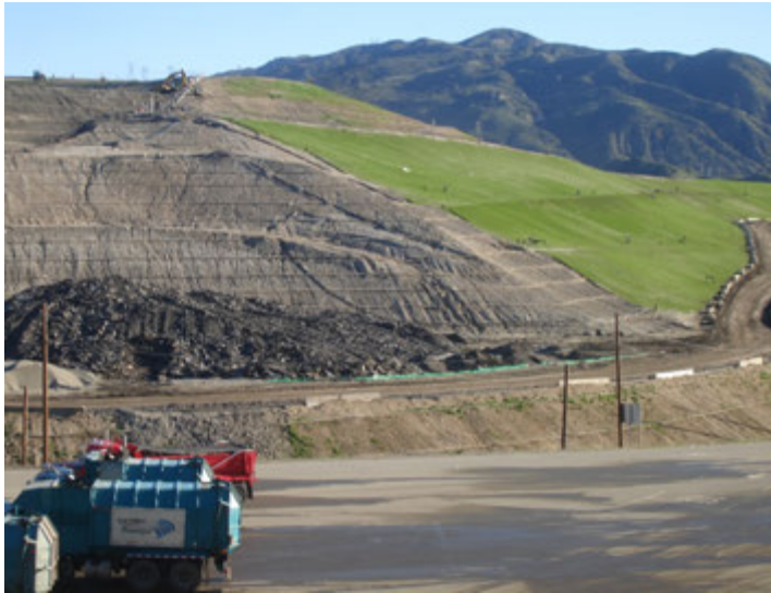
Photo 117: Posi-Shell and Closure Turf: January 22, 2019
