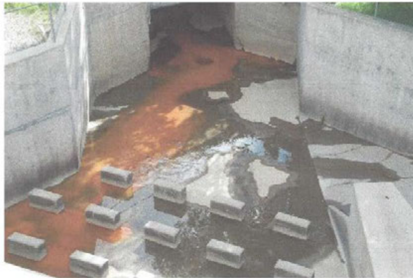
Photo 7: Reddish water exiting Terminal basin
