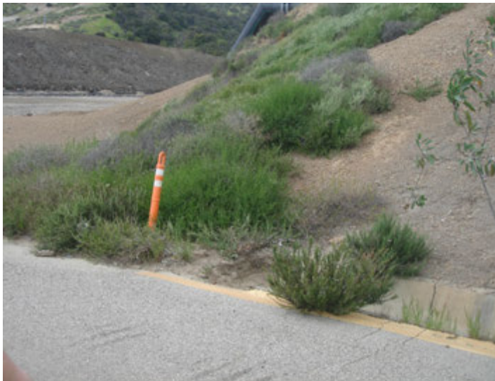
Photo 183: County Flare Road Plugged Drainage: March 28, 2019
