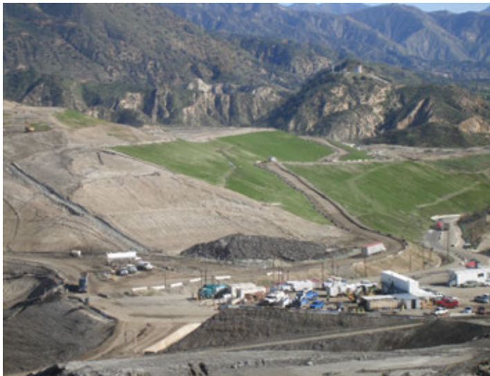
Photo 115: Posi-Shell and Closure Turf: January 22, 2019
