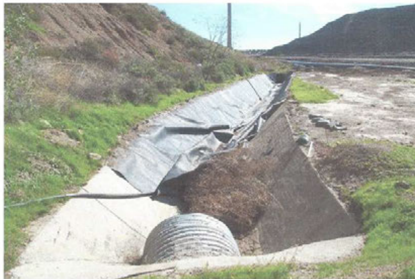
Photo 14: Damage to membrane on first segment of channel west of the access road to Flares 9-11
