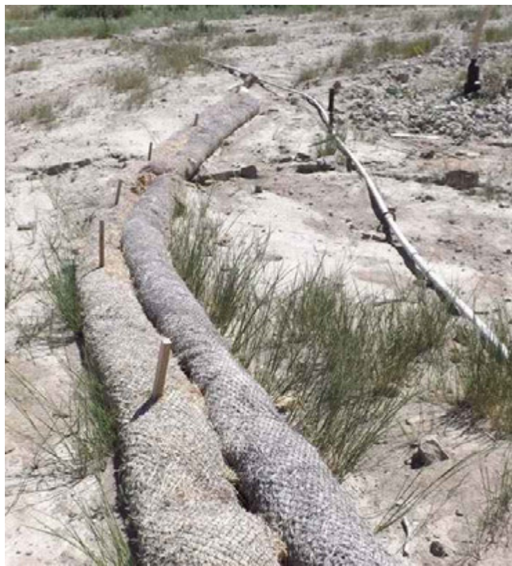
New straw wattle installation behind original to help eliminate erosion
