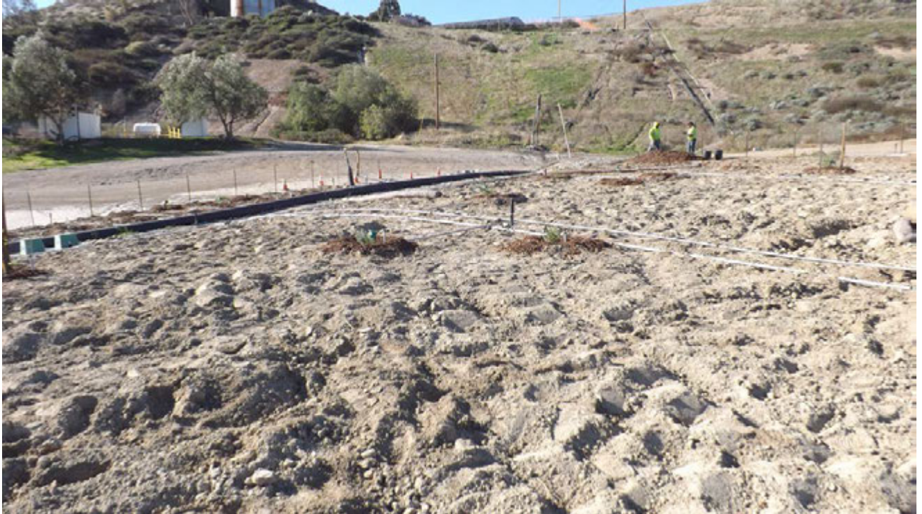
View looking south-west – Deck B
