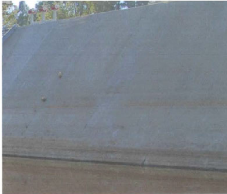
Photo 7: Vegetation in cracks of inside wall of Terminal basin
