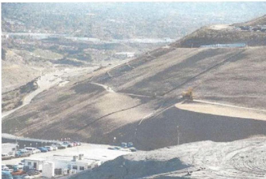
Photo 1: Settlement depression on slope above access road near administration pad
