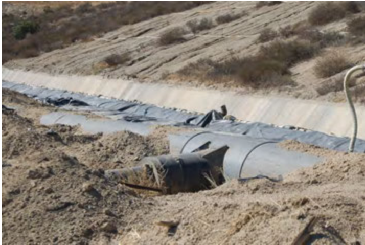
Photo 285: Sacrificial Liner Replacement Near County Sage: October 13, 2018
