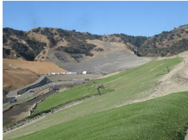
Photo 156: Posi-Shell and Closure Turf: October 23, 2018
