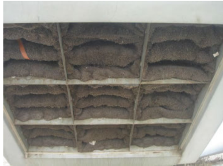
Photo 366: Flare 9 Blower Intake Air Filter: September 25, 2018
