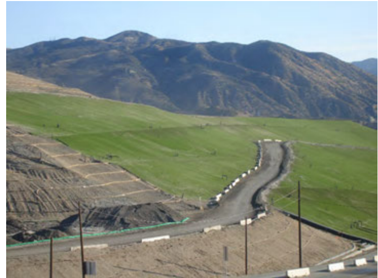
Photo 170: Posi-Shell and Closure Turf: November 20, 2018
