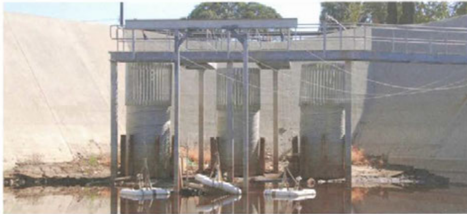
Photo 5: Sediment behind the decant towers of Terminal Basin
