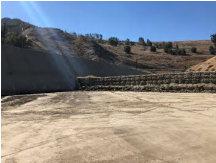
Photo 387: Terminal Basin Gabion Wall: July 24, 2018
