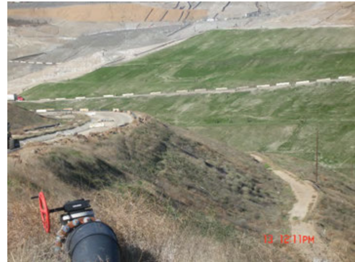
Photo 172: Posi-Shell and Closure Turf: December 13, 2018
