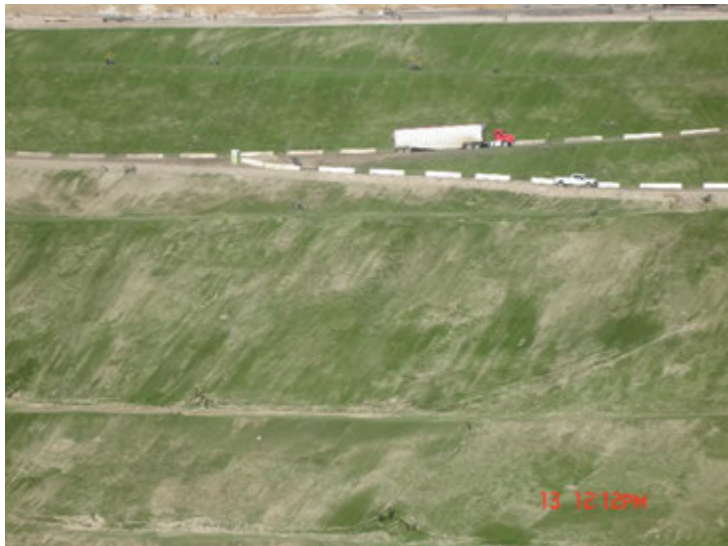
Photo 175: Posi-Shell and Closure Turf: December 13, 2018
