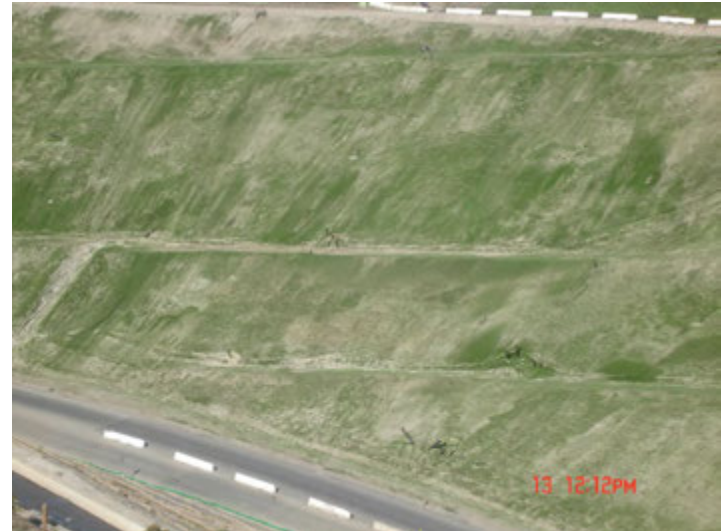
Photo 178: Posi-Shell and Closure Turf: December 13, 2018
