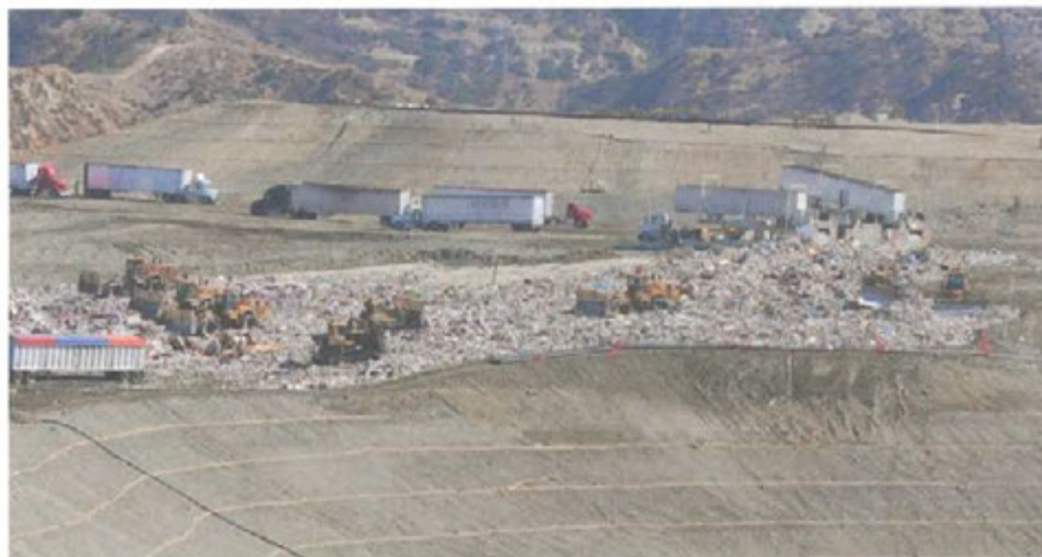
Photo 3: Tilters in use at waste face on Cell CC4 Part 1
