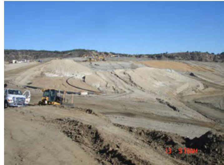
Photo 72: County Soil Stockpile Erosion Near CC-4 Parts 1&2: December 13, 2018
