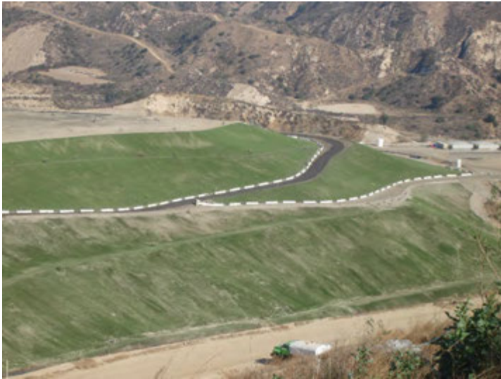
Photo 165: Posi-Shell and Closure Turf: November 20, 2018
