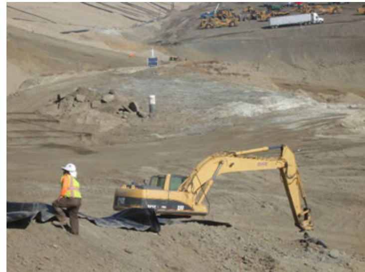
Photo 24: Basin A Temporary Outlet HDPE Channel: November 20, 2018
