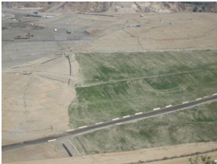
Photo 159: Posi-Shell and Closure Turf: November 6, 2018
