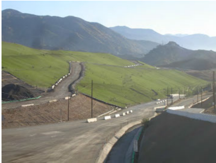
Photo 153: Posi-Shell and Closure Turf: October 23, 2018
