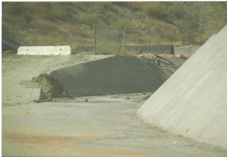
Photo 8: Earth check dam removed at Terminal basin
