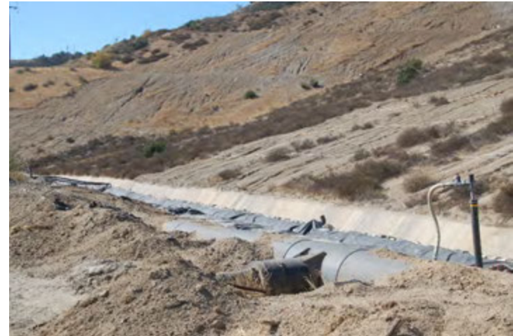
Photo 286: Sacrificial Liner Replacement Near County Sage: October 13, 2018
