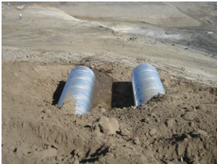
Photo 15: Basin A Temporary Outlet Pipes: November 6, 2018
