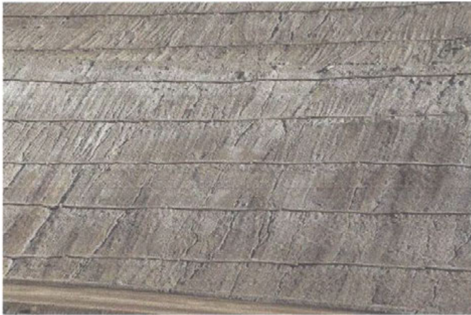
Photo 15: Minor erosion gullies on wattle protected slopes
