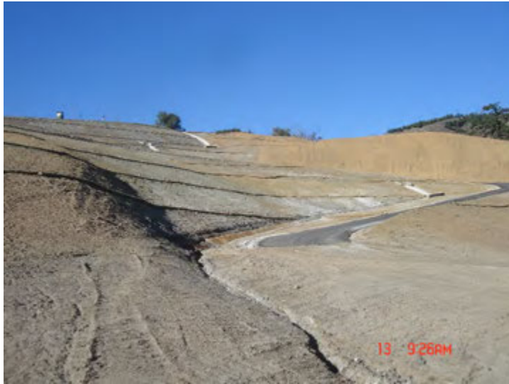
Photo 149: CC4 Part 3 Buttress Excavation Area: December 13, 2018
