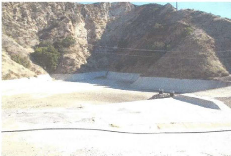
Photo 10: Basin D – small amount of sediments near intake towers
