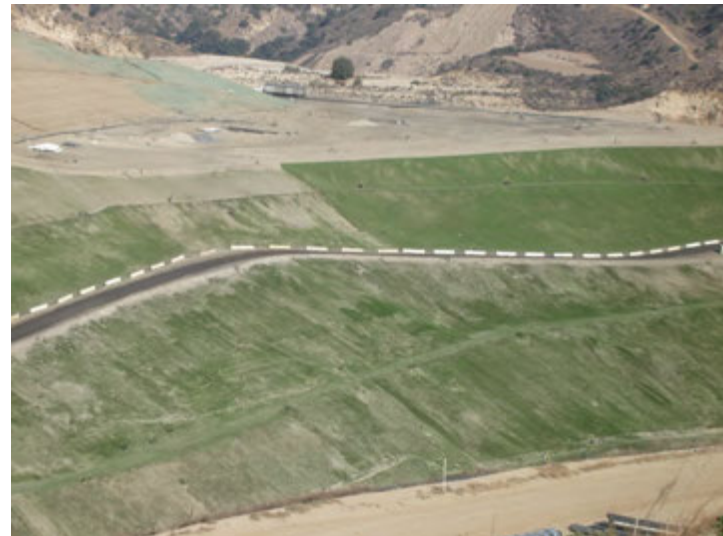
Photo 164: Posi-Shell and Closure Turf: November 20, 2018
