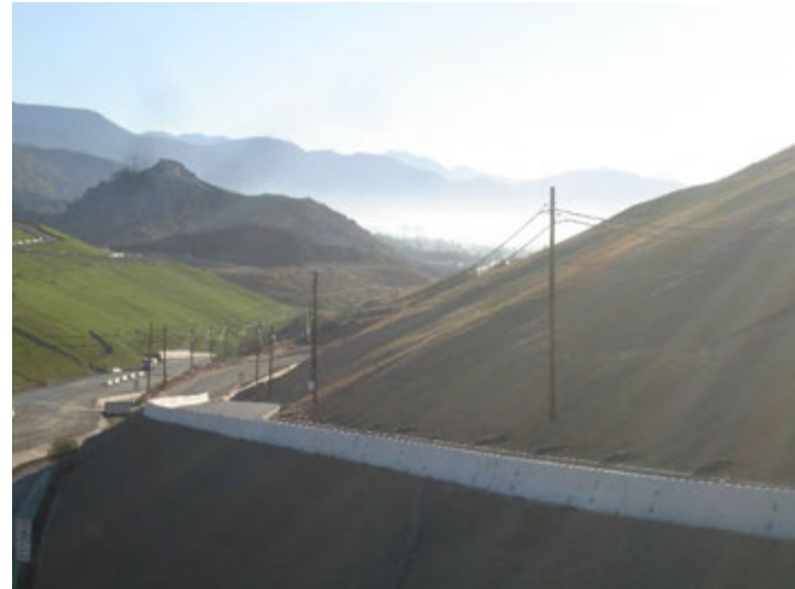
Photo 154: Posi-Shell and Closure Turf: October 23, 2018
