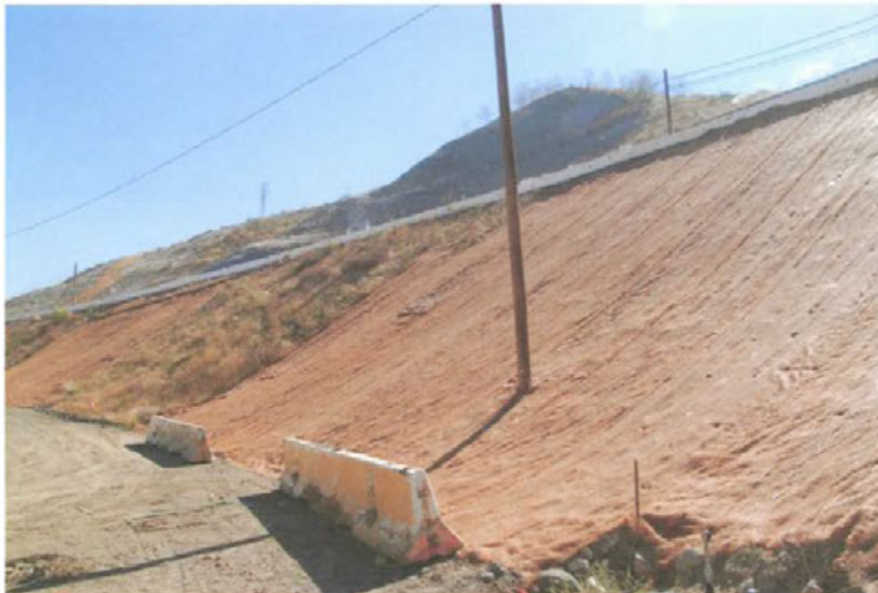
Photo 15: Repaired sloughed areas on slope of access road embankment at Terminal basin
