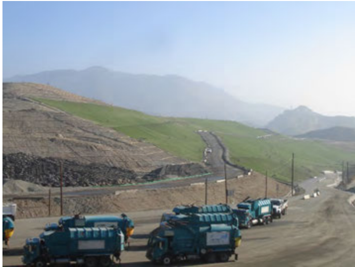
Photo 157: Posi-Shell and Closure Turf: November 6, 2018
