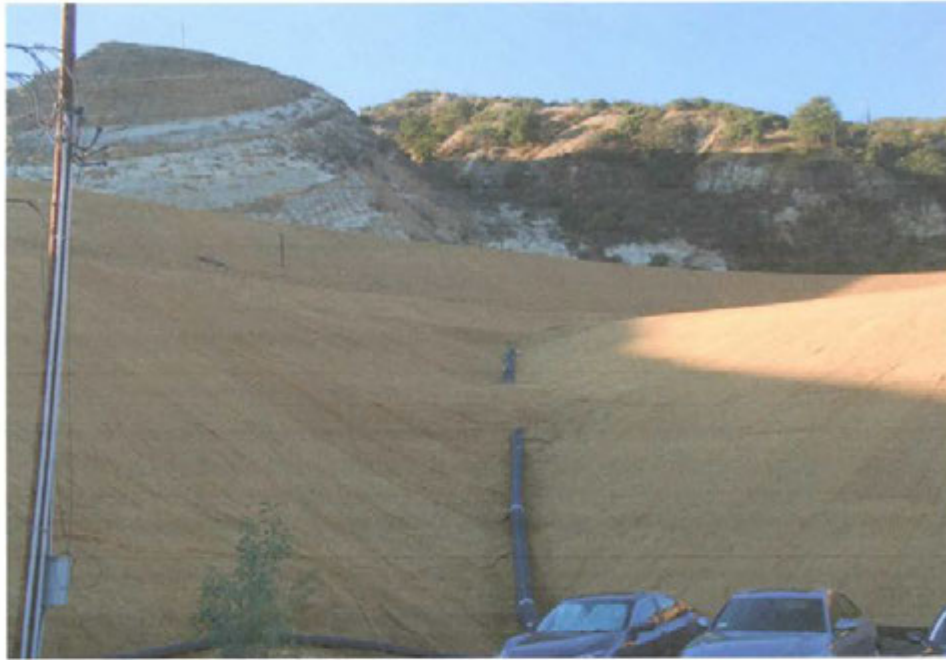
Photo 13: Erosion protection BMPs behind the administration buildings
