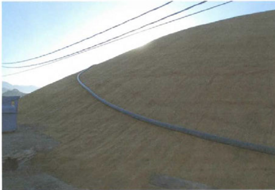
Photo 1: Erosion control blanket on access road near administration pad
