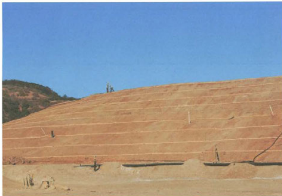
Photo 13: Erosion protection BMPs behind the administration buildings
