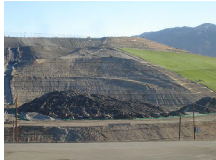
Photo 152: Posi-Shell and Closure Turf: October 23, 2018
