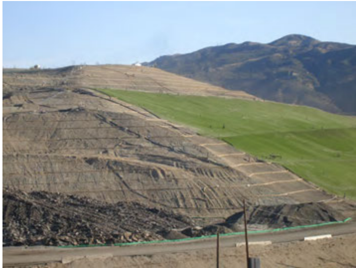
Photo 169: Posi-Shell and Closure Turf: November 20, 2018
