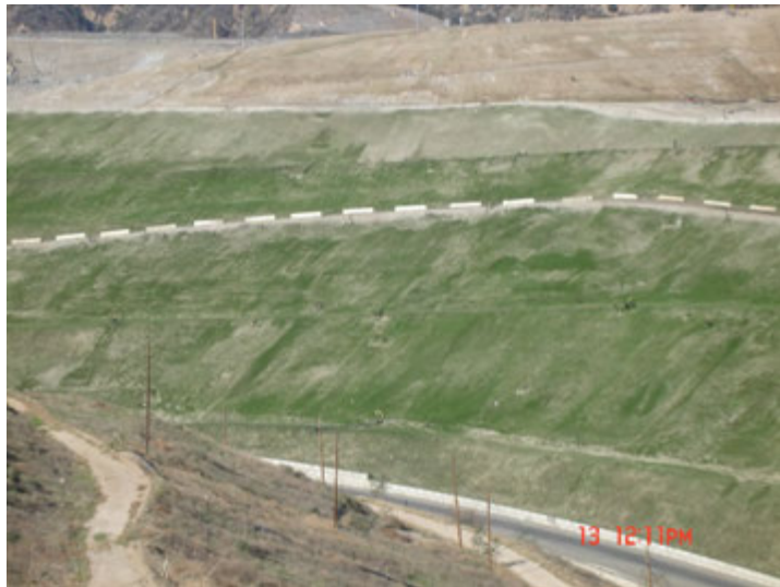
Photo 173: Posi-Shell and Closure Turf: December 13, 2018
