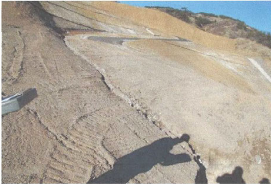
Photo 13: Erosion gully at end of unfinished drainage ditch along road to Flare 3
