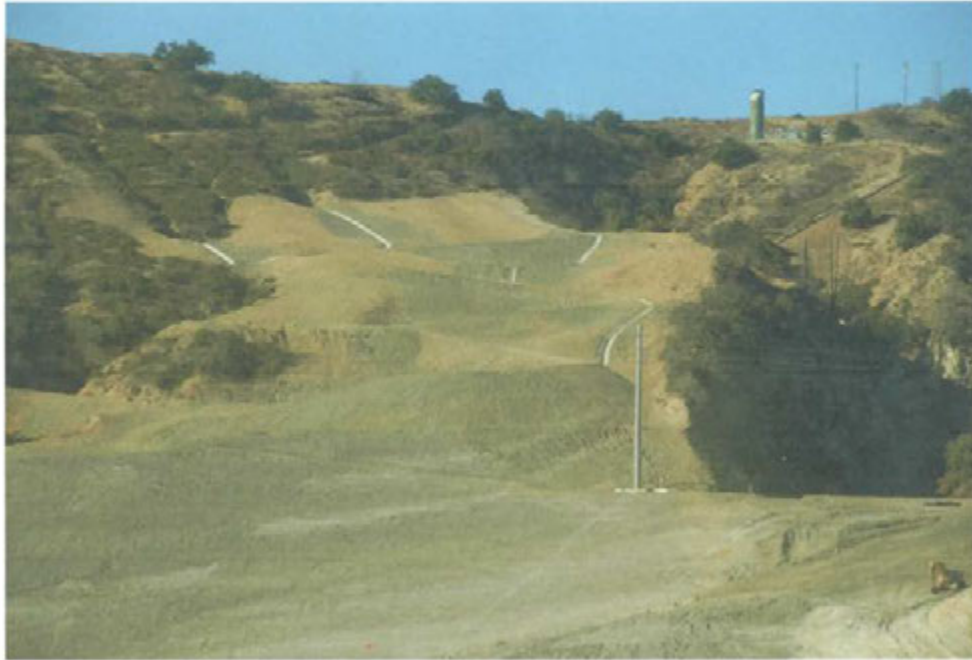
Photo 15: Shotcrete ditches on slope beneath Flare 3
