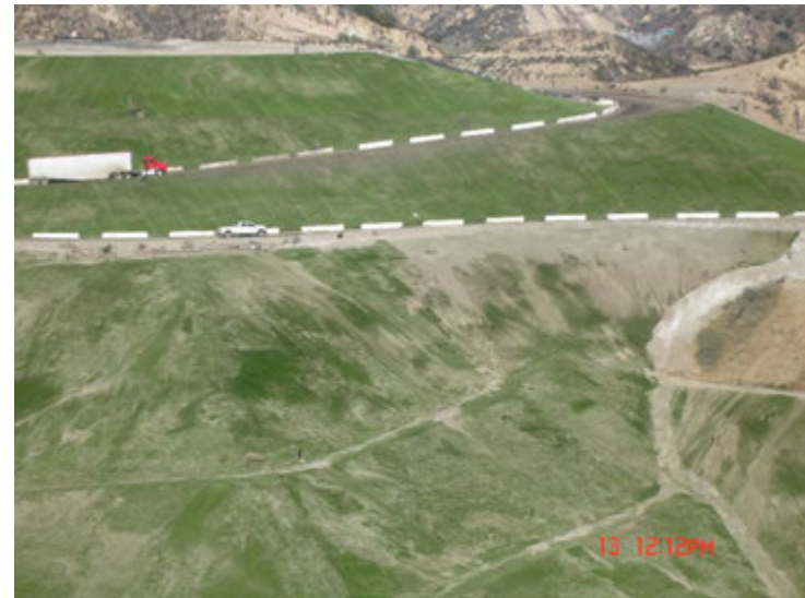
Photo 176: Posi-Shell and Closure Turf: December 13, 2018
