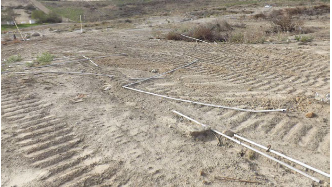
Irrigation Damage due to vehicular traffic
