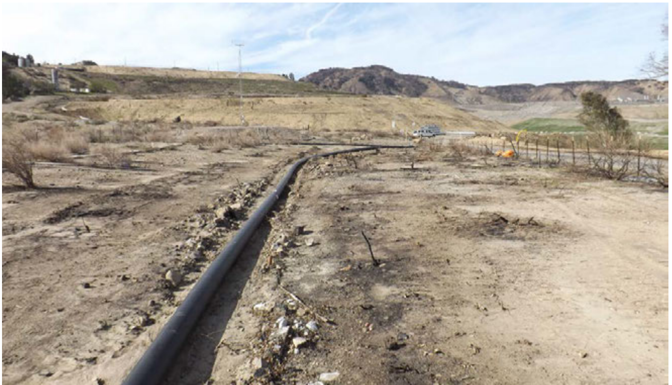
New on-grade gas line where previous vegetated swale used to exist
