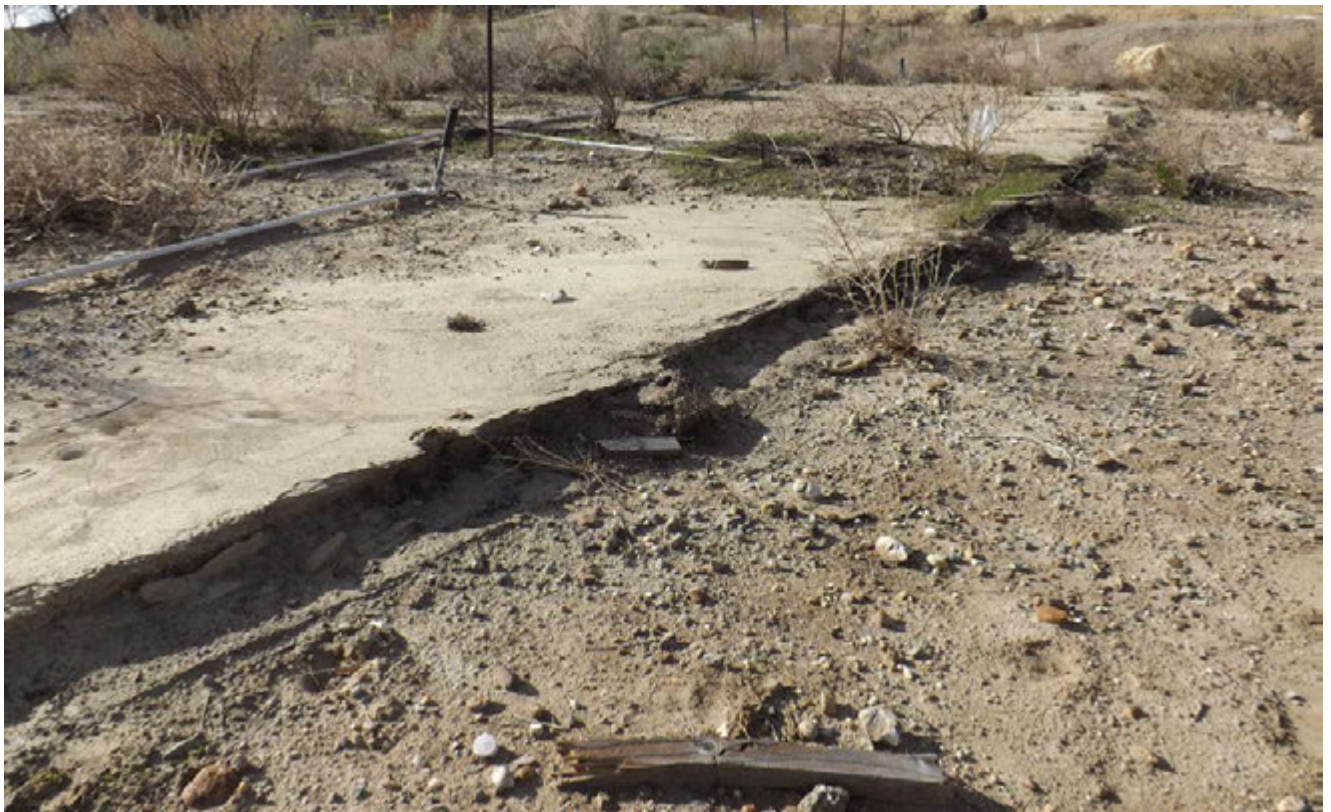
Previous area where straw wattle existed. Note sediment collection build up
