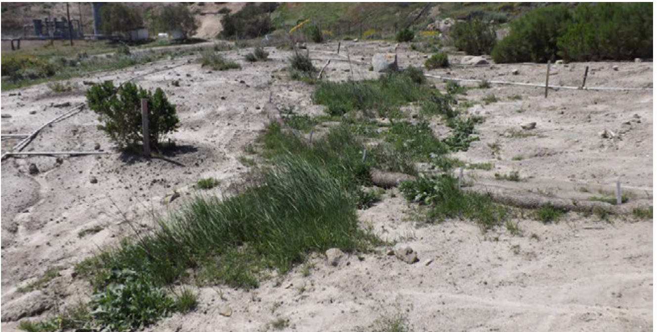
Straw wattles holding back sediment with native grasses ( Leymus ) within swaleline
