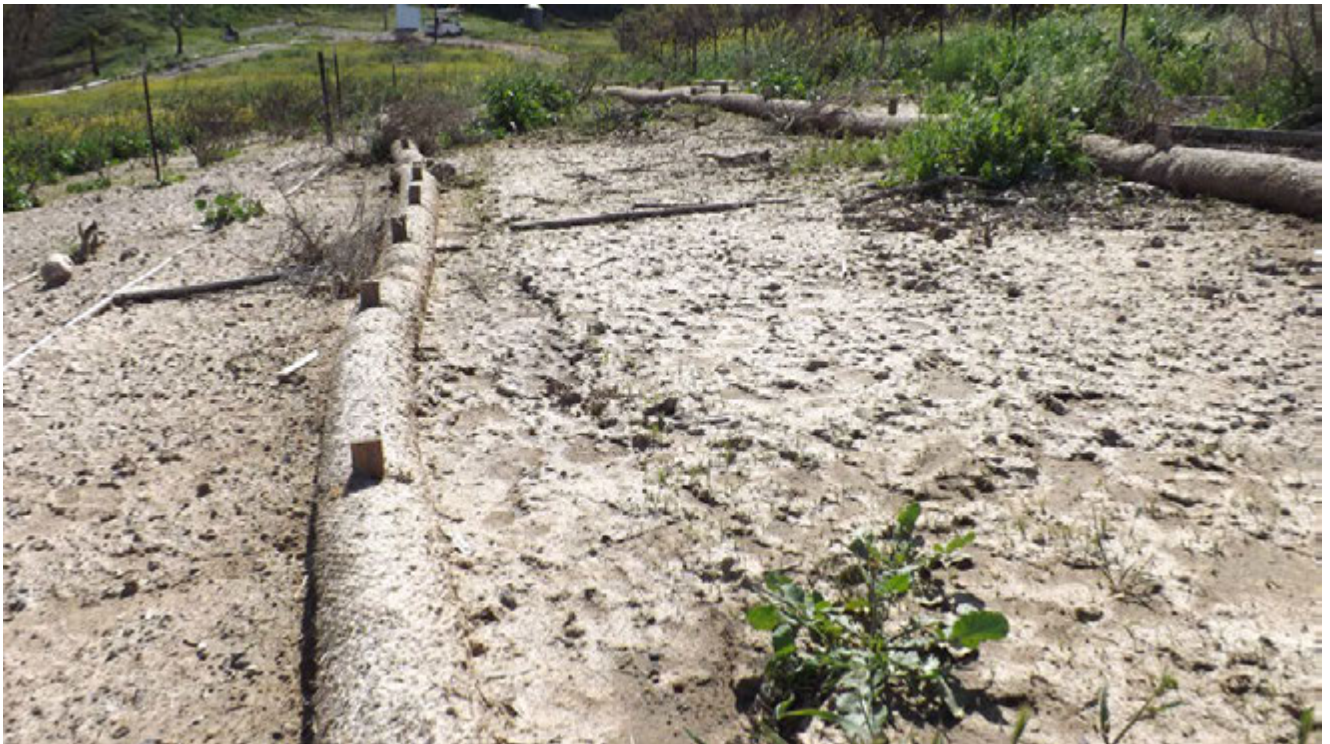
New Straw Wattles with emerging seedlings from recent hydroseeding
