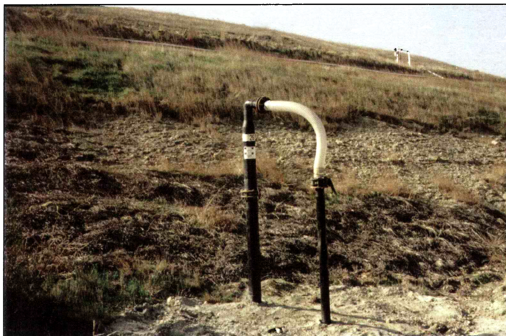
View of gas extraction wells at existing inactive landfill.
