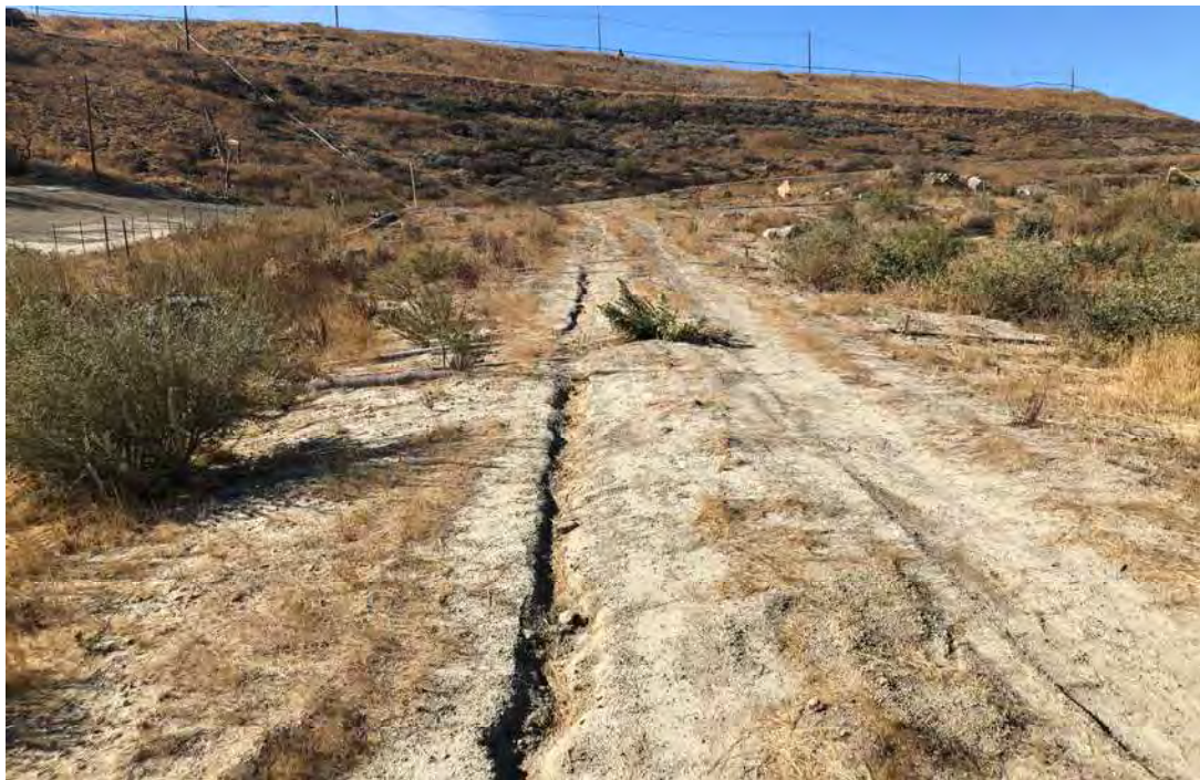
Rill erosion along access used during Fire. Recommend installing straw wattles to eliminate rill erosion (40' o.c.) and closing off west end of access road with T-Bar staking
