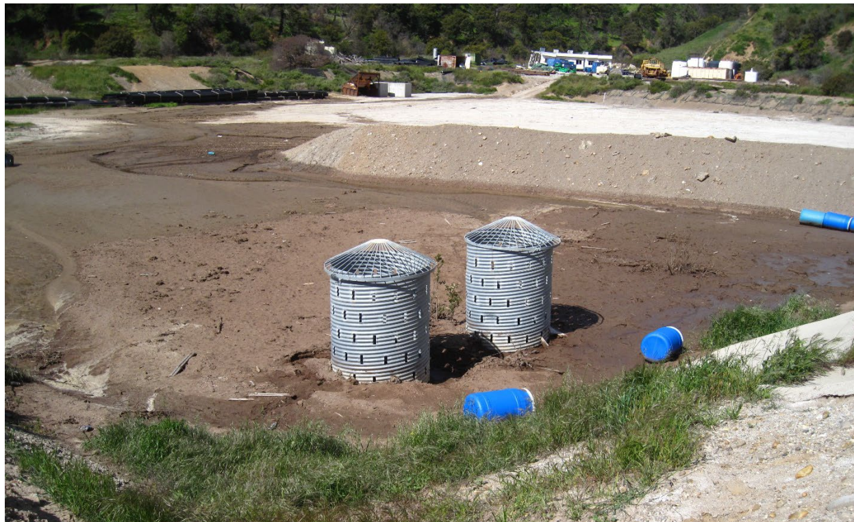
Photo 5. Sediment Basin D at the northern end of the canyon, looking north. This basin was in good condition and had ample capacity for stormwater runoff from the slopes to the north of the landfill.
