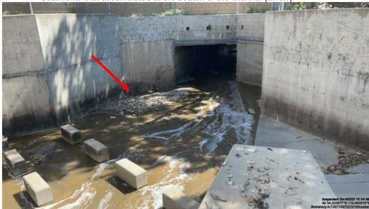
Photo 3. Water from the Terminal Basin flows offsite through this box culvert into Bull Creek, which is part of the Los Angeles County storm sewer system. Note the coarse-sized sediments that accumulated at the bottom of the channel (arrow).
