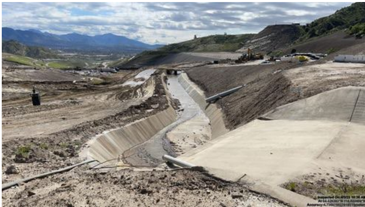
Photo 12. A view of the perimeter stormwater drainage channel surrounding the Landfill. The concrete lined channels were generally in good condition.
