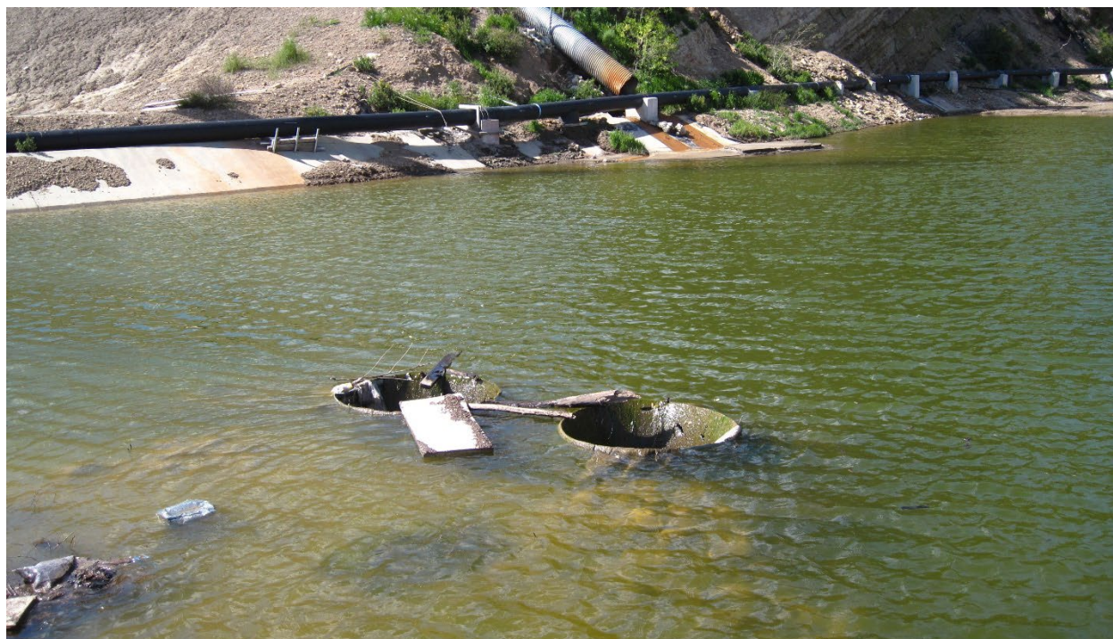
Photo 4. Sediment Basin A at the west edge of the Landfill. The top screens of the two risers had been damaged in recent storms and a significant amount of sediment accumulated at the bottom of the base.
