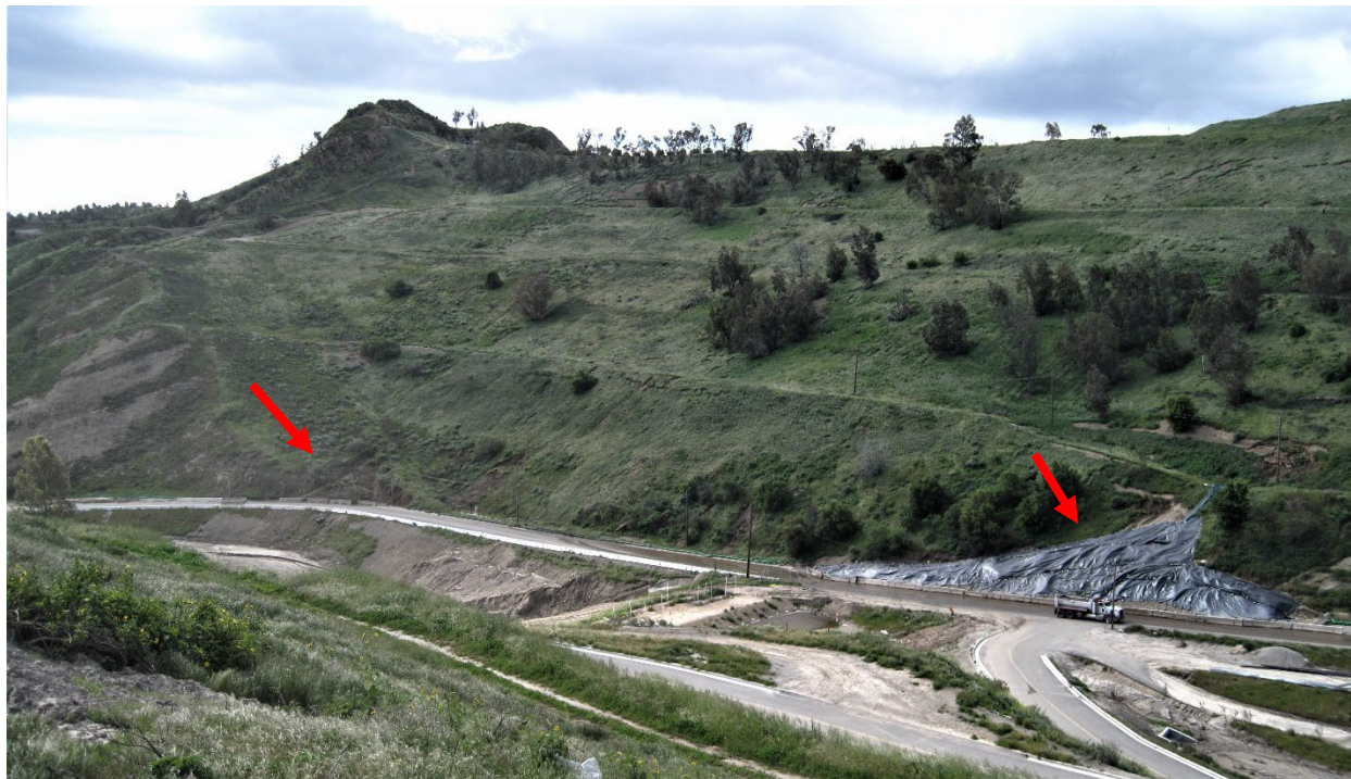
Photo 12. A view of the perimeter stormwater drainage channel surrounding the Landfill. The concrete lined channels were generally in good condition.
