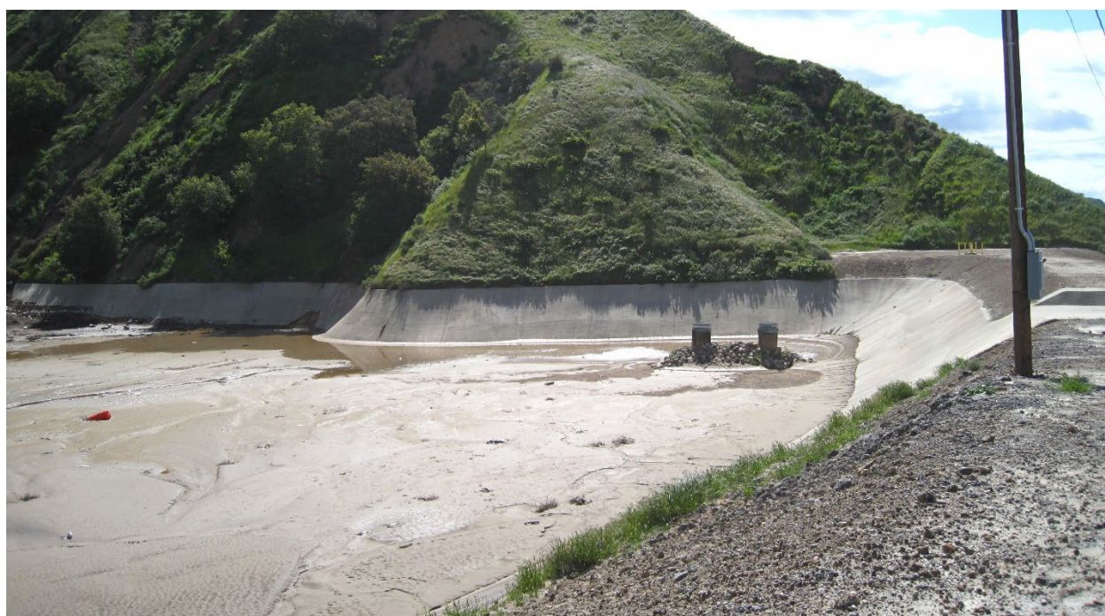
Photo 6. Sediment Basin B at the eastern edge of the Landfill, looking east. This basin receives water from Basin D to the north and discharges to the landfill's perimeter channel that ends at the Terminal Basin to the south.
