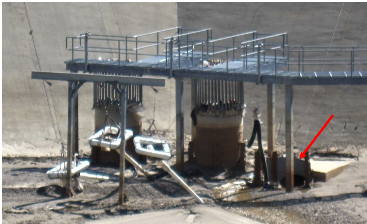
Photo 2. A close-up of the three risers of the Terminal Basin that discharge stormwater offsite. The riser on the right (arrow) was damaged (cut from the top end) during a storm in January 2023.
