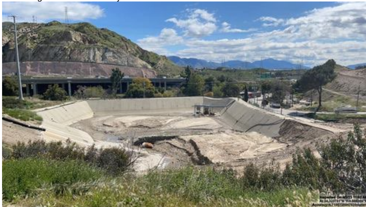
Photo 1. The Terminal Basin at the entrance of the Landfill, looking southeast. This sediment basin is at the mouth of the Sunshine Canyon and receives all stormwater runoff generated in the canyon.
