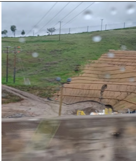
Photograph 6 (Taken February 20, 2024) Rills and erosion on active landfill slope.
