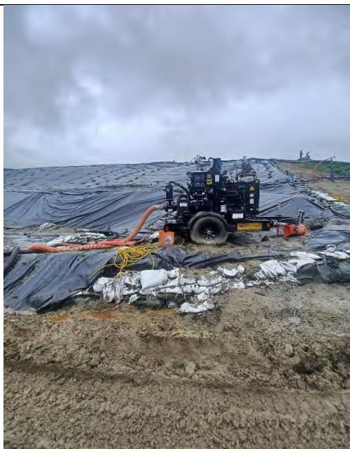
Photograph 8 (Taken February 20, 2024) The leachate seepage/leaking area and collection point located at the landfill perimeter upgradient of the stormwater basin and across from the concrete drainage channel/v-ditch; an emergency pumping equipment observed continuously pumping.
