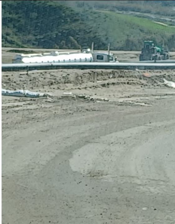
Photograph 5 (Taken January 29, 2024) Broken sandbags in a check dam.
