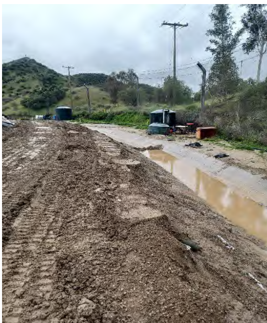
Photograph 7 (Taken February 20, 2024) Dirt check dam present in concrete-lined drainage channel/v-ditch adjacent to leachate seepage area with muddy stormwater flow.
