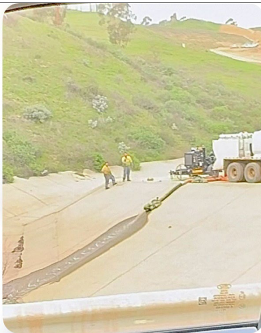
Photograph 4 (March 16, 2024 Complaint, COMP-60321) Photograph showing active pumping and discharge from either the south detention basin or the vacuum truck.
