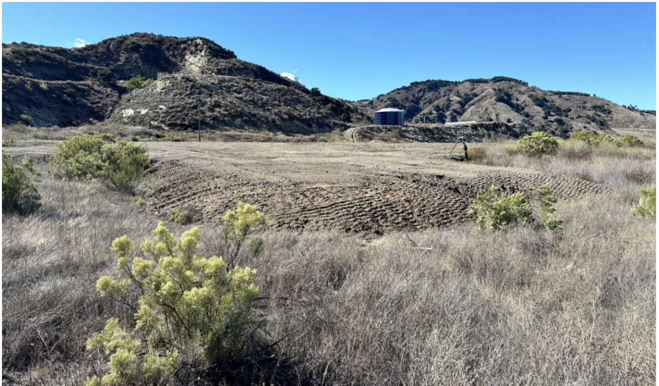
New grading on Deck A to fill in areas where settlement occurred
