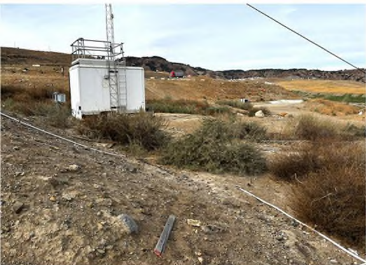
Photo Station #9 - December 2024 (West)
