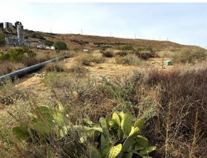
Photo Station #6 - December 2024 (West)
