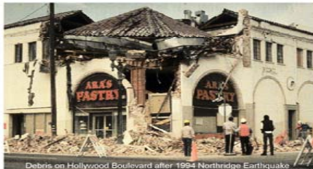
Debris on Hollywood Boulevard after 1994 Northridge Earthquake
