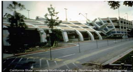
California State University Northridge Parking Structure after 1994 Earthquake
