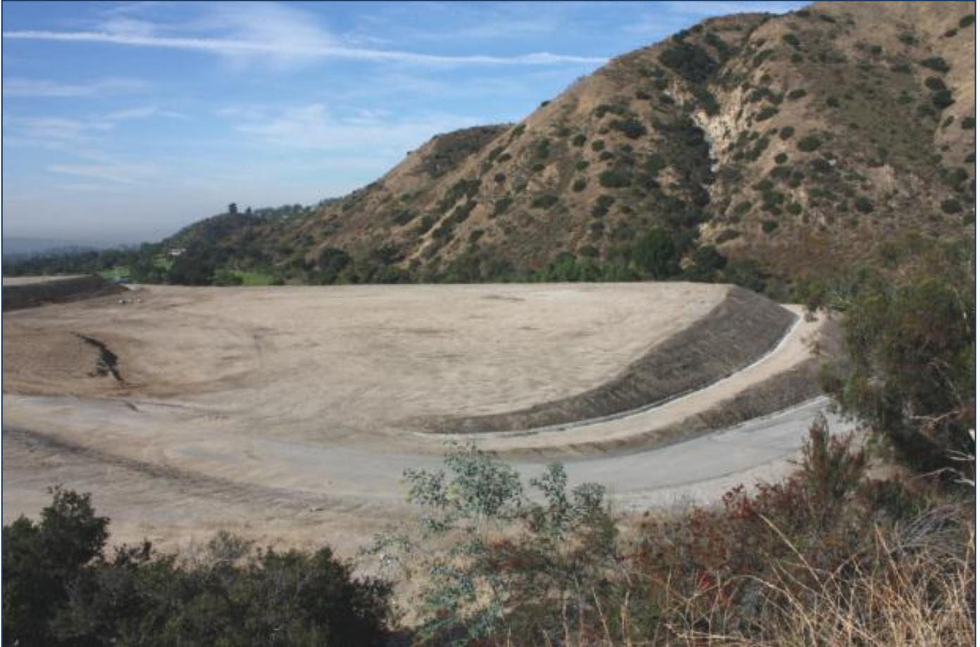
Figure 8-63 San Dimas SPS Looking Southwest
