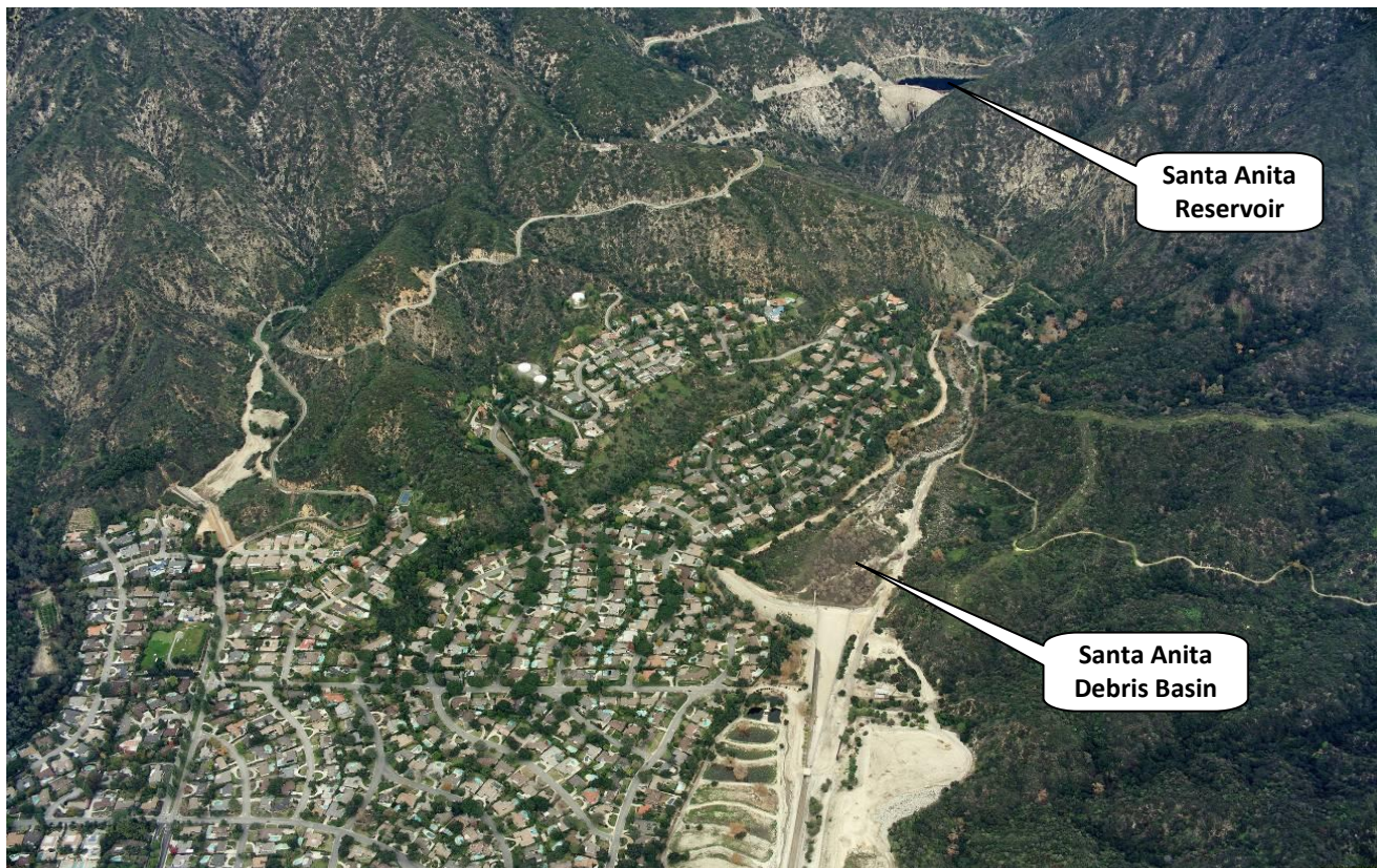
Figure 8-79 Santa Anita Debris Basin
