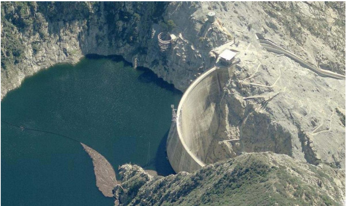
Figure 8-29 Photo of Pacoima Dam
