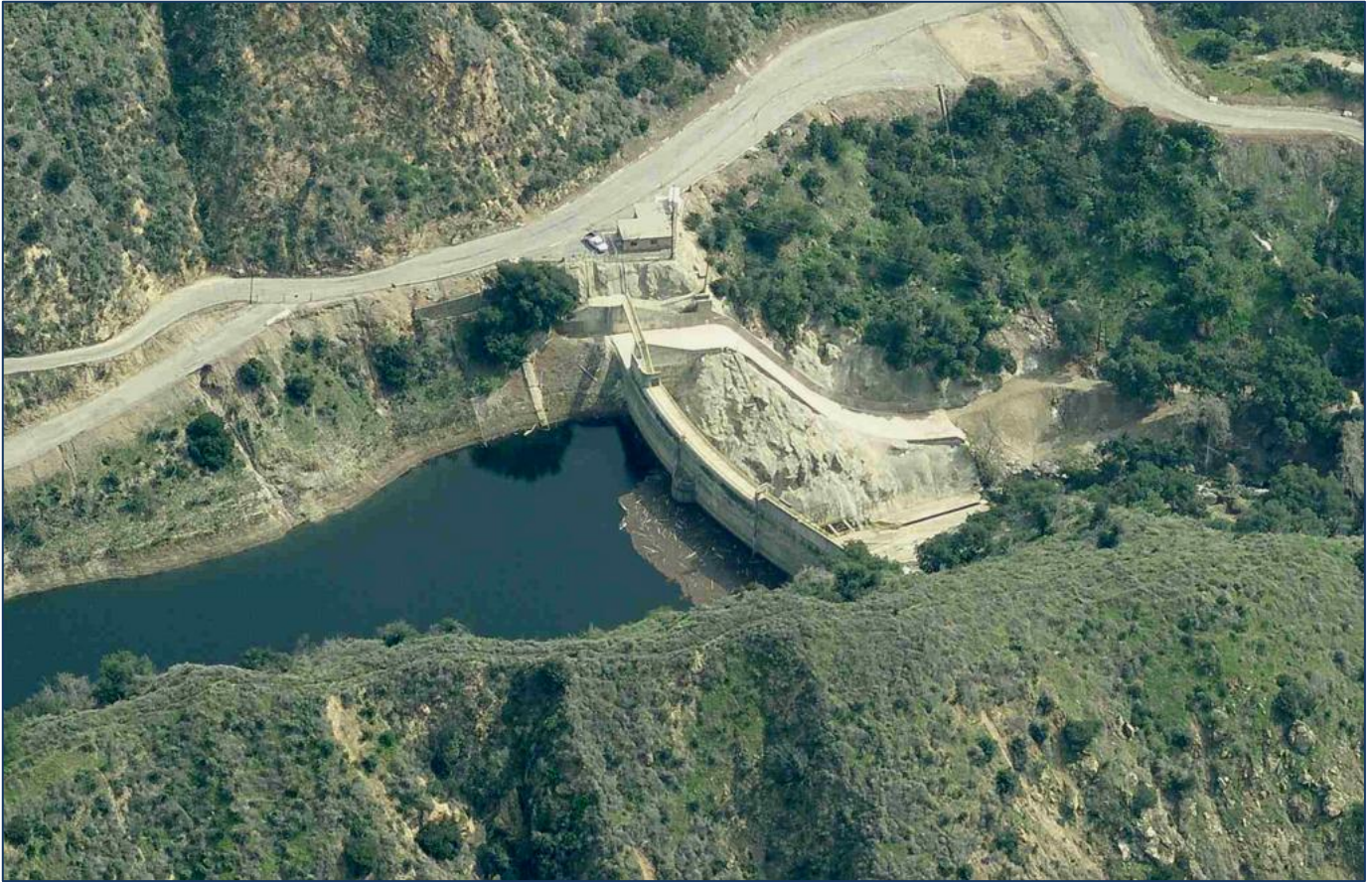
Figure 8-58 Photo of San Dimas Dam
