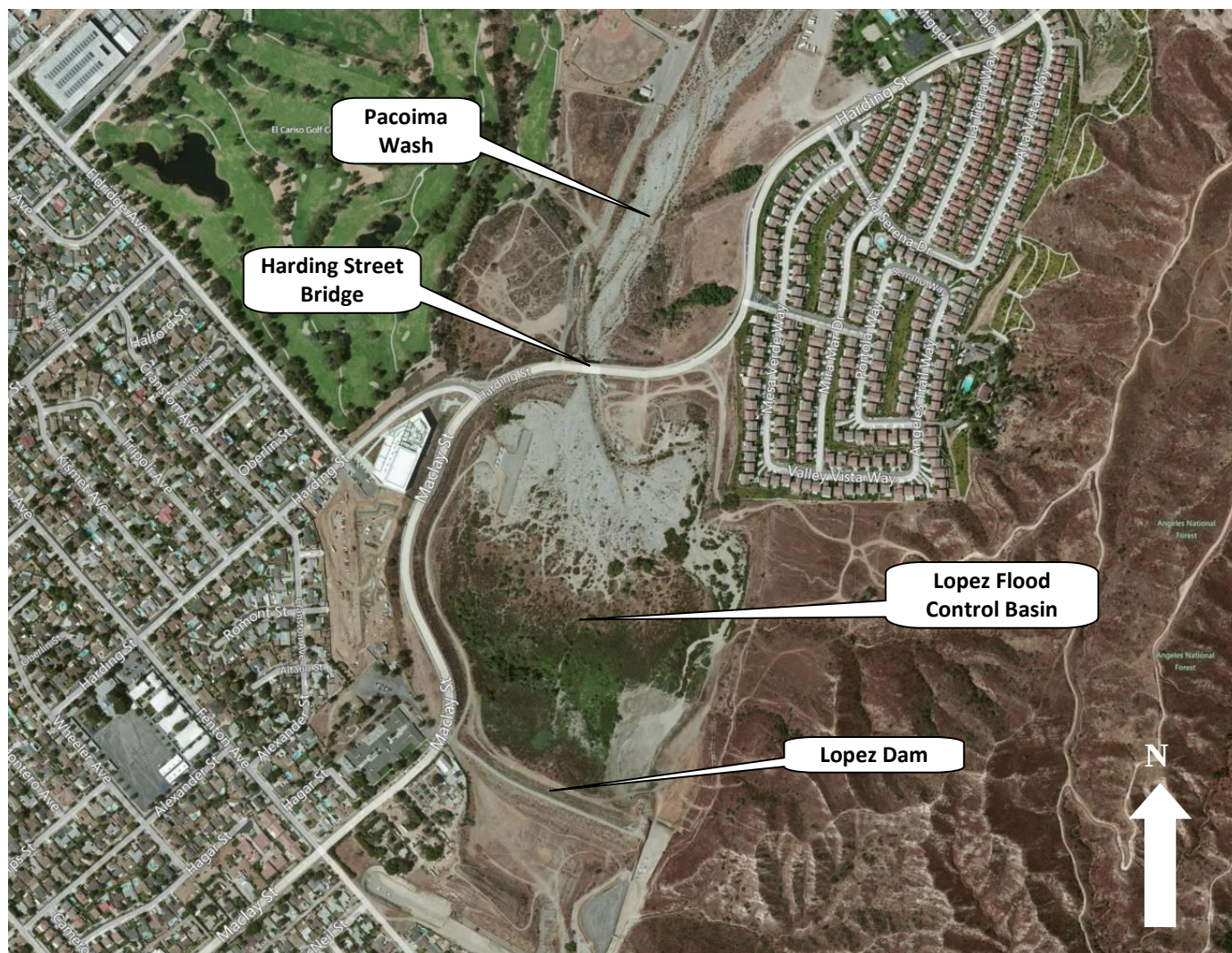
Figure 8-34 Lopez Flood Control Basin
